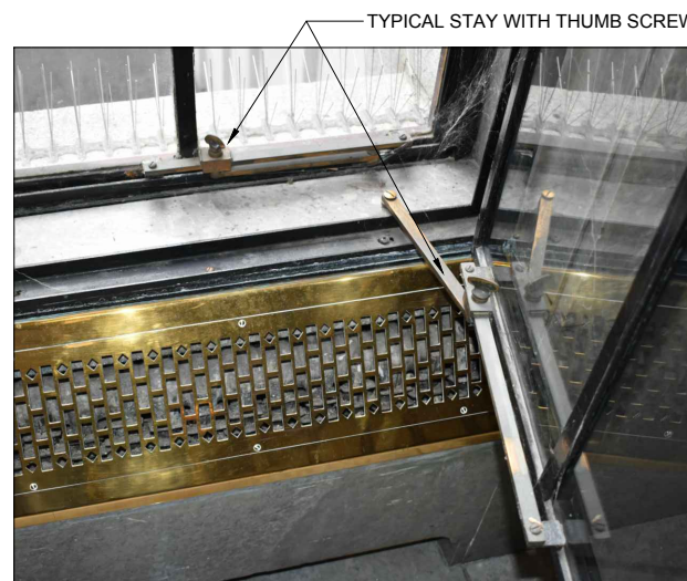
TYPICAL STAY WITH THUMB SCREW LOCATION
