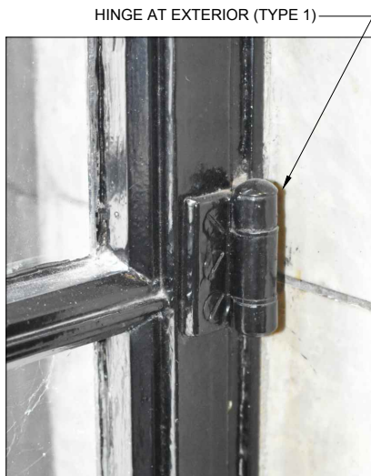
5 A15 NTS TYPICAL HINGES SHOWING FASTENERS
