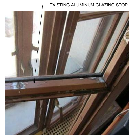
EXISTING STOP WITH FASTENERS
