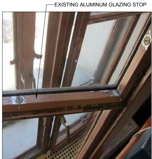
7 A15 NTS EXISTING STOP WITH FASTENERS
