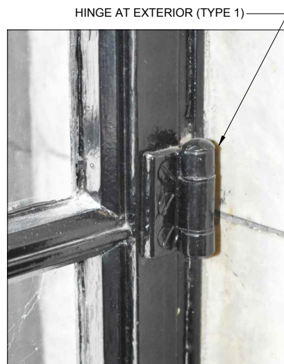
TYPICAL HINGES SHOWING FASTENERS
