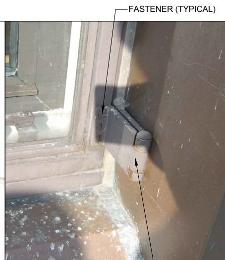
HINGE AT EXTERIOR (TYPE 2)
