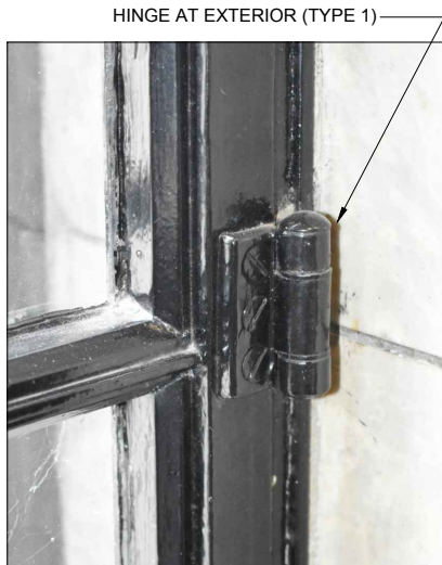
5 A15 NTS TYPICAL HINGES SHOWING FASTENERS
