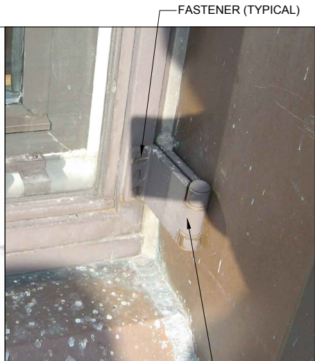
HINGE AT EXTERIOR (TYPE 2)
