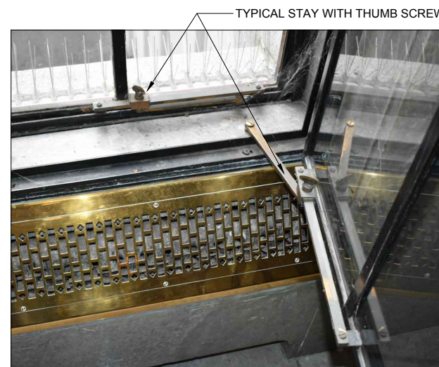
TYPICAL STAY WITH THUMB SCREW LOCATION
