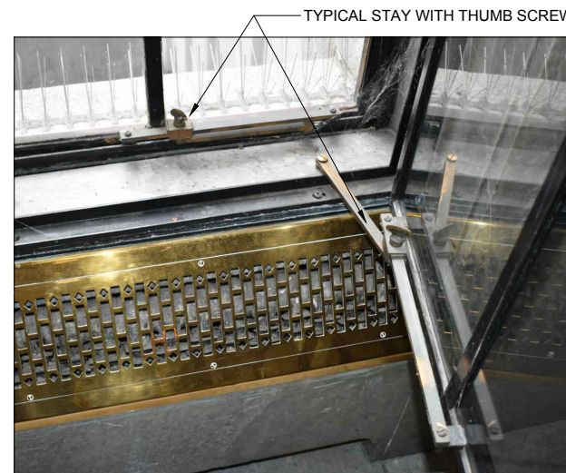
6 A15 NTS TYPICAL STAY WITH THUMB SCREW LOCATION
