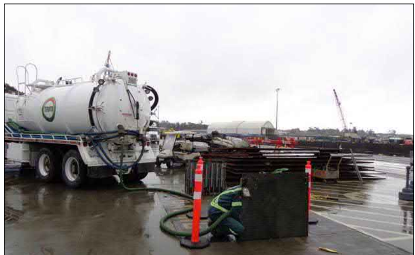
Lift Station Maintenance.
