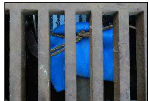
Filter cloth secured over sump well valve to allow stormwater flow.
