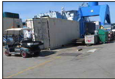
AUTHORIZED Sanitary Sewer Discharge point, Lift Station #15.
