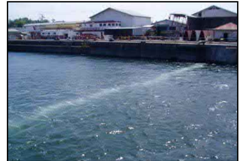
Bubble curtain employed during vessel transfer.
