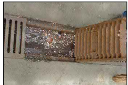
Do not allow trench drains to build up with debris. This helps to prevent flooding during heavy stormwater events.
