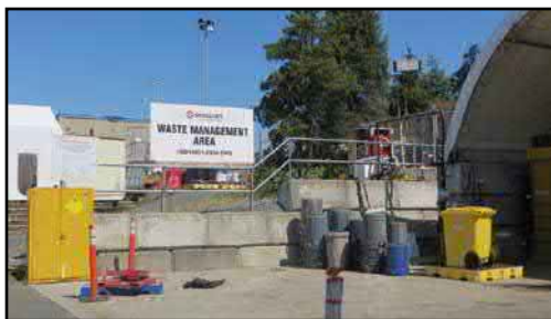
An example of a Waste Management Area at the EGD.
