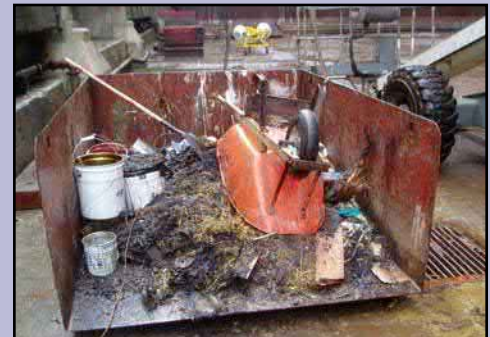
INADEQUATE waste grit storage.
