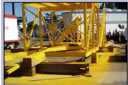
INADEQUATE containment.
