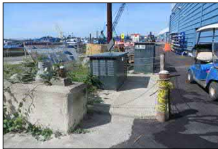
AUTHORIZED Sanitary Sewer Discharge point, Lift Station #11.
