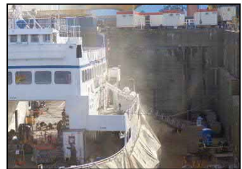
INADEQUATE containment.
