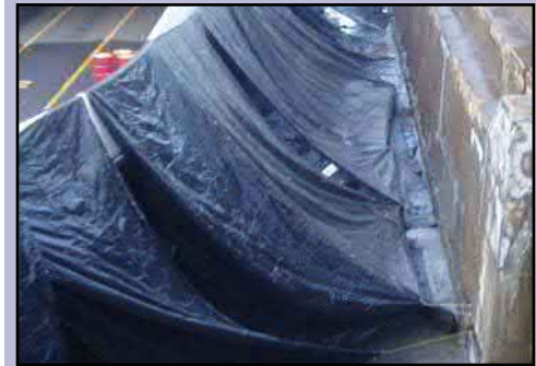
INADEQUATE containment.
