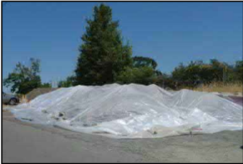
ADEQUATE soil stockpile management. Soils placed on poly and covered.
