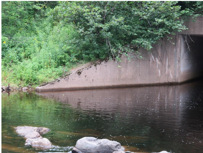
Figure 6: Wingwall located at Bennett Brook Culvert Outlet (South Side)
