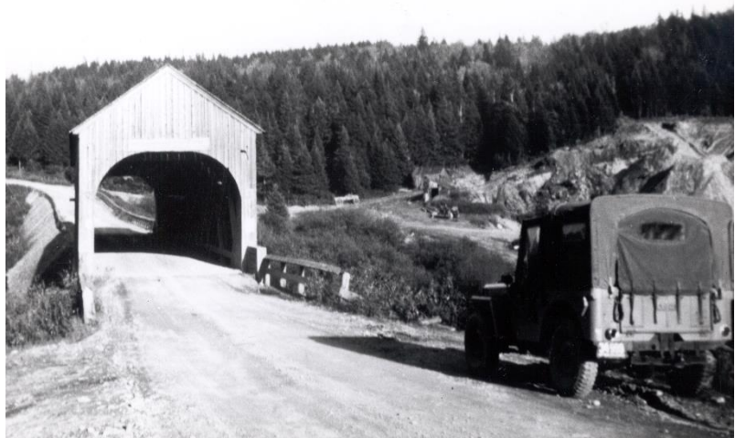
Figure 12: Bennett Lake Covered Bridge & Area South of the Highway (1950)
