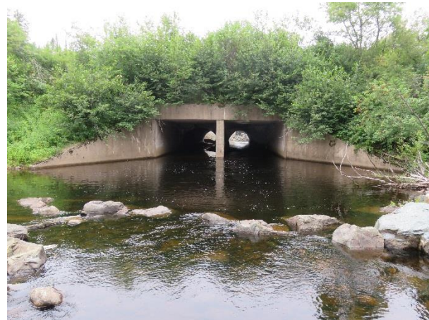
Figure 4: Culvert Outlet View
