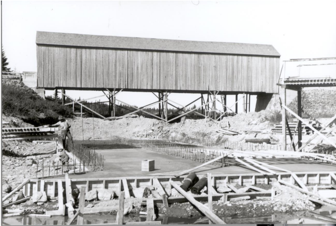
Figure 2: Construction of Original Culvert Prior to 1955
