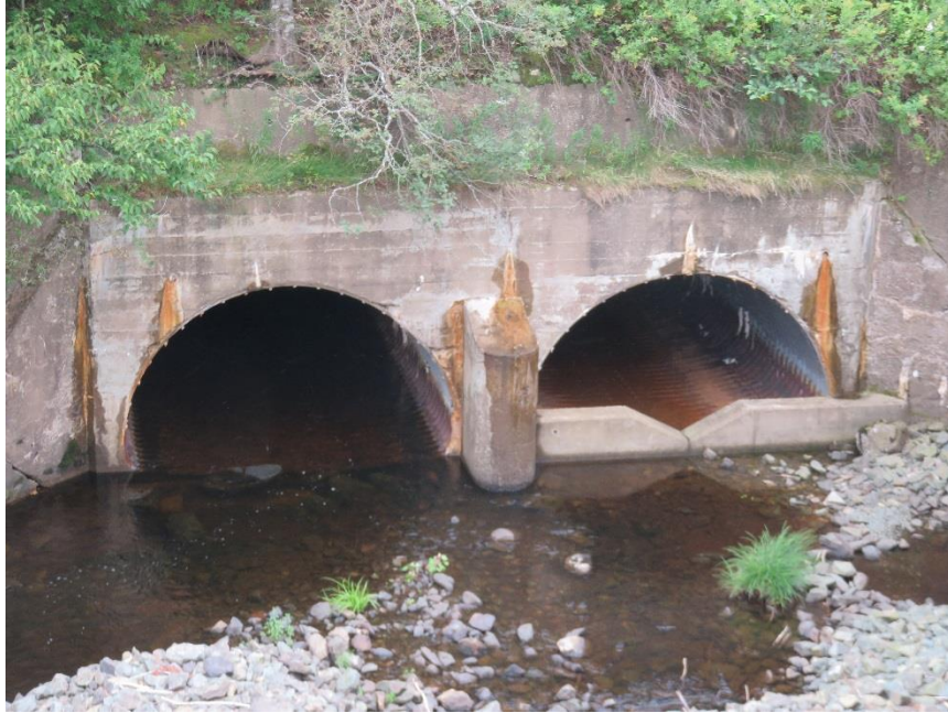
Figure 7: Bennett Brook Culvert Inlet Headwall (North End)
