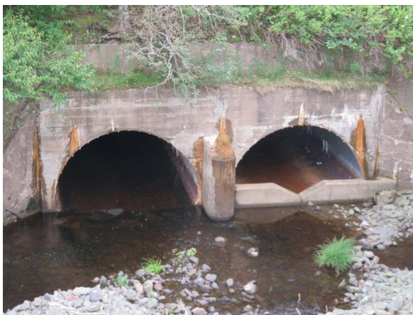
Figure 3: Culvert Inlet View
