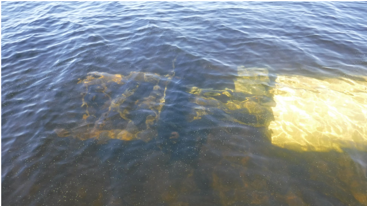
Figure 8 – LL1380 Existing Navaid and Steel Structure (to be removed)
