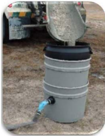
(Concrete Washout Filter (EPA 2012), Mark Shaw, Ultra Tech International, Inc.)
