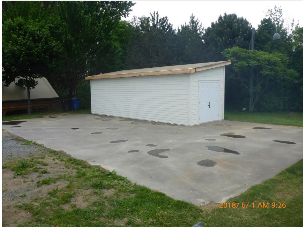
Photo 1: Location where the services are to be laid out and the existing building (electrical room and storage area)
