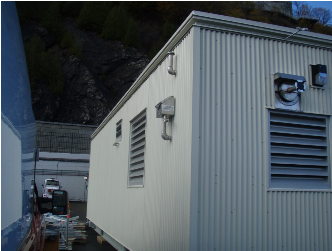
Photo 12: New shelter to be installed
