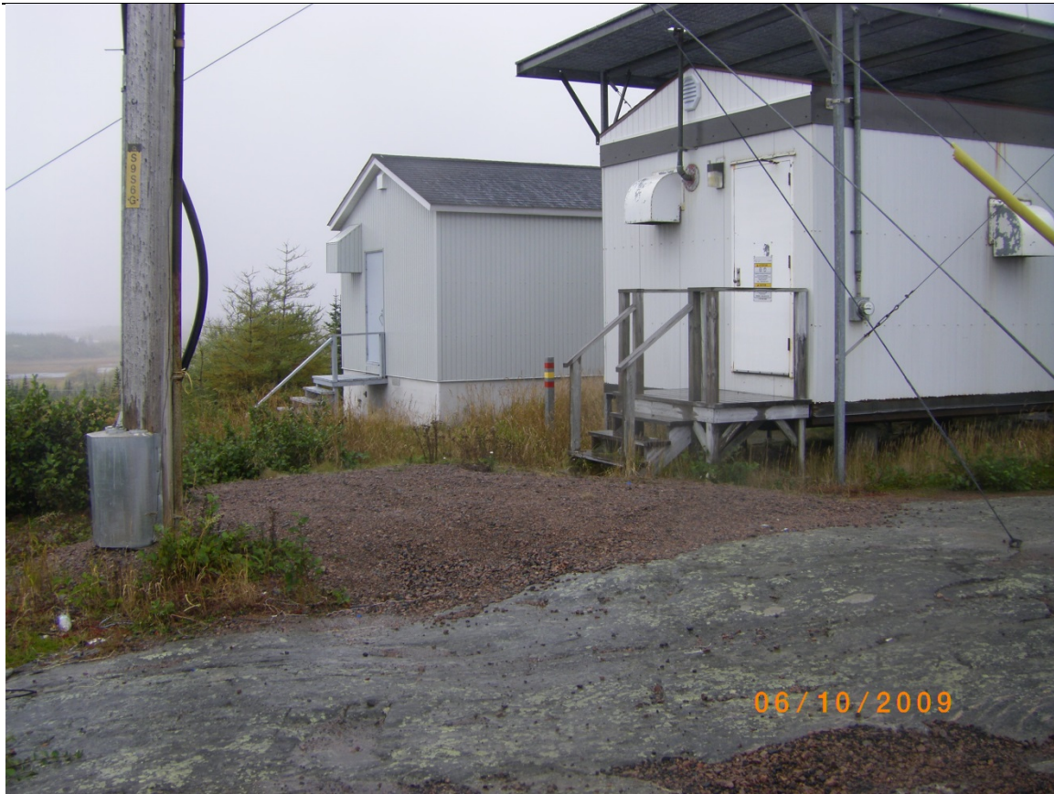
Photo 6: Electrical pole and rock found on surface.
