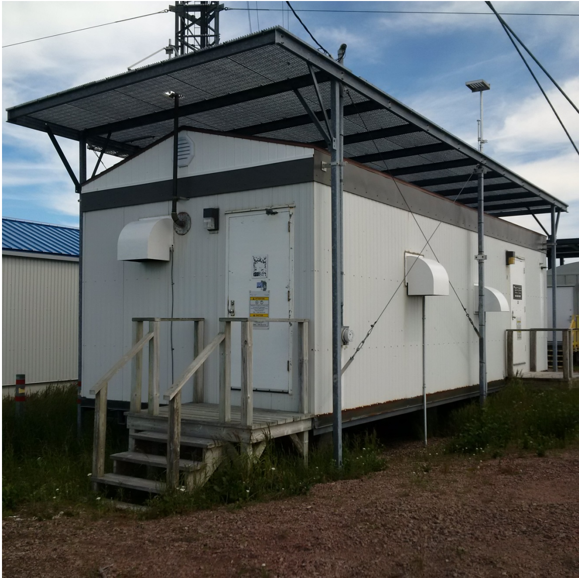
Photo 3: Existing CCG shelter
