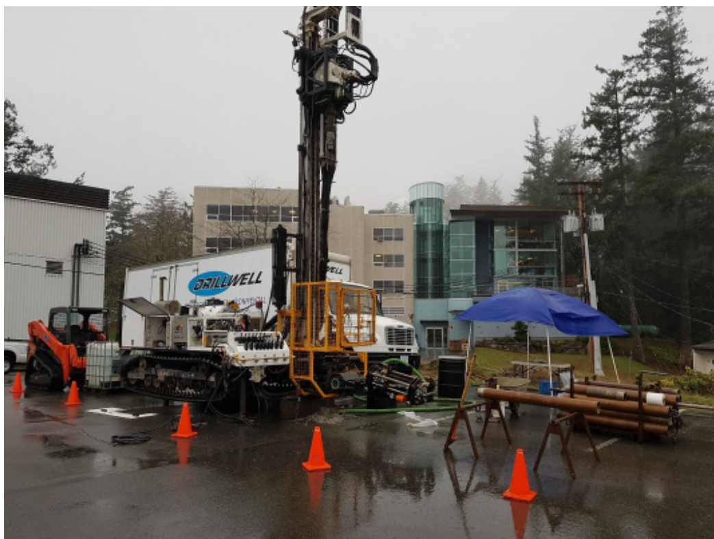
Photo 1: Track mounted sonic rig and equipment set up at SDH18-01.
