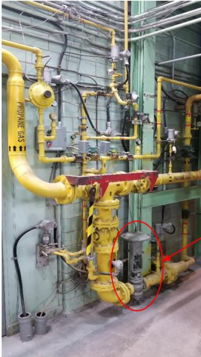
Image 3. Main gas supply to Wall and Floor combustion testing furnaces. Main distribution.
