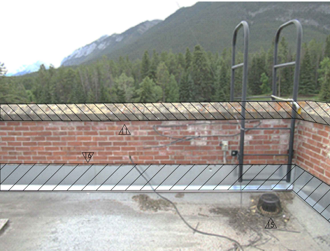
2 TOWER ROOF - LOOKING NORTH A113
