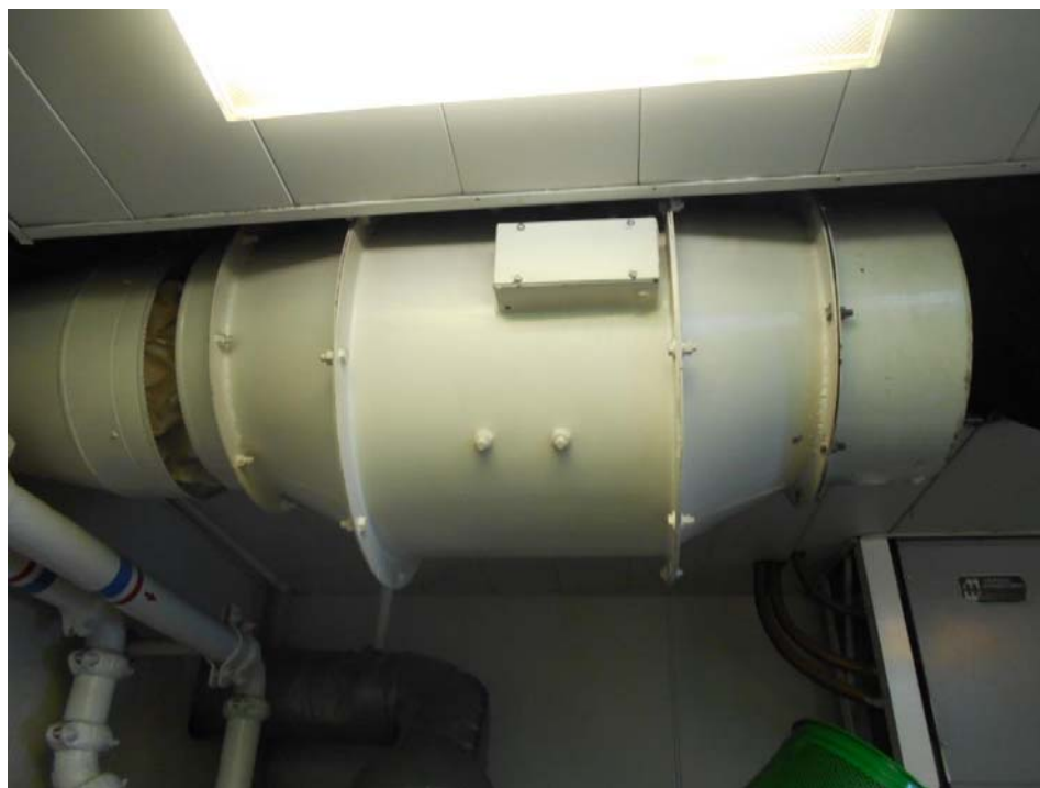
Figure 6: Photograph of in-situ emergency generator supply axial fan.
