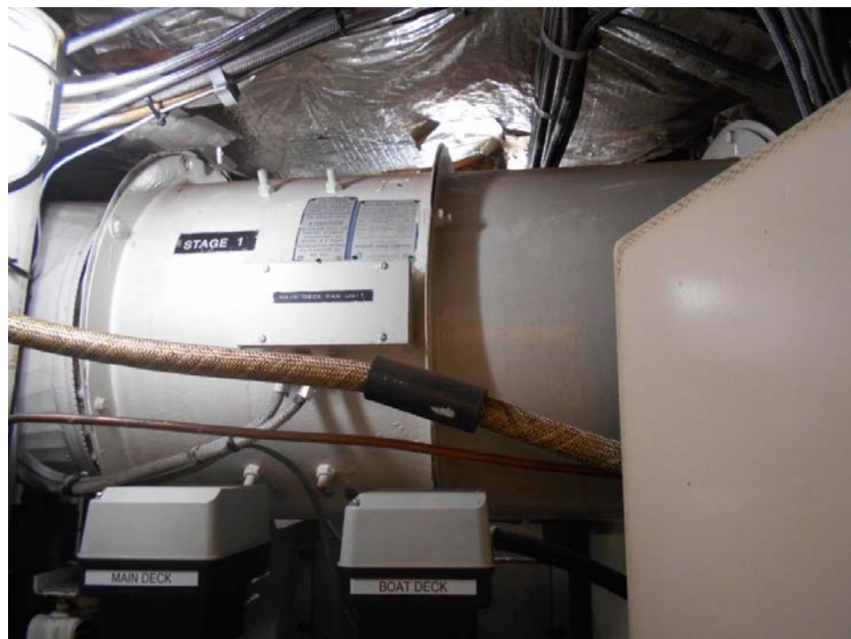
Figure 4: Photograph of in-situ main deck supply axial fan.
