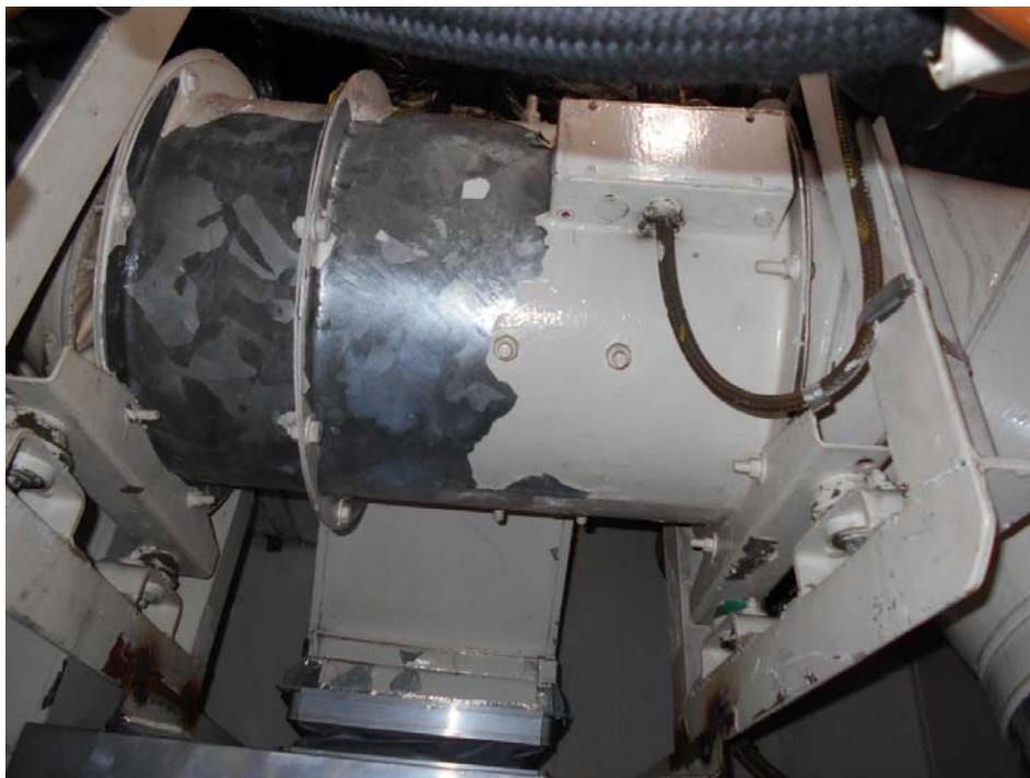
Figure 7: Photograph of in-situ focsule deck supply axial fan.
