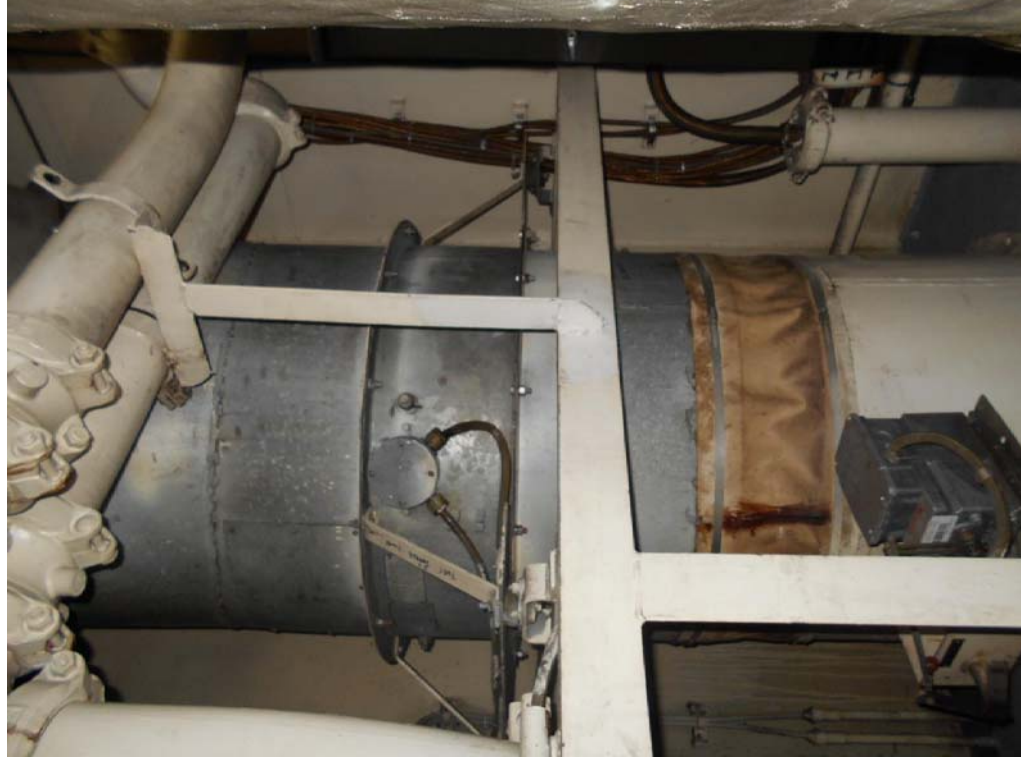
Figure 2: Photograph of in-situ engine room exhaust axial fan.
