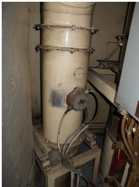
Figure 10: Photograph of in-situ MCR supply axial fan.
