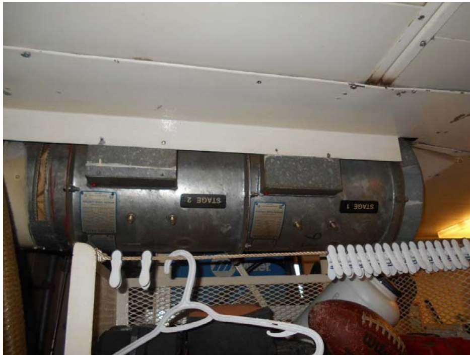
Figure 9: Photograph of in-situ deck workshop supply axial fan.
