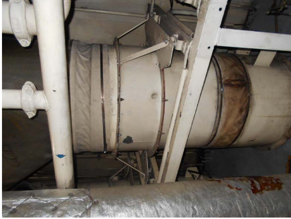
Figure 1: Photograph of in-situ engine room supply axial fan.
