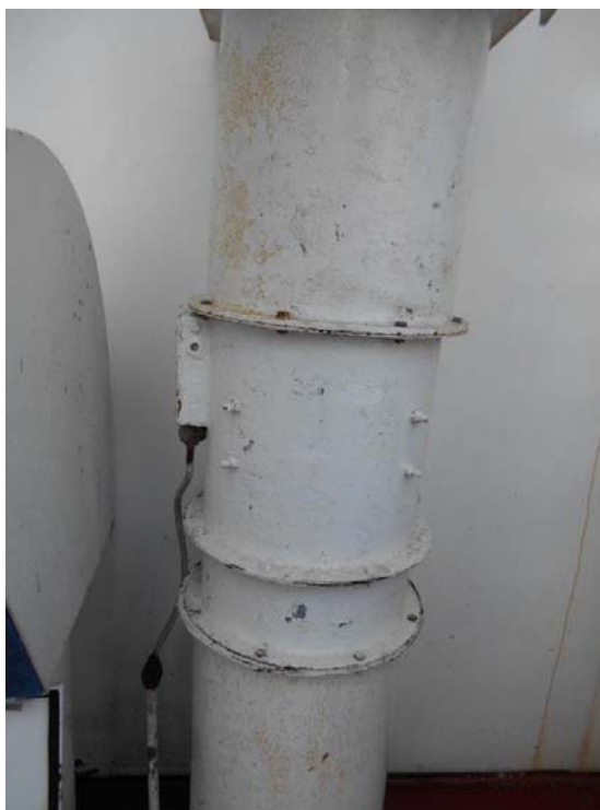
Figure 8: Photograph of in-situ galley exhaust axial fan.
