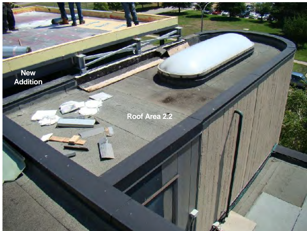
Photograph 57: Roof Area 2.2 – This small roof area is situated over the central stairwell and consists of a modified bitumen membrane system installed in the early to mid 1990's. The addition to the mechanical room is situated directly to the east of this roof area.
