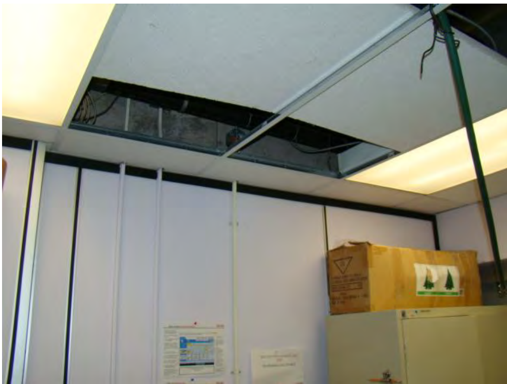
Photograph 18: Roof Area 1.2 (Interior) – Missing ceiling tile along east wall of office S208 due to ongoing roof leak at transition with the central stairwell wall.
