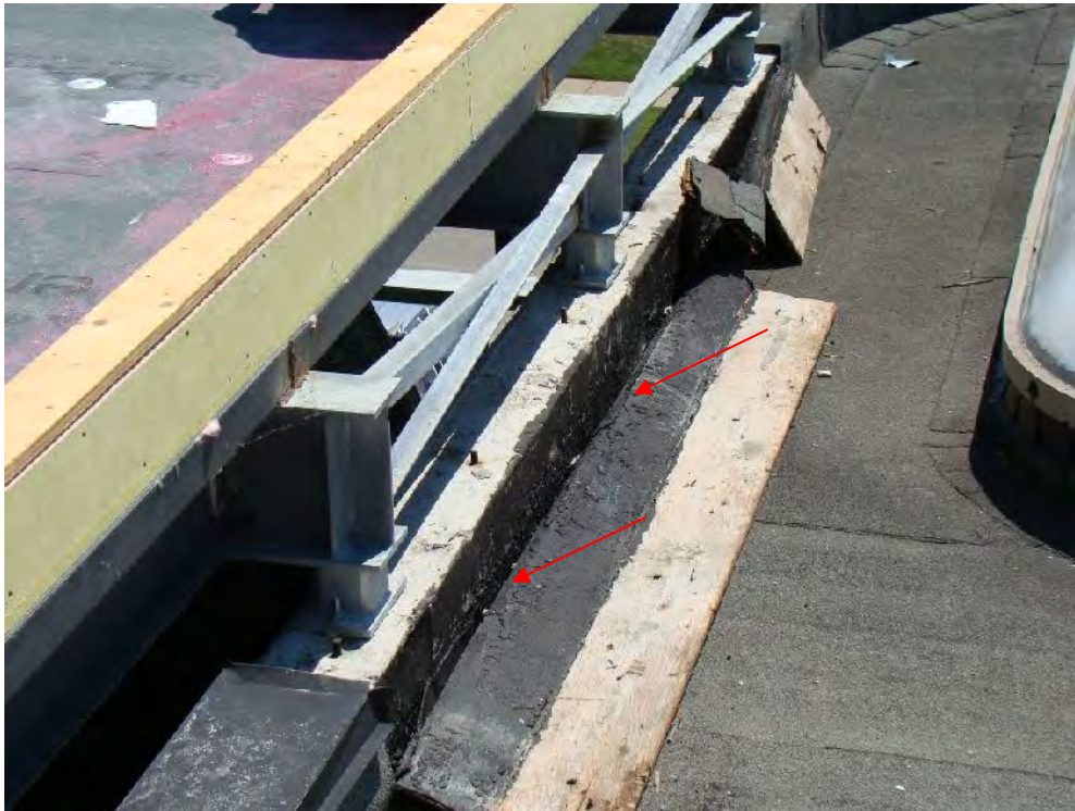
Photograph 59: Roof Area 2.2 - The east parapet flashings have been removed to facilitate construction of the new addition. It appears that minimal protection from water entry has been provided along the edge.
