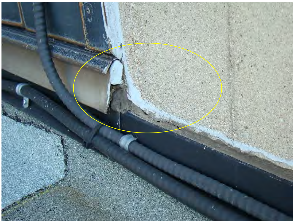
Photograph 26: Roof Area 1.2 – Openings in sealant along reglet flashing details may be contributing to leakage.
