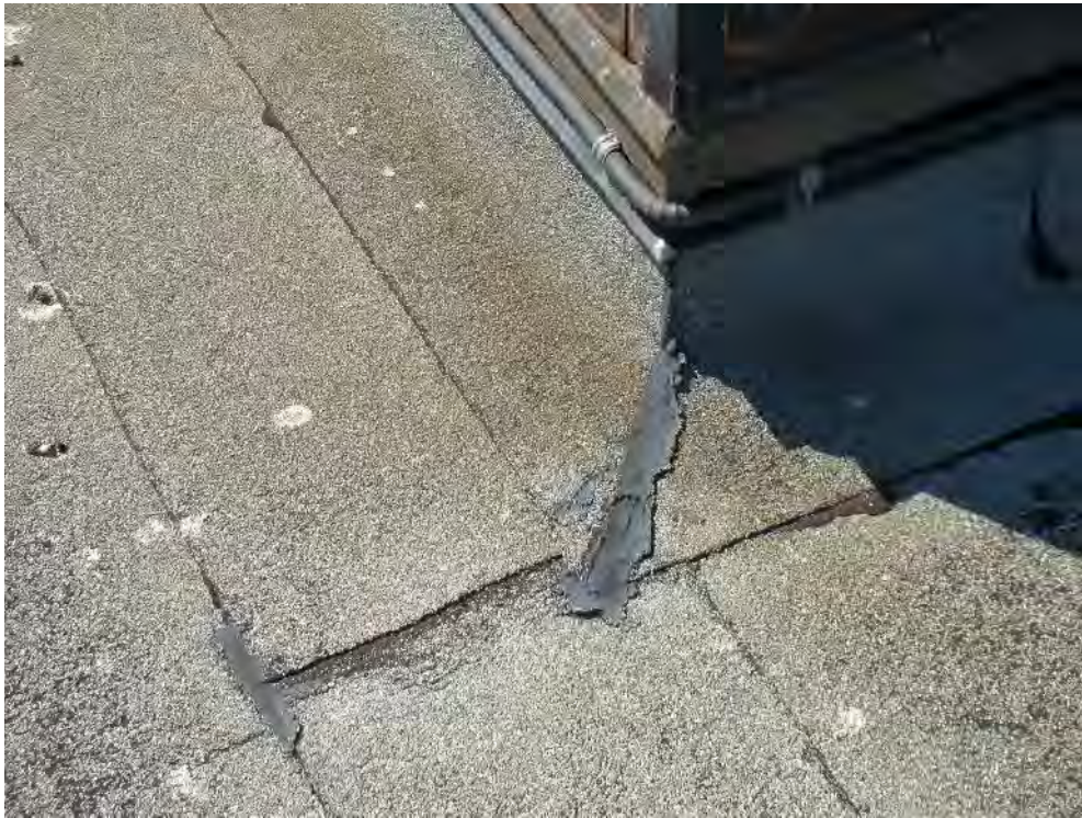
Photograph 41: Roof Area 1.2 – Failed sealant repairs were observed at several corner transitions.
