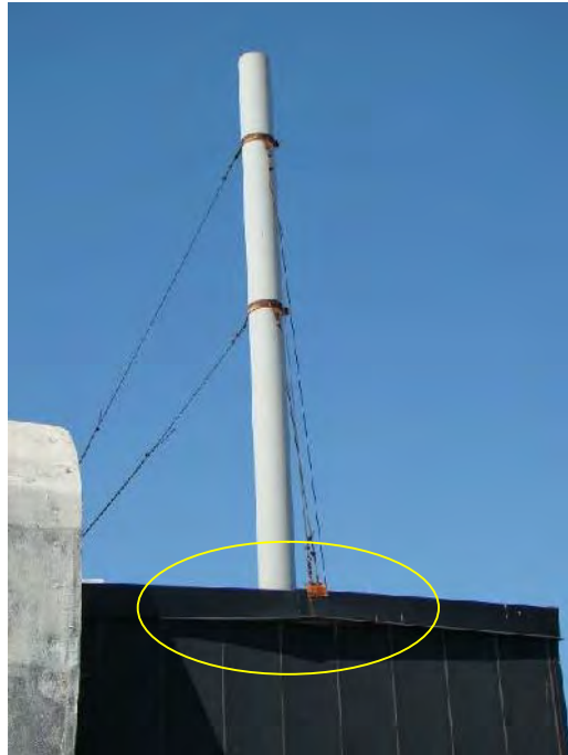
Photograph 81: Roof Area 3.1 – The guy wire chimney support along the east parapet has dislodged the existing metal flashings at its securement point. This has resulted in less than optimal support for the stack.
