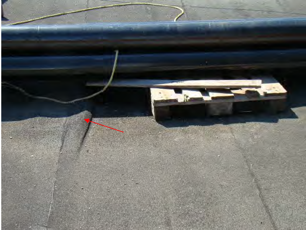
Photograph 39: Roof Area 1.2 – Membrane blister has been crushed under the weight of construction materials stockpiled on the roof. This condition will likely cause membrane damage and water entry.
