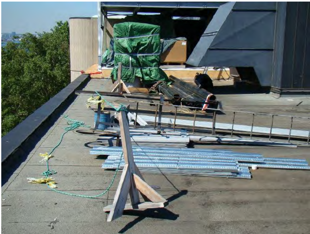
Photograph 44: Roof Area 1.2 – Heavy construction materials have been stockpiled on the membrane in the southeast corner of the roof area.
