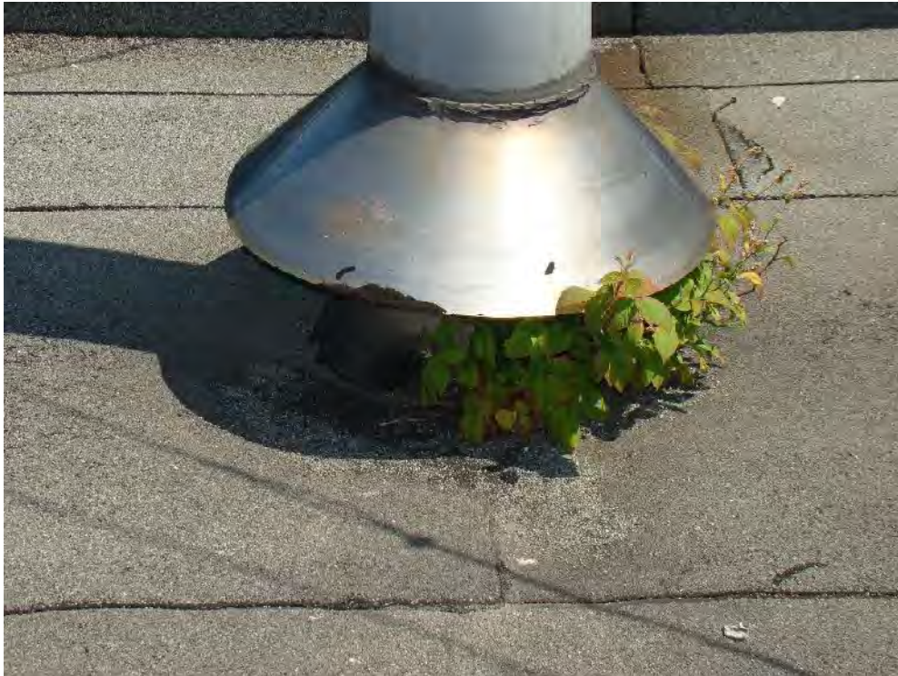
Photograph 73: Roof Area 3.1 – Vegetation was observed around the b-vent flashings at the northeast corner of the roof further confirming that the insulation below the membrane is filled with moisture and is supporting vegetation growth.
