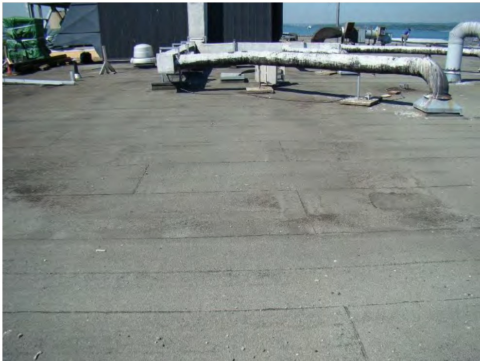
Photograph 14: Roof Area 1.2 – View looking west along the central portion of the roof area. Evidence of heavy ponding is noted by the dark colouration of the membrane.
