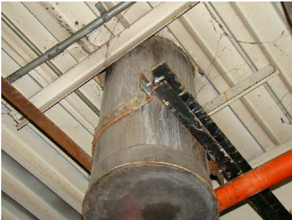
Photograph 74: Roof Area 3.1 – Water entry was visible from below around the b-vent chimneys. This is likely due to the saturated condition of the insulation causing water to infiltrate anywhere there are openings in the steel decking.
