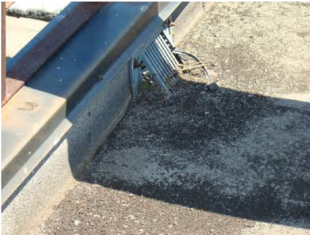
Photograph 76: Roof Area 3.1 – The primary drainage for this roof area is provided by two – six inch scuppers along the north perimeter. Both scuppers are heavily obstructed by debris.
