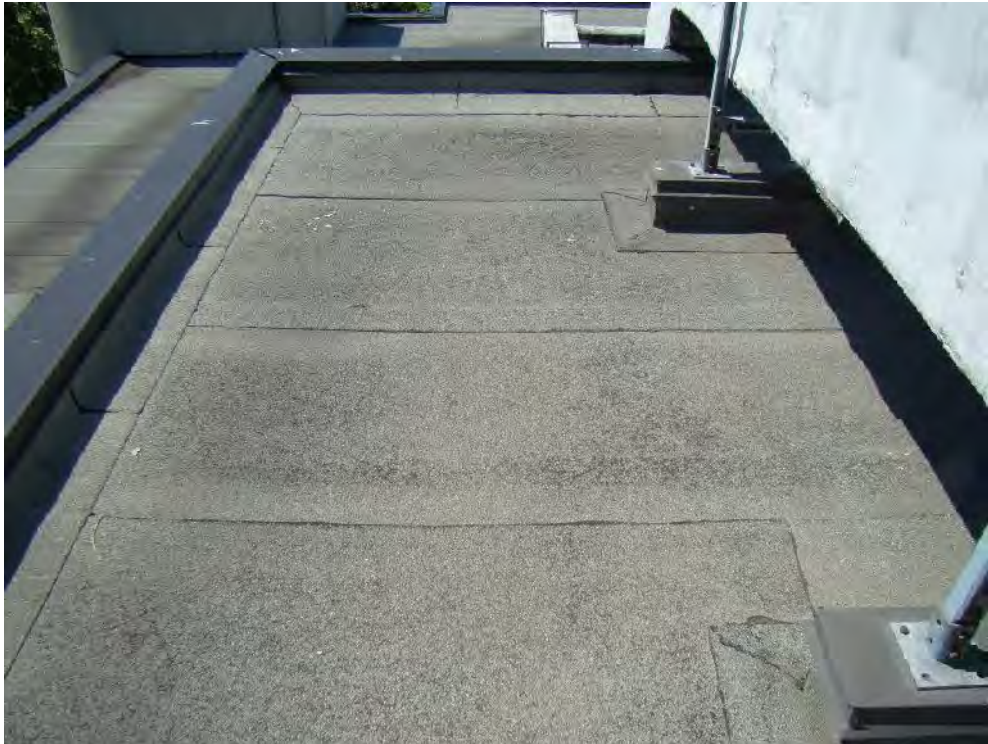
Photograph 77: Roof Area 3.1 – The cap sheet membrane appears weathered and worn with general granule surface loss throughout the roof area.
