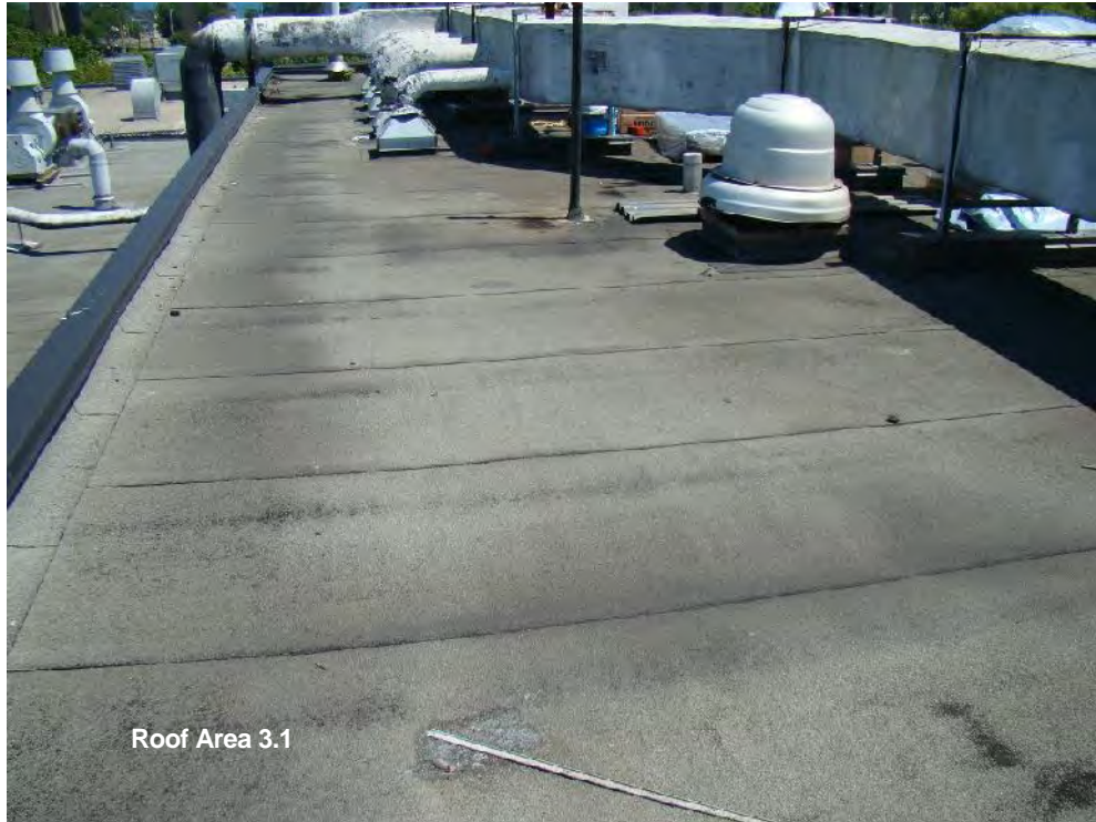
Photograph 67: Roof Area 3.1 – This roof is situated over the upper mechanical room and consists of a modified bitumen membrane system installed in the early to mid 1990's.
