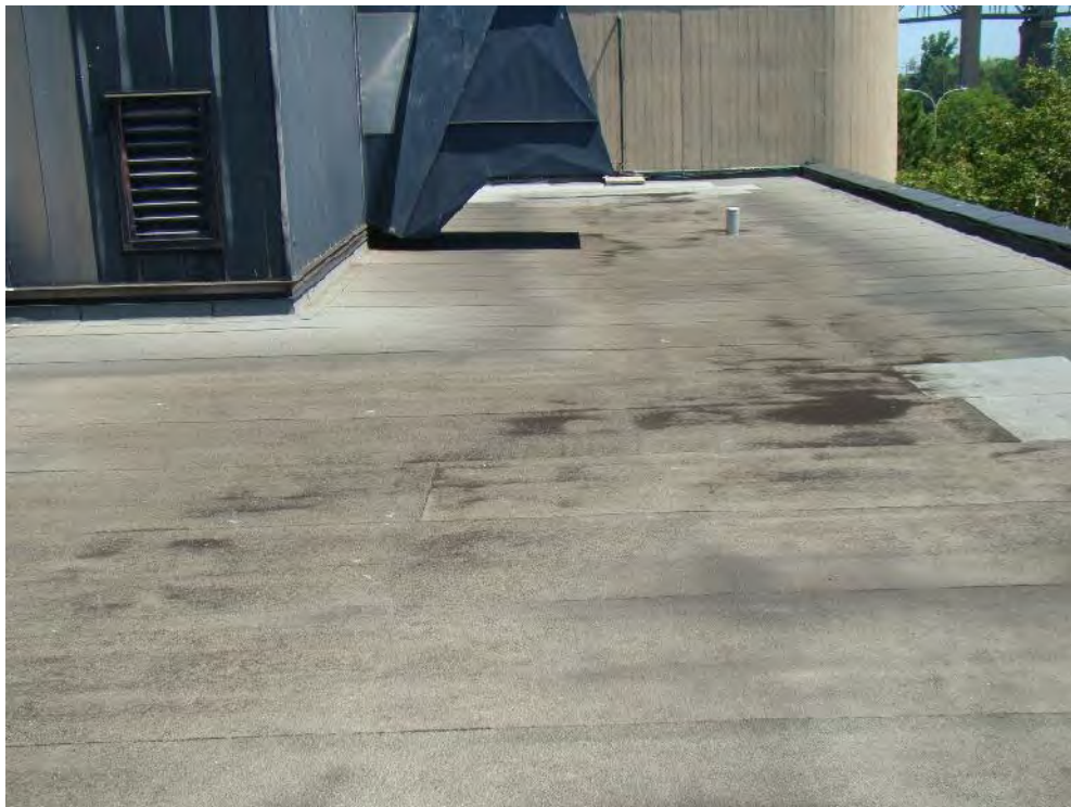
Photograph 16: Roof Area 1.2 – View looking east along the south portion of the roof showing evidence of ponding. Tapered insulation is directing water into the central portion of the roof.
