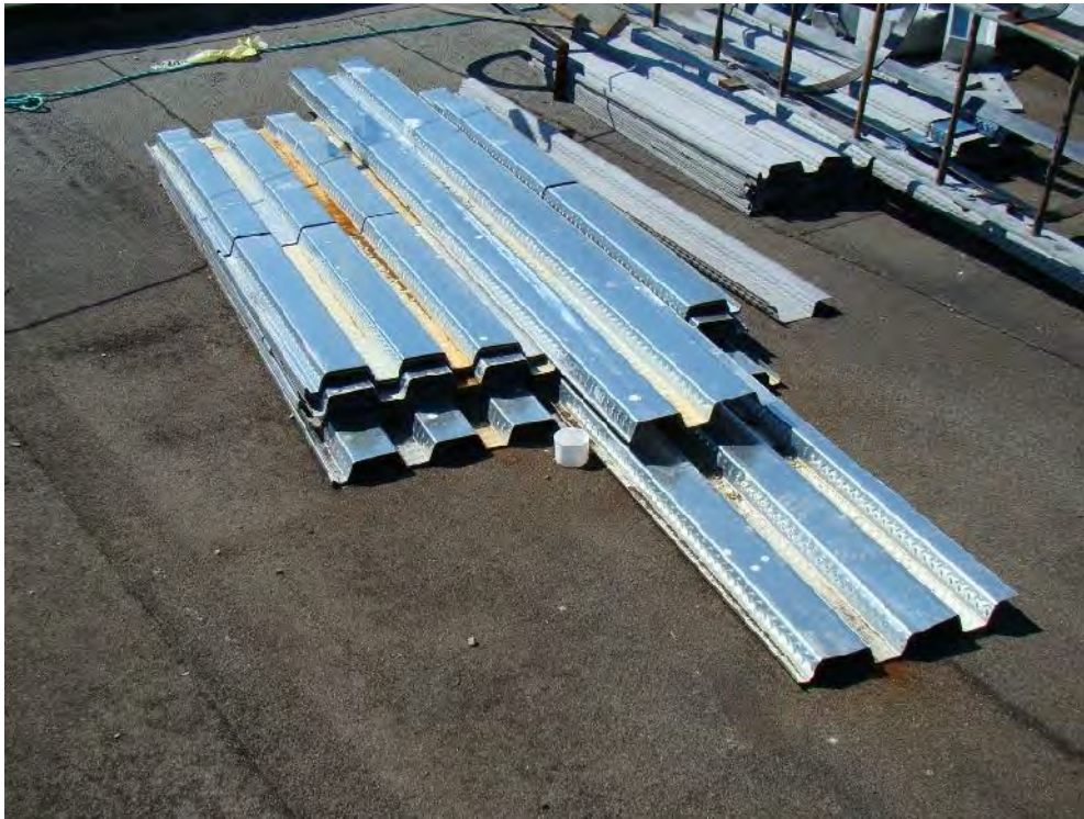
Photograph 45: Roof Area 1.2 – Inadequate protection has been provided under the materials which will result in damage to the membrane.
