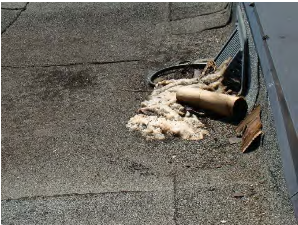
Photograph 60: Roof Area 2.2 – Debris is obstructing the drainage scupper.
