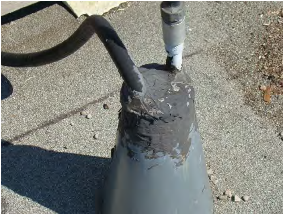
Photograph 47: Roof Area 1.2 – Electrical cone flashings adjacent to HVAC units are poorly sealed and open to moisture entry.
