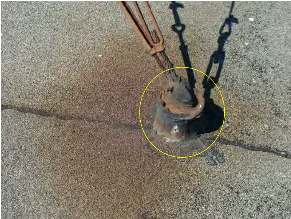
Photograph 48: Roof Area 1.2– Deterioration of the filler material was evident at guy wire pitch pocket penetrations.
