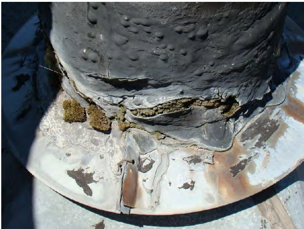
Photograph 80: Roof Area 3.1 – Severe deterioration of the ductwork waterproofing is resulting water infiltration and saturation of the underlying insulation (moss growth under waterproofing visible).
