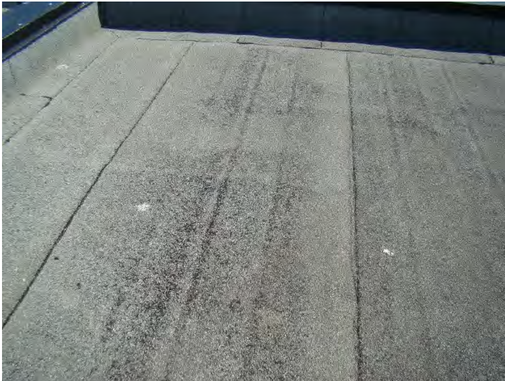
Photograph 63: Roof Area 2.3 – The cap sheet membrane appears weathered and worn with general granule surface loss throughout
