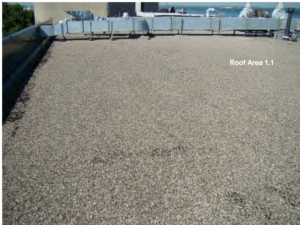
Photograph 4: Roof Area 1.1 - Overall view looking west. The existing roof system on this area was assessed to be in serviceable condition requiring preventative maintenance in order to extend service life.
