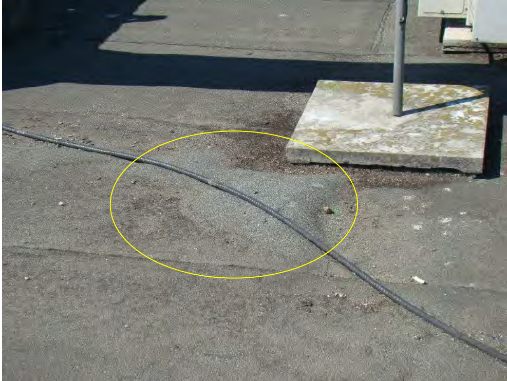
Photograph 37: Roof Area 1.2 – Widespread membrane blistering exists within the field of the roof and is indicative of poor adhesion of the membrane to the insulation substrate or delamination between the base and cap sheet membranes.
