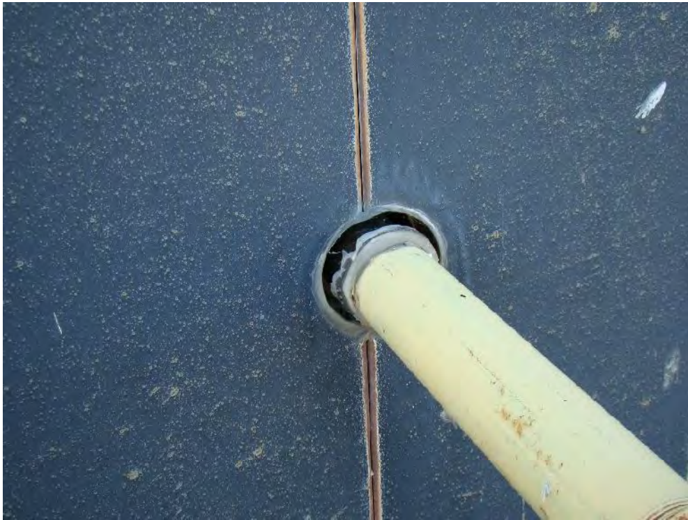
Photograph 51: Roof Area 1.2 - Sealant at the gasoline penetration through the north penthouse wall has failed resulting in water infiltration.
