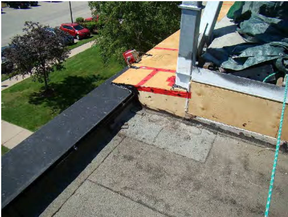
Photograph 20: Roof Area 1.2 – View of the transition of the new addition with the existing roof. Due to the unfinished construction, there may be multiple avenues for water to infiltrate the interior space below.
