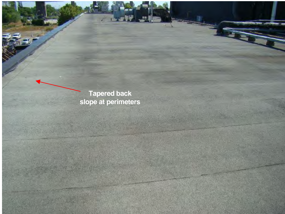
Photograph 15: Roof Area 1.2 – View looking east along the north portion of the roof area. Tapered insulation back slope has been installed to provide positive drainage away from the perimeters. The back slope extends approximately 4 to 6 feet out from the wall.
