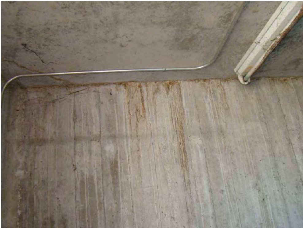
Photograph 66: Roof Area 2.3 – Evidence of moisture staining along the east wall indicates previous leakage.
