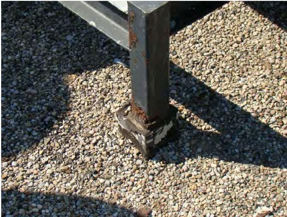
Photograph 11: Roof Area 1.1– Deterioration of the filler material was evident at pitch pocket penetrations along mechanical ductwork supports.
