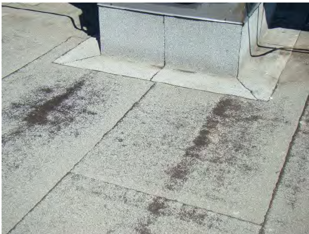
Photograph 34: Roof Area 1.2 – Granule loss is typical around mechanical curbs due to regular foot traffic patterns.
