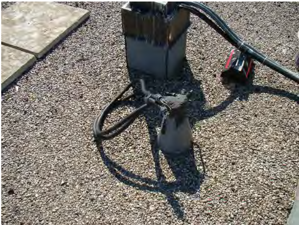
Photograph 12: Roof Area 1.1 – Unused cone penetrations are evident in various locations and should be removed at the time of the next roof replacement.
