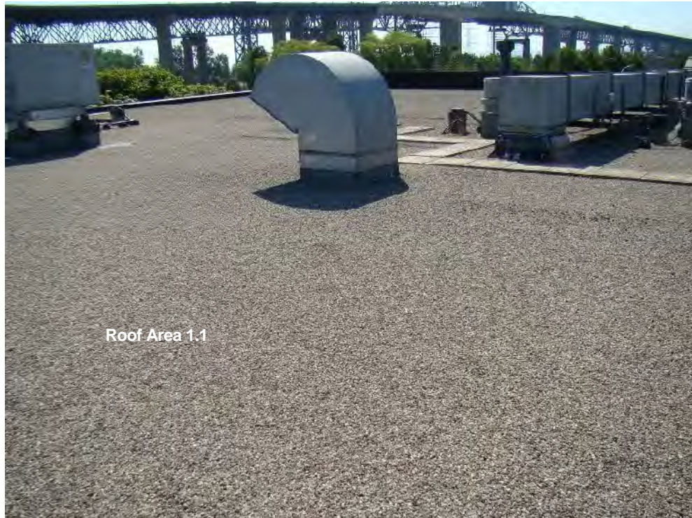
Photograph 3: Roof Area 1.1 – Overall view looking south. This roof area is situated over the east addition to the building and consists of a conventional 4 ply built up bituminous membrane system installed in 1996.
