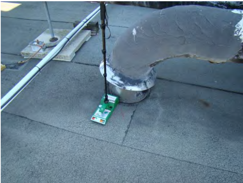
Photograph 24: Roof Area 1.2 – Moisture detected adjacent to tall cone chimney penetrations due to membrane flashing delamination and sealant failure.
