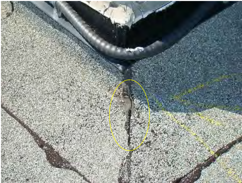
Photograph 28: Roof Area 1.2 – Open membrane flashings were observed to be causing moisture entry at the corner of the stairwell wall.
