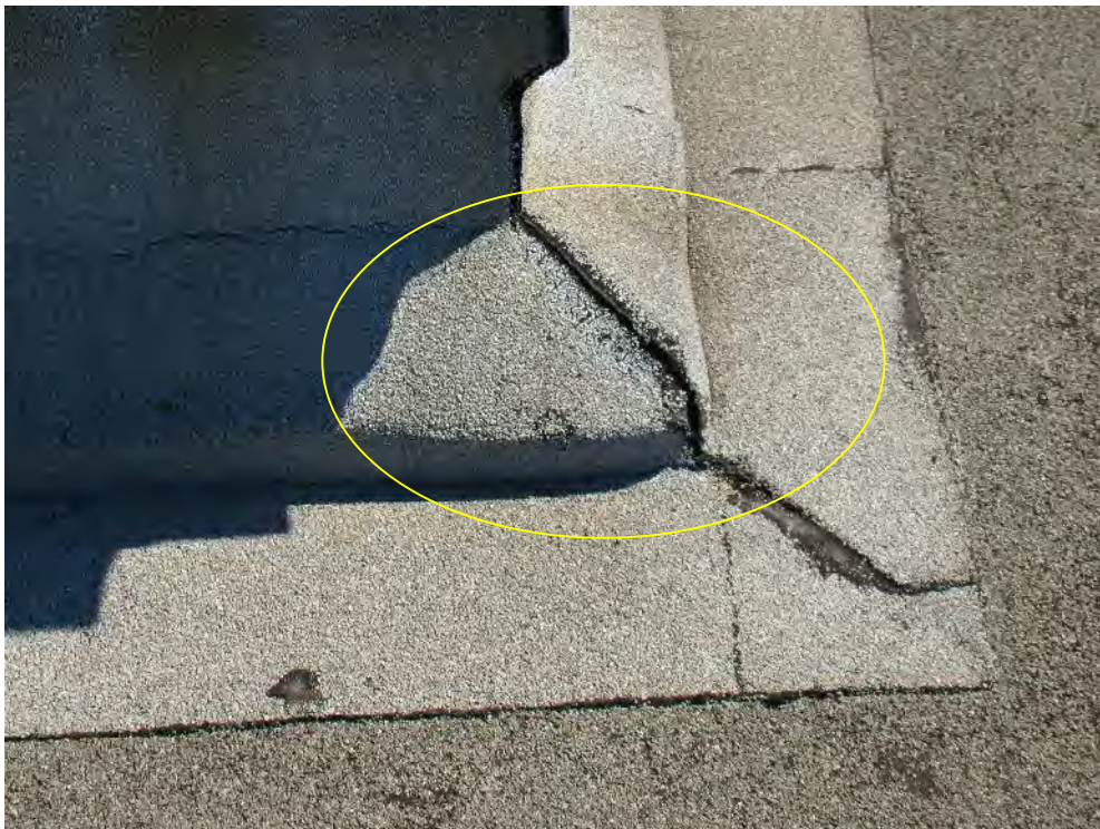
Photograph 40: Roof Area 1.2 – Delaminating membrane flashings were typically found at the corners of mechanical curb flashings.
