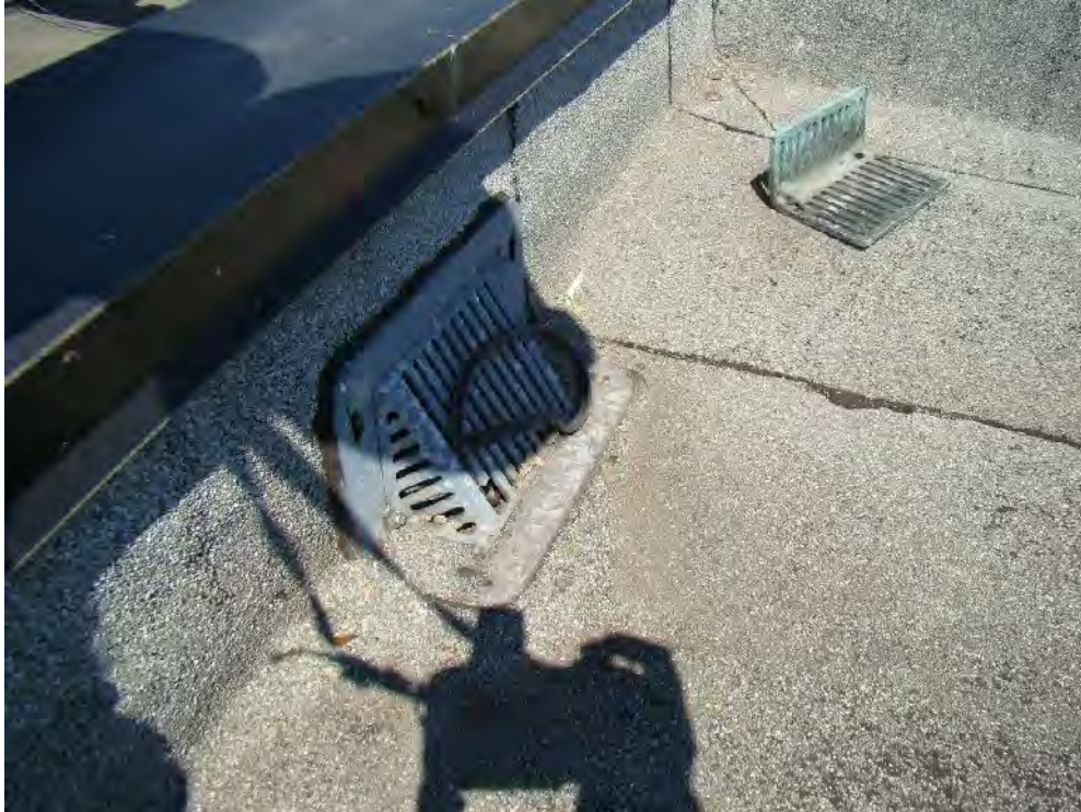
Photograph 65: Roof Area 2.3 – Minor debris accumulation at drainage scupper.
