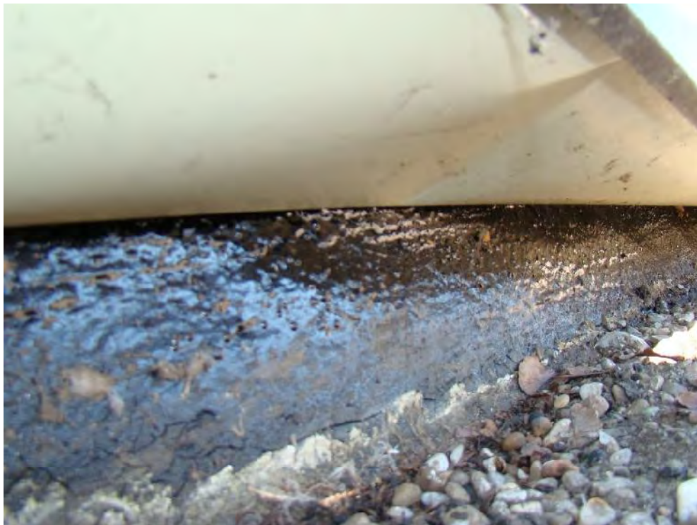
Photograph 6: Roof Area 1.1 – Membrane flashings where exposed for review appeared in serviceable condition with the asphalt glaze coating still in tact.
