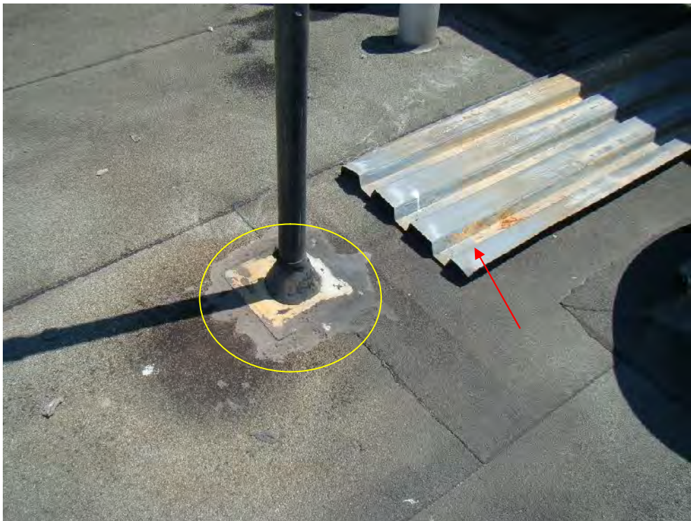
Photograph 78: Roof Area 3.1 – The existing stack penetration in the central portion of the roof is not adequately flashed into the roof system and is likely a major source of water entry. Construction debris from the adjacent construction was also observed scattered throughout the roof area.
