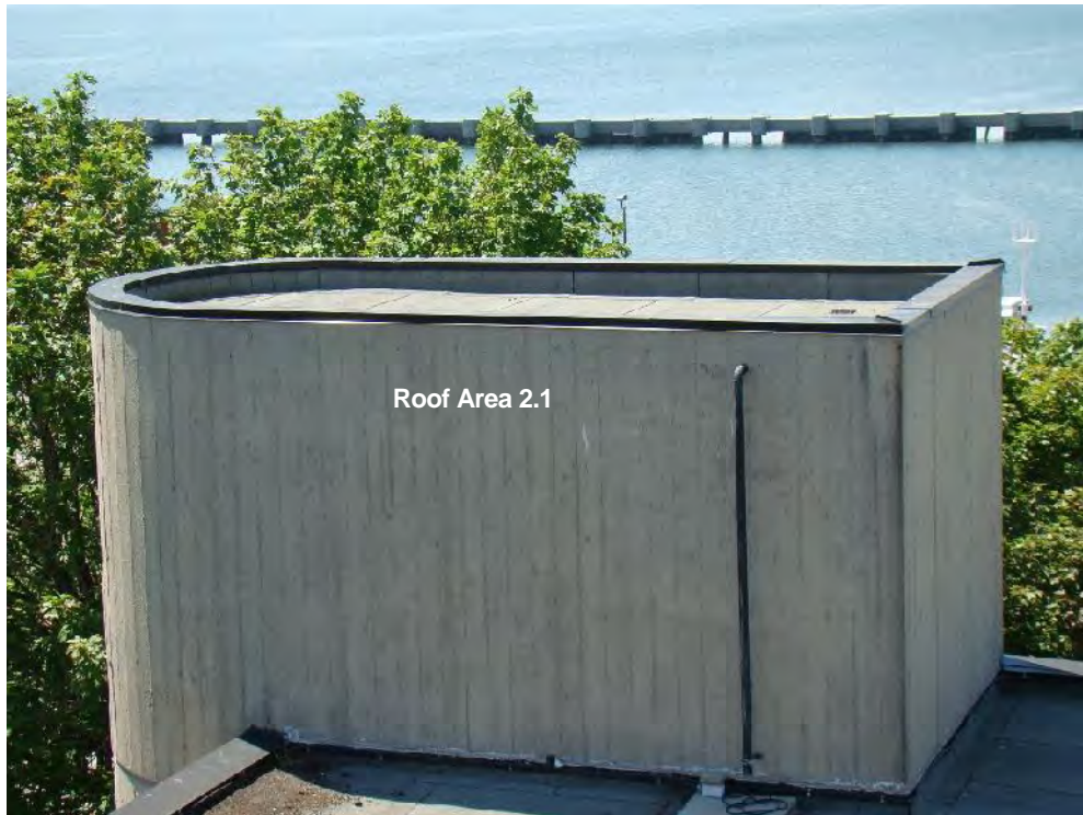
Photograph 53: Roof Area 2.1 – This small roof area is situated over the west stairwell and consists of a modified bitumen membrane system installed in the early to mid 1990's.
