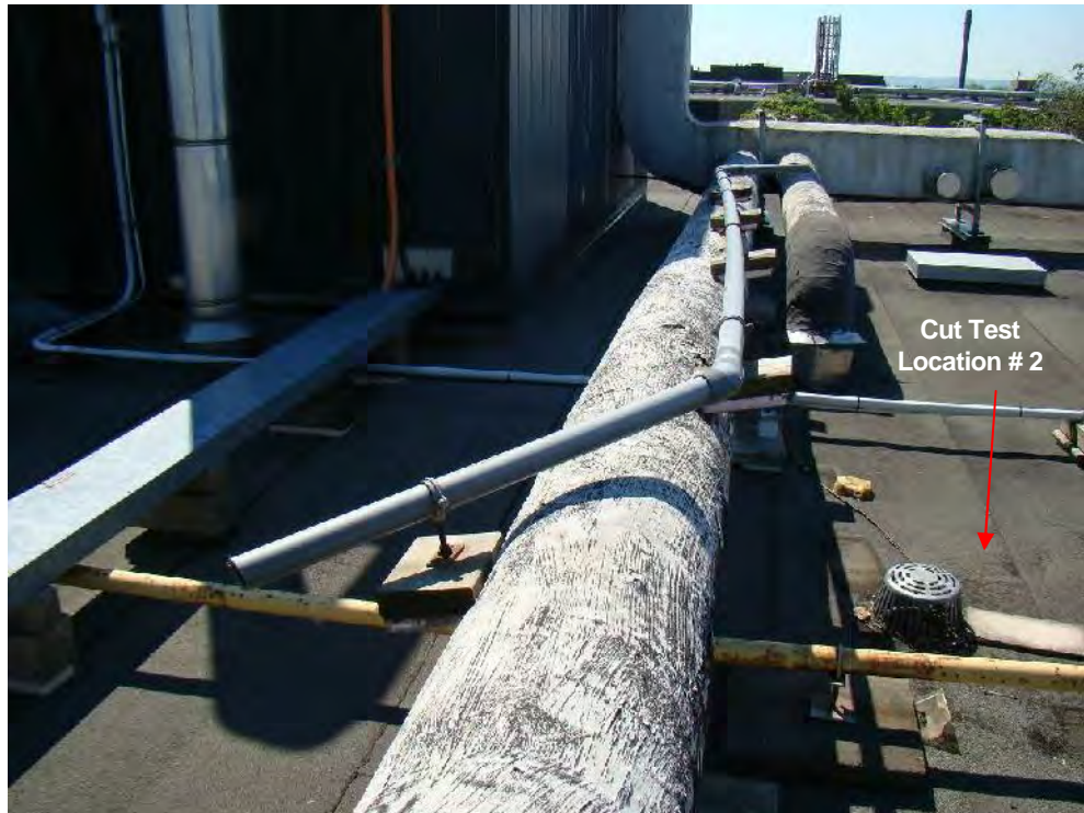
Photograph 31: Roof Area 1.2 – Test Cut #2 - The second test location was in the field of the roof adjacent to the west roof drain.
