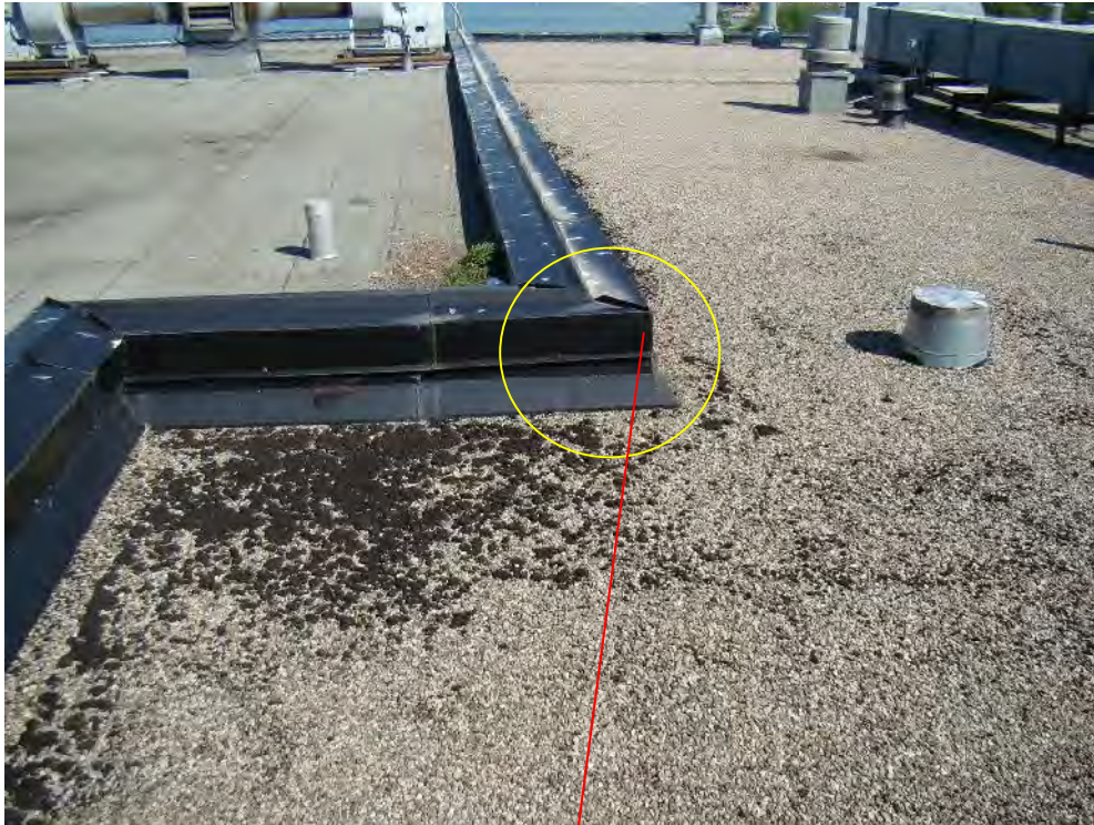
Photograph 7: Roof Area 1.1 – View of expansion joint between original building and east addition. Yellow circle indicates location where deteriorating flashings were found. See next photo.
