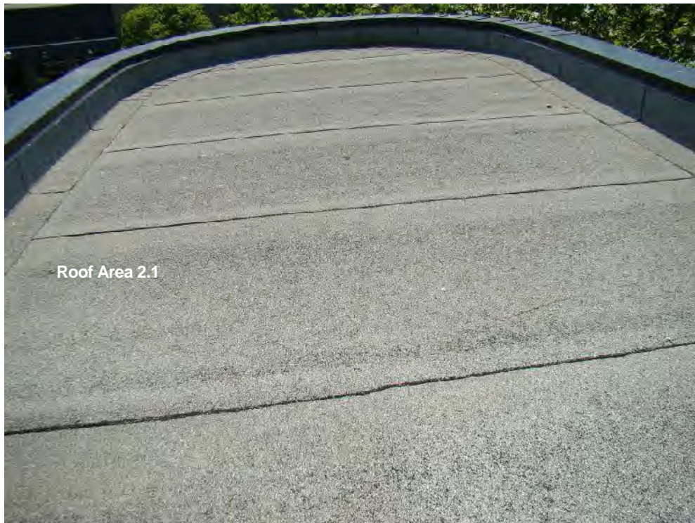
Photograph 54: Roof Area 2.1 – Overall view at roof level showing general granule surface loss.
