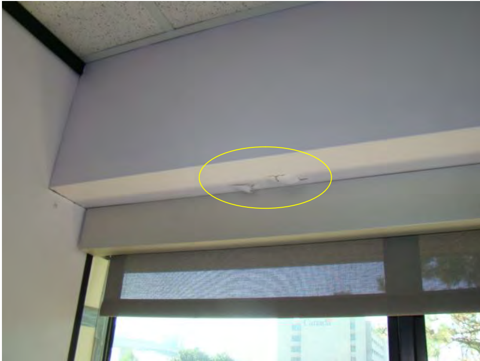
Photograph 17: Roof Area 1.2 (Interior) – Water stained drywall bulkhead above window in office S203 along the south perimeter of the building.
