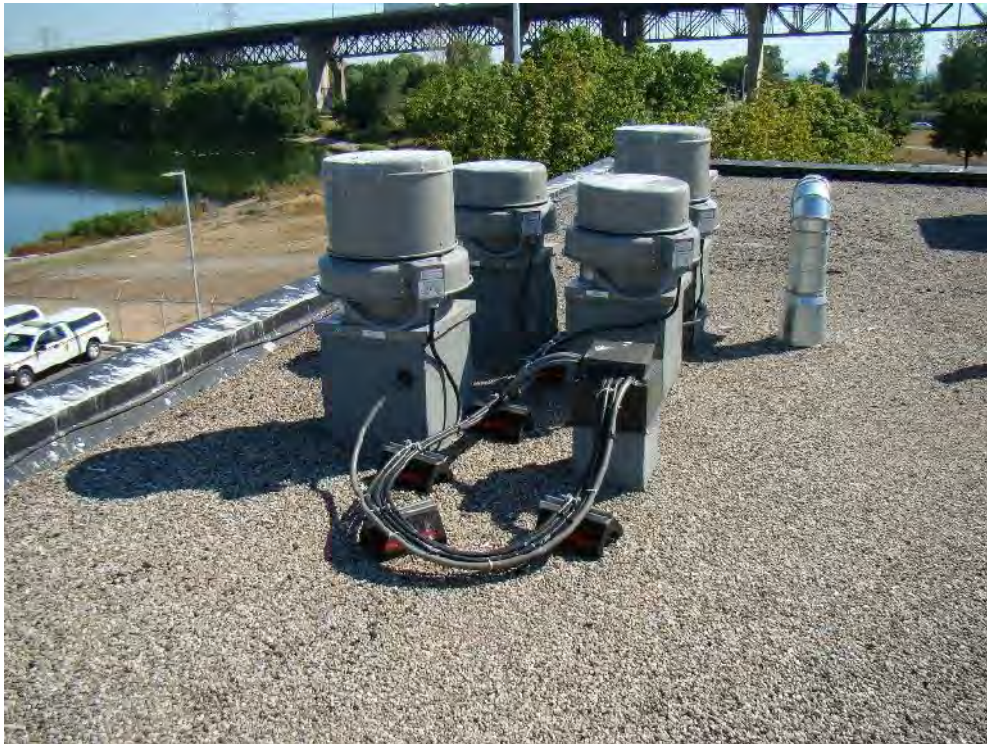
Photograph 9: Roof Area 1.1 – Various pieces of new mechanical equipment have been installed in the northeast corner of the roof and appear to have been flashed into the existing roof using acceptable materials and installation methods.
