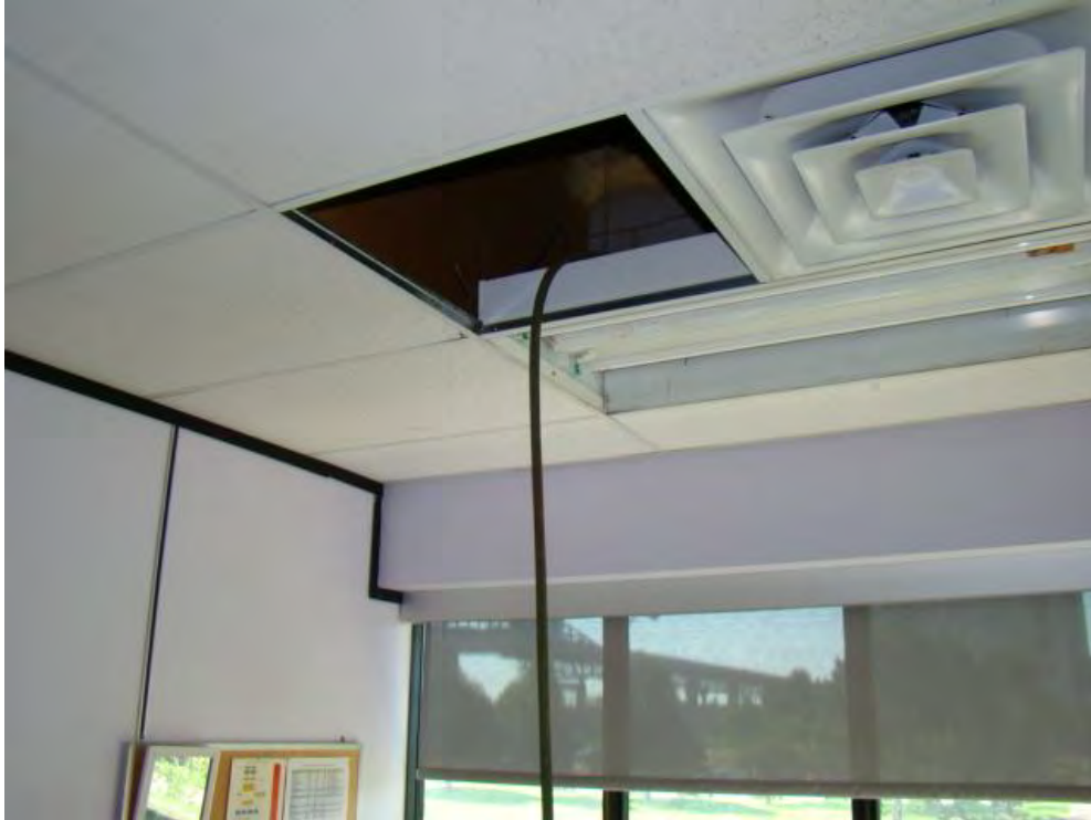
Photograph 19: Roof Area 1.2 (Interior) – Ongoing leakage above central portion of office S249. This location is directly below the ongoing construction of the mechanical room addition (see photographs 2 and 20). Occupants noted that leaks did not exist prior to construction.
