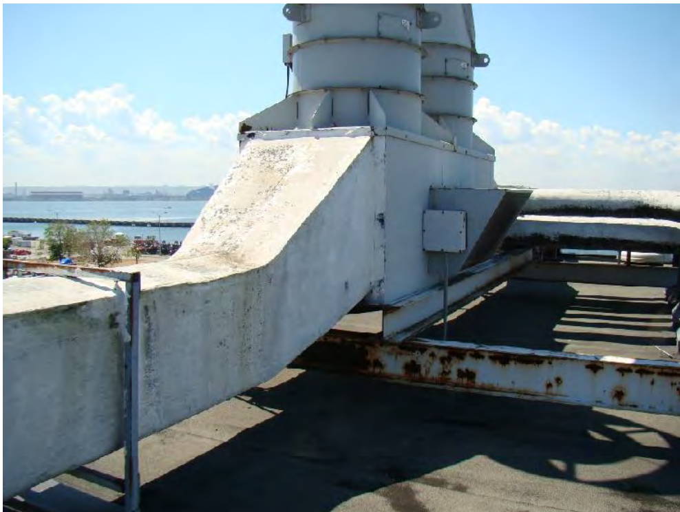
Photograph 68: Roof Area 3.1 – The roof is covered with a heavy concentration of mechanical equipment and ductwork which would tend to increase roof replacement costs significantly.
