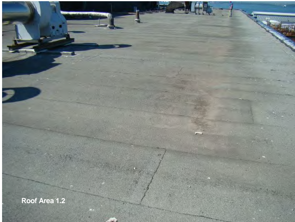
Photograph 13: Roof Area 1.2 – View looking west along the north portion of the roof area. This roof area is situated over the majority of the second floor level and consists of a modified bitumen membrane system installed in the early to mid 1990's.
