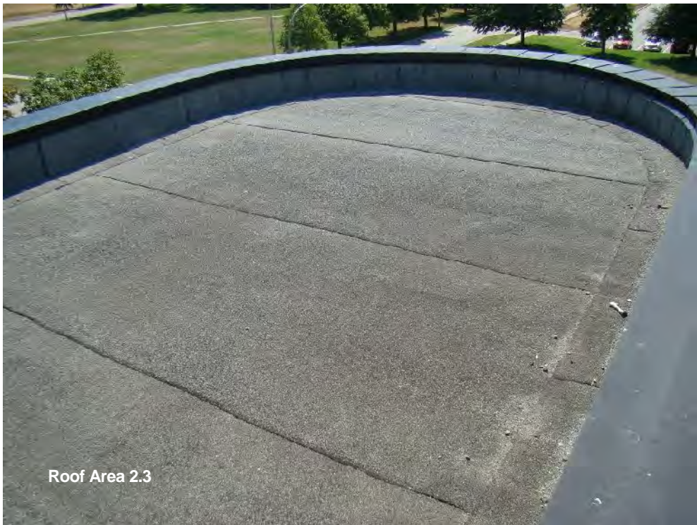
Photograph 62: Roof Area 2.3 - This small roof area is situated over the east stairwell and consists of a modified bitumen membrane system installed in the early to mid 1990's.
