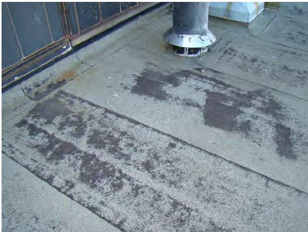
Photograph 33: Roof Area 1.2– The membrane exhibits widespread and severe granule surface loss and weathering.
