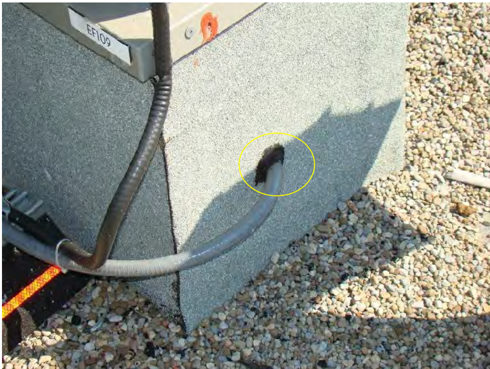
Photograph 10: Roof Area 1.1 – Electrical conduit penetrations at the new equipment have been fed through the sides of the support curbs which will tend to be an ongoing maintenance item.
