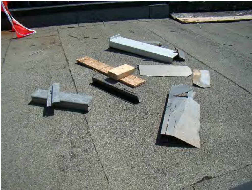
Photograph 61: Roof Area 2.2 – Construction debris is scattered throughout roof area.
