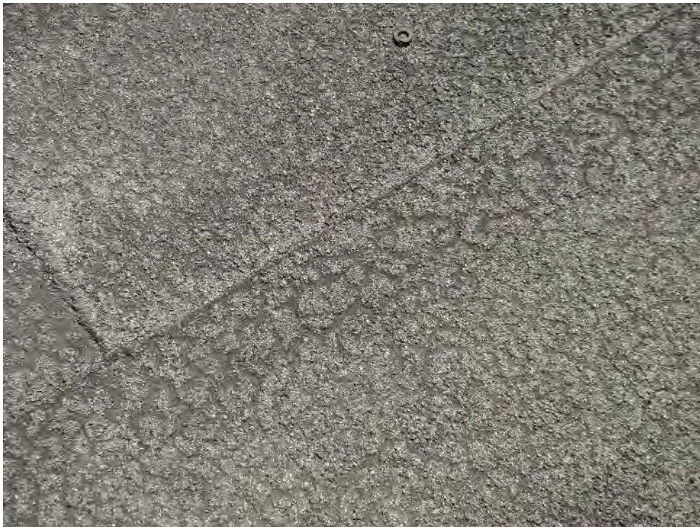
Photograph 36: Roof Area 1.2 – Severe surface deterioration and cracking, typical of advanced aging.
