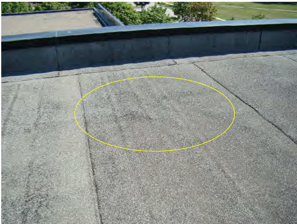
Photograph 64: Roof Area 2.3 – Membrane wrinkling and blistering was evident within the field of the roof.
