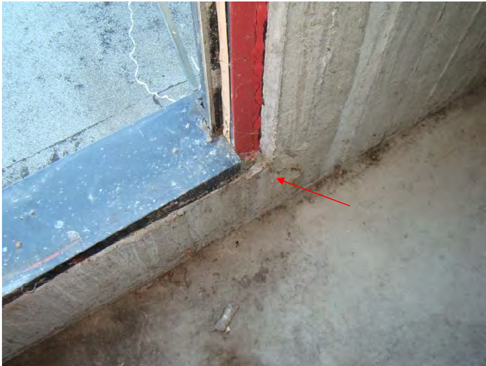
Photograph 43: Roof Area 1.2 – Evidence of water entry was observed along the base of the door into the stairwell which could be related to the sealant deterioration or due to inadequate weather stripping along the bottom of the door.
