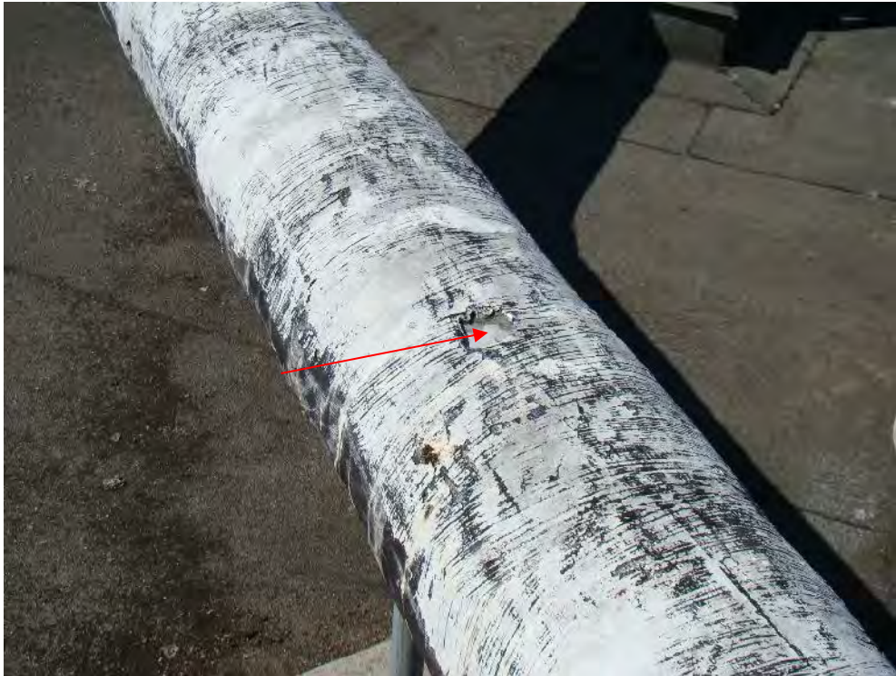
Photograph 49: Roof Area 1.2 - The existing waterproofing application over mechanical ductwork was assessed to be in poor condition (cracking, splitting) resulting in several instances of water infiltration and saturation of the underlying insulation.
