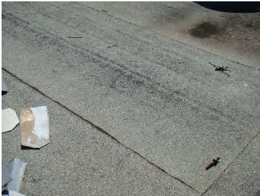
Photograph 58: Roof Area 2.2 - The cap sheet membrane appears weathered and worn with general granule surface loss throughout.
