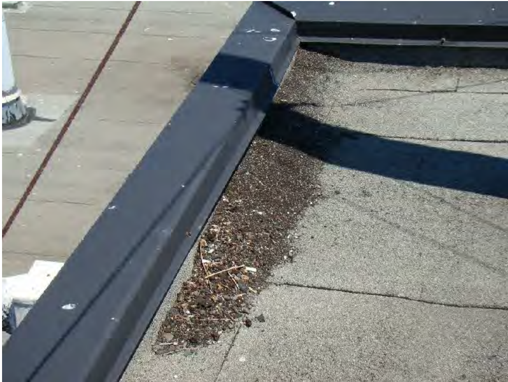
Photograph 75: Roof Area 3.1 – Overall drainage patterns appear inadequate with evidence of ponding throughout along with organic debris build up at perimeters.
