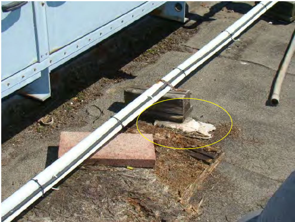
Photograph 52: Roof Area 1.2 - Polystyrene protection pads under various wood blocking supports have disintegrated due to UV exposure. The lack of adequate protection causes the wood blocks to damage the membrane.
