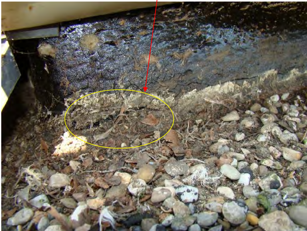
Photograph 8: Roof Area 1.1 – View of cracked membrane flashings at the south end of the expansion joint.
