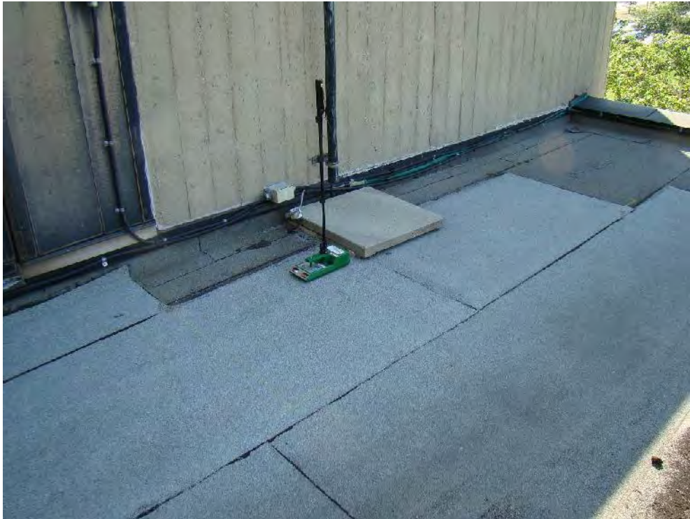
Photograph 25: Roof Area 1.2 – Moisture detected adjacent to the stairwell wall transition above office S208. This location is actively leaking notwithstanding recent membrane repairs (see photo 18).
