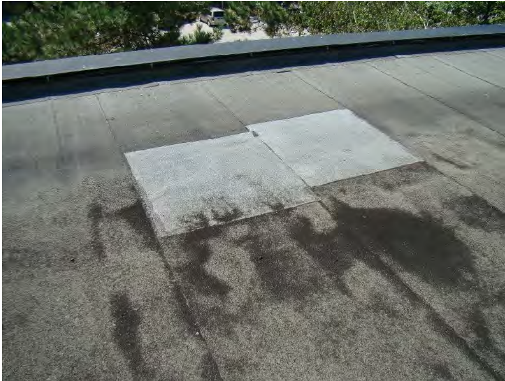
Photograph 35: Roof Area 1.2 – Granule surface loss due to prolonged ponding.
