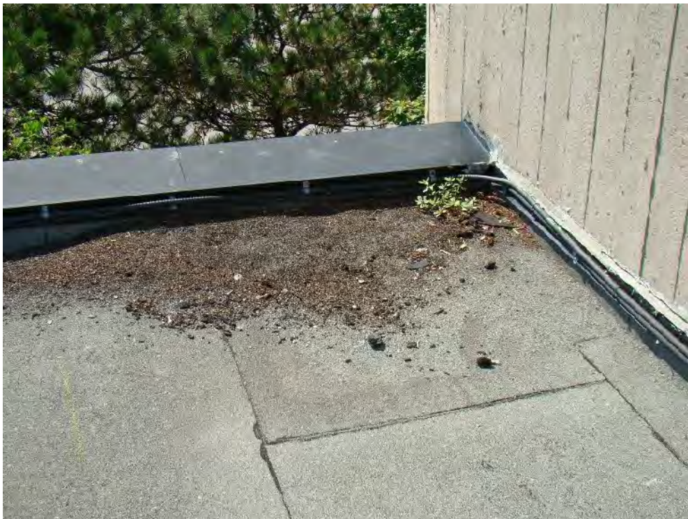
Photograph 50: Roof Area 1.2 – Heavy organic debris and vegetation accumulation is present at corner transitions which have the potential to result in accelerated membrane deterioration.
