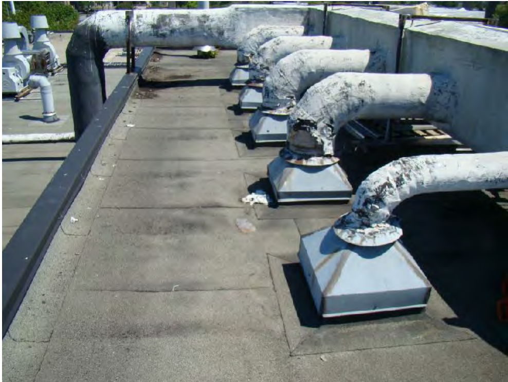
Photograph 79: Roof Area 3.1 – The existing waterproofing application over mechanical ductwork was assessed to be in poor condition.
