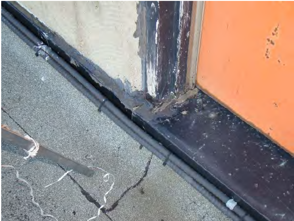
Photograph 42: Roof Area 1.2– Sealant failure exists at the door frame along the north wall of the east stairwell penthouse.
