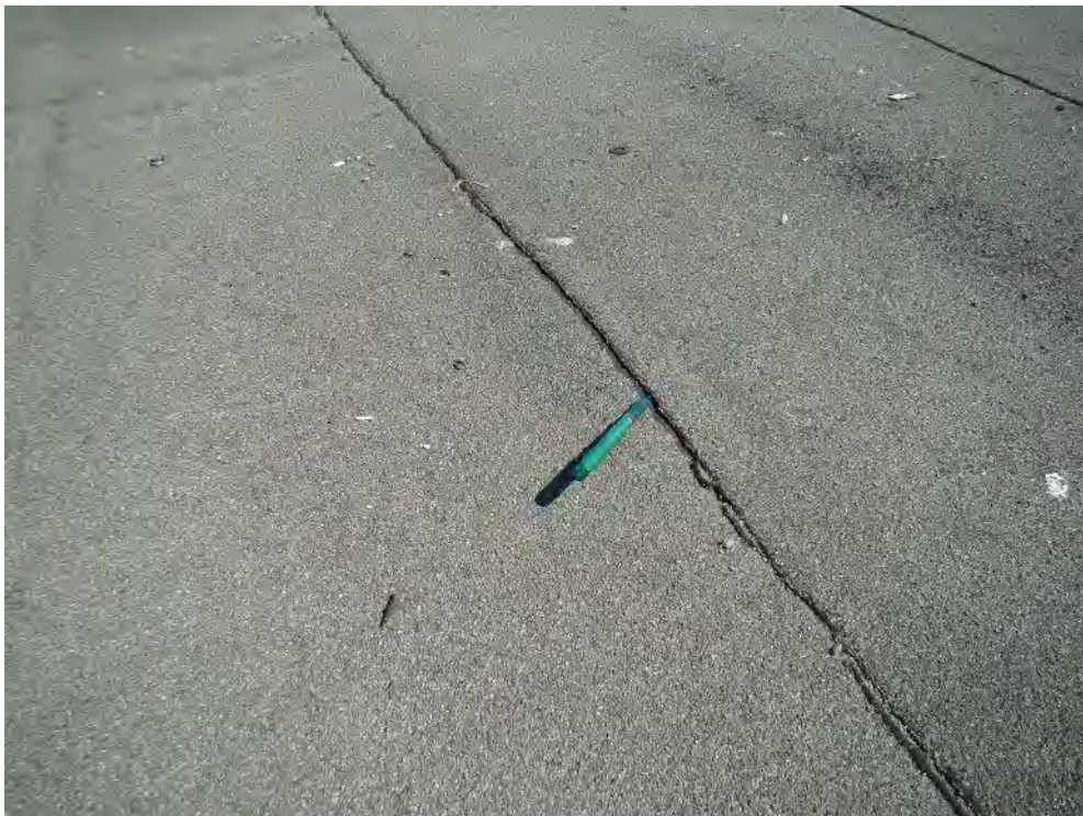
Photograph 38: Roof Area 1.2 – Severe blistering is causing developing membrane laps to delaminate and be susceptible to water entry.
