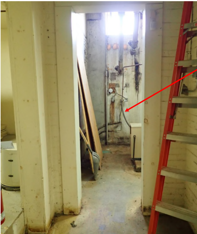
Entrance to sump pump and furnace Room
