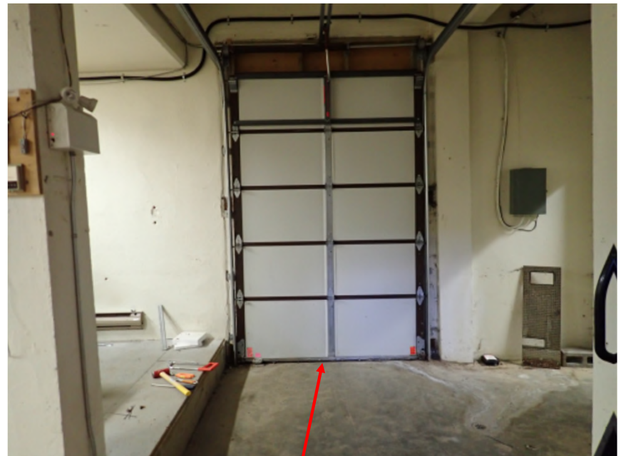
Basement door to exit ramp
