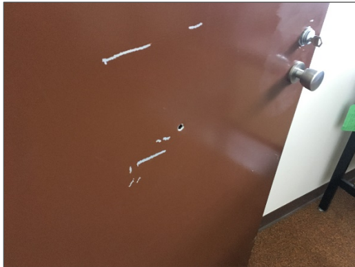
Non-asbestos brown paper inside door within the Office (Location 7)
