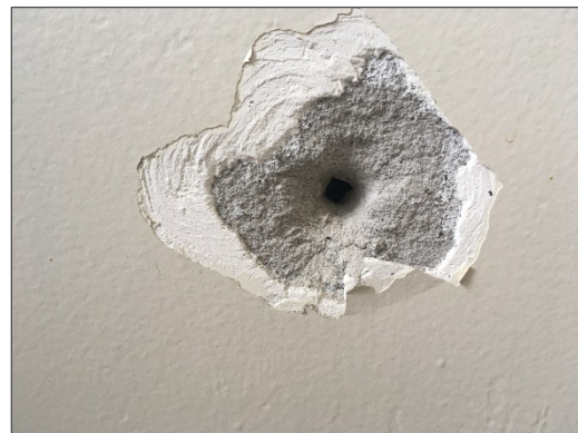
Destructive testing in plaster wall within the Kitchen (Location 2)
