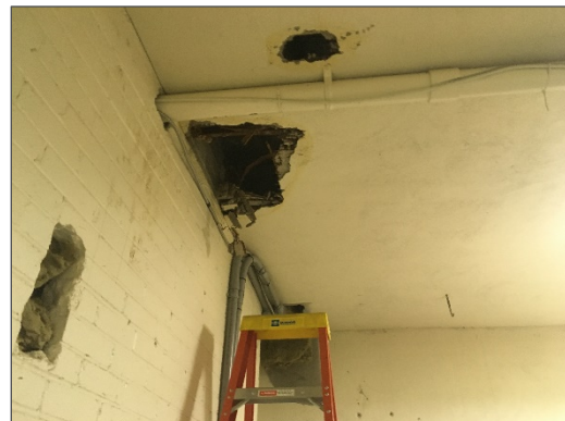
Non-asbestos grey cementitious grey plaster present within the Storage Room (Location 9)
