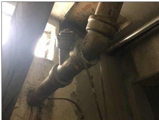
Lead caulking in pipe line within the Sump Pump Room (Location 10)
