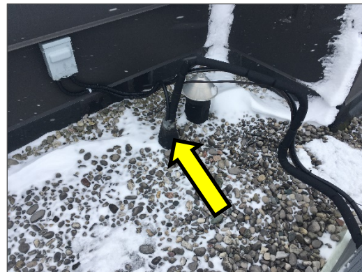
Non-asbestos tar around roof vent on the Roof
