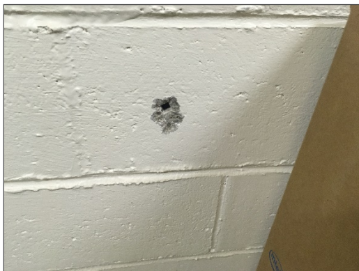
Destructive testing in masonry block wall within the Furnace Room (Location 4)
