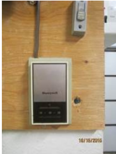
ME-017 – Wall mounted thermostat (baseboard heaters).
