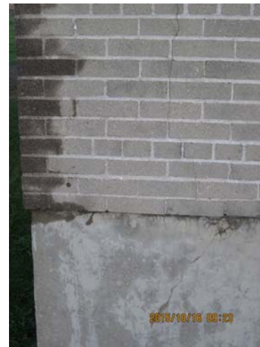
AR-020 – Crack through foundation and lower portion of masonry wall.
