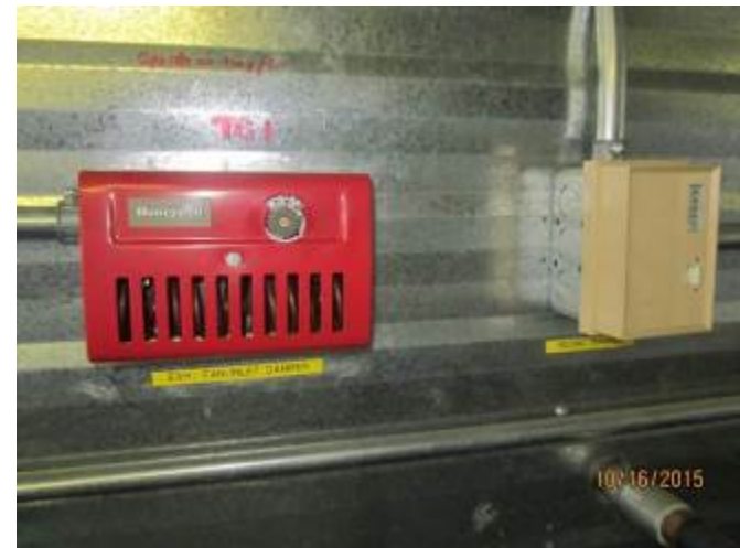
ME-020 – Thermostats for heat control in the emergency generator portable unit.
