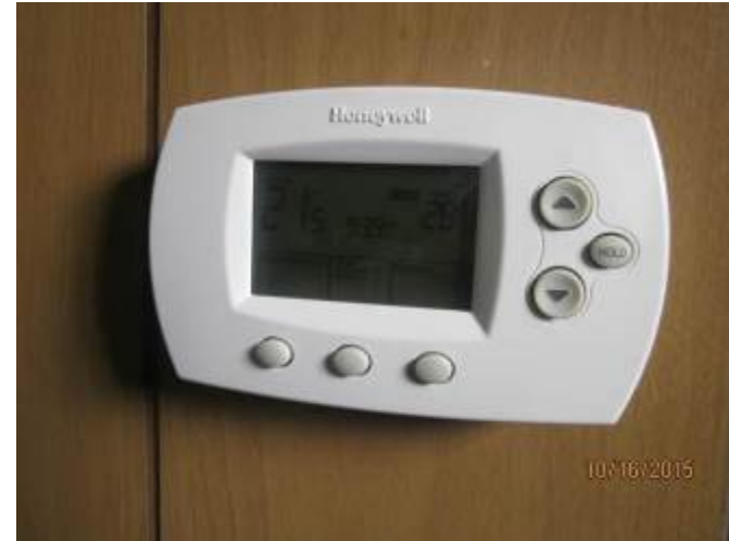
ME-018 – Wall mounted thermostat (AHU).
