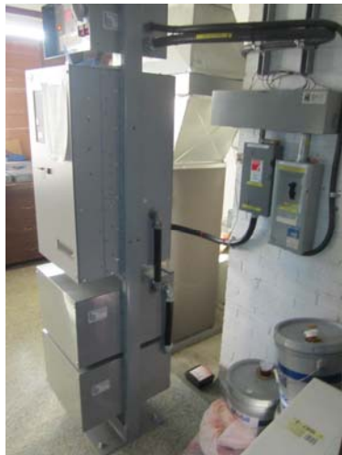
EL-007 – UPS installed in furnace room near heat source and flammable materials.
