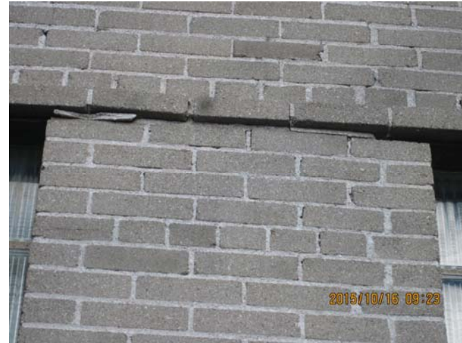
AR-022 – Deteriorating mortar at ends of rusting lintels.
