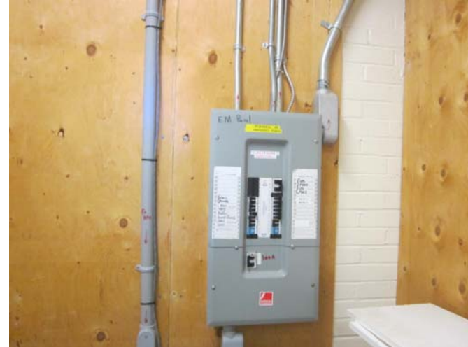
EL-006 – Overloaded emergency power panel.
