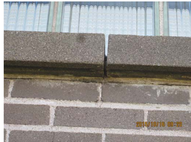
AR-024 – Open joint at concrete window sill.
