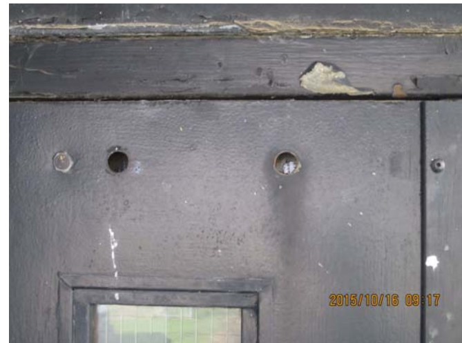
AR-028 – Unsealed holes at door outer surface.
