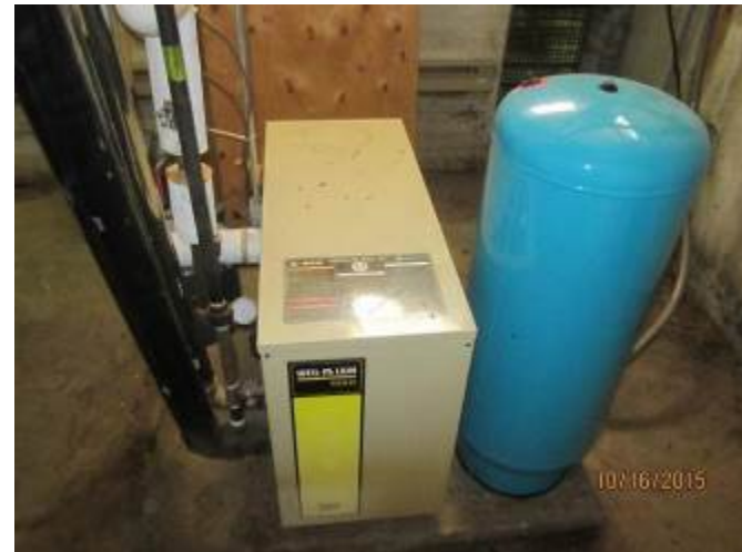
ME-008 – Weil-McLain decommissioned hot water boiler (yr. 1996).
