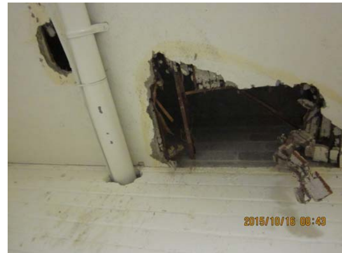
AR-036 – Several damaged areas of suspended plaster ceiling in northeast room of basement – reason unknown.
