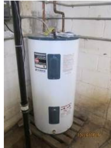
ME-026 – Electric domestic hot water tank (yr. 2006).
