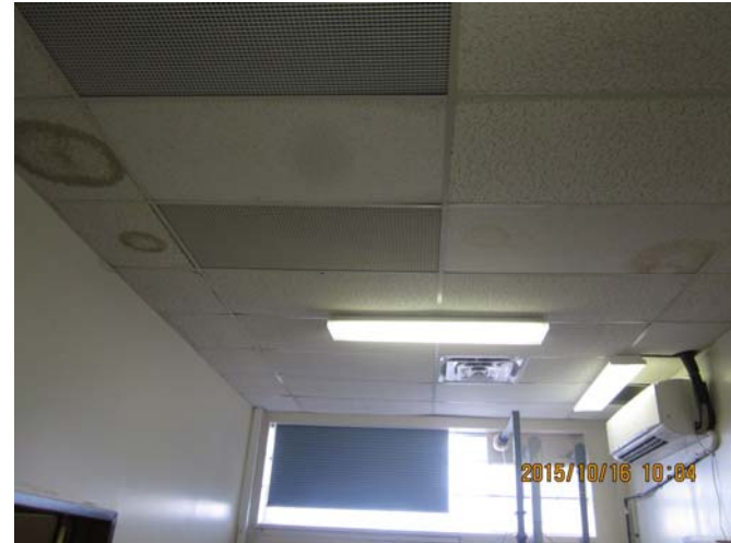
AR-038 – Water damaged ceiling tiles in office area.
