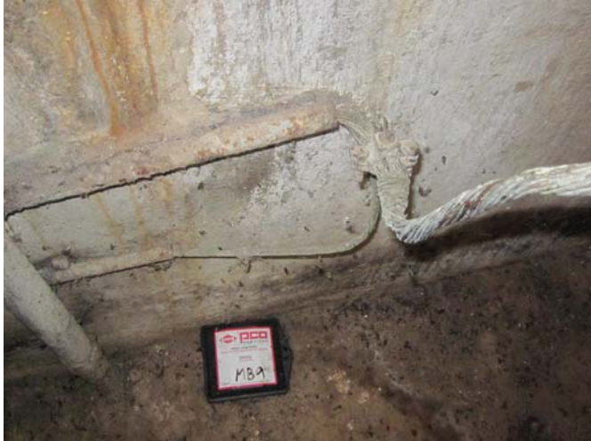
EL-005 – Corroded main facility electrical system grounding.
