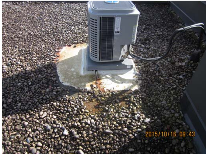
AR-029 – Deteriorated insulation pad below rooftop equipment.
