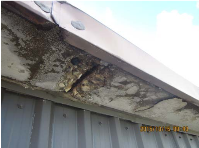
AR-013 – Spalled concrete and exposed rebar with corroded surface at underside of penthouse roof slab.
