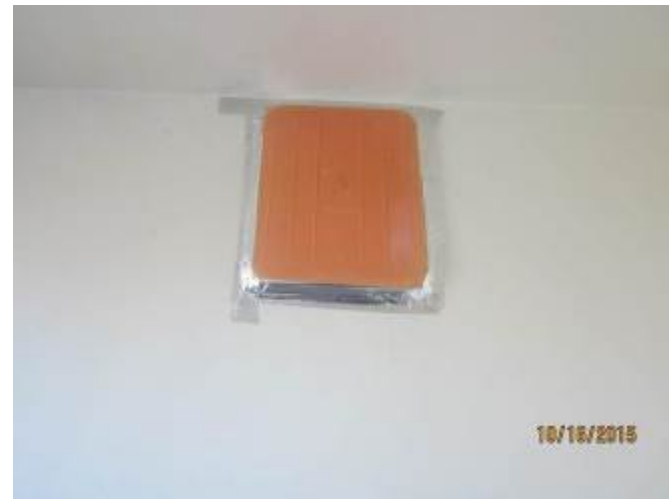
ME-016 – Obstructed exhaust fan (kitchen).
