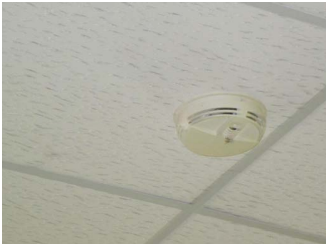
EL-023 – Integrated smoke detector to security system.
