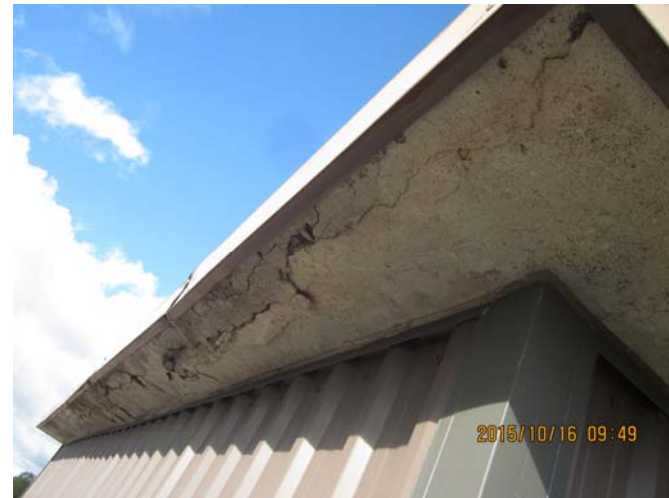
AR-012 – Deteriorated concrete at underside of penthouse roof slab.
