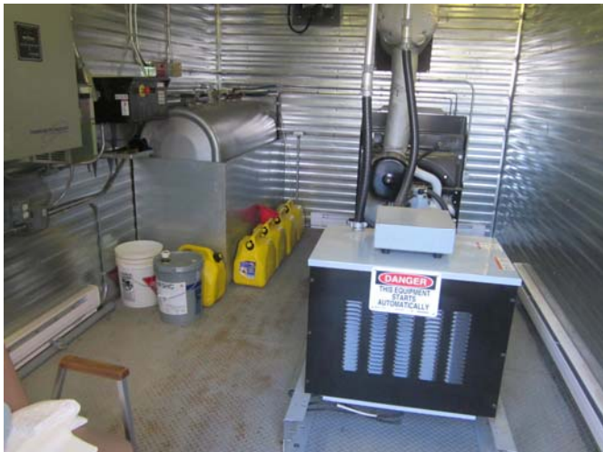
EL-011 – Emergency power generator system.
