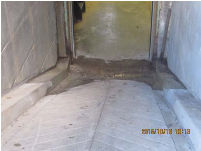
AR-011 – Water at bottom of basement access ramp.
