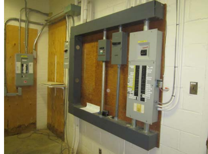
EL-002 – Main service equipment and troughs.
