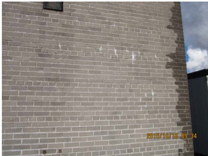
AR-019 – Stained masonry surfaces on east elevation.
