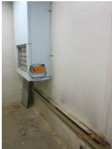
ME-003 - Electric baseboard heater (basement).
