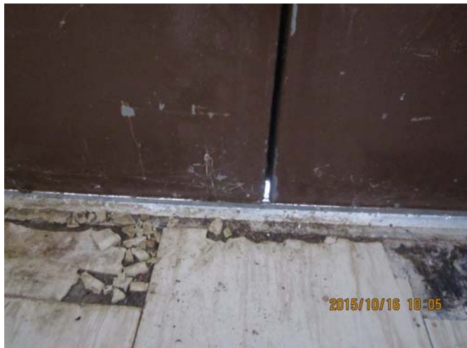
AR-039 – Deteriorating vinyl tile flooring and daylight visible at door edges and sills.
