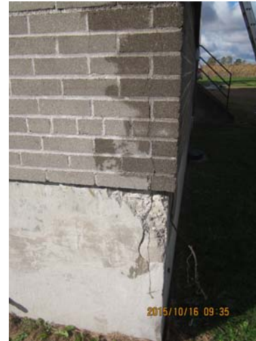
AR-006 – Deteriorated concrete at foundation corner.
