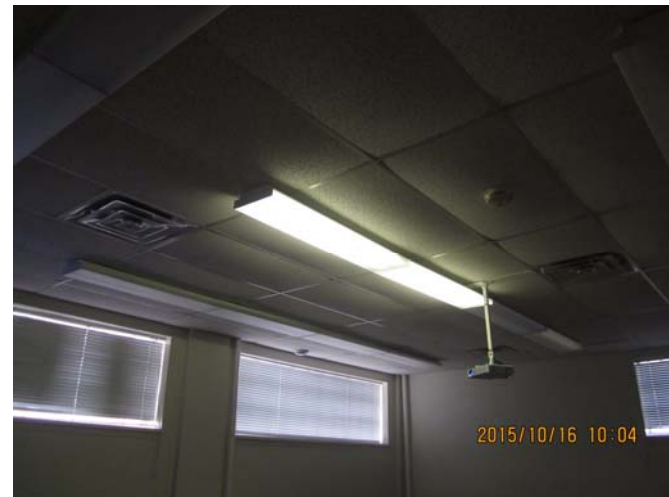
AR-040 – Warped ceiling tiles throughout classroom.
