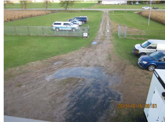
PS-002 – Standing water and vegetation growth at various locations throughout gravel paving.
