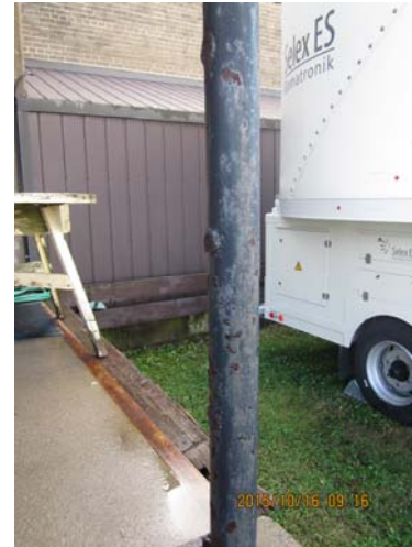
AR-014 – Deteriorated paint finish and corroded metal surfaces at loading dock canopy column.
