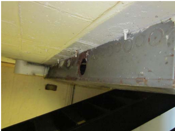
EL-003 – Example of rust-out on service equipment.
