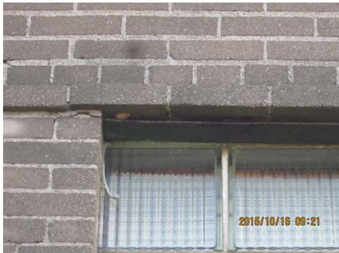
AR-023 – Rusting and deformed lintel and deteriorated sealant at glass block head.
