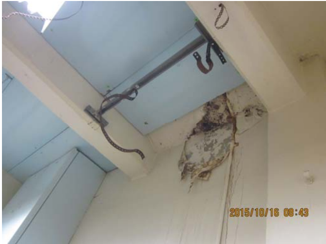
AR-009 – Water damage in basement electrical room - at underside of loading dock stair.
