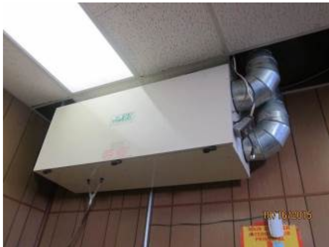
ME-015 – Heat recovery ventilator (disconnected).
