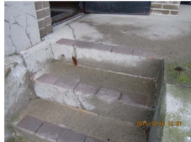
AR-008 – Loading dock stair with missing guard (right), cracked concrete with rusting rebar staining, and open joints at tile nosing - leakage below.
