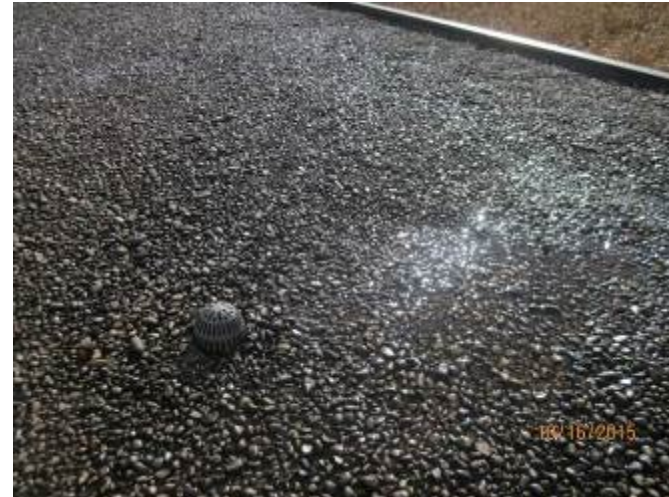
ME-022 – Roof drain collector.
