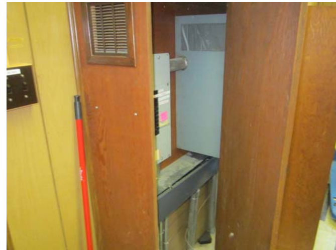
EL-004 – Electrical equipment installed in wood cabinets.
