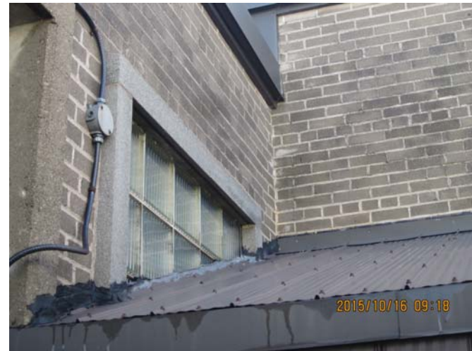
AR-032 – Metal roofing not flashed into wall along edge.
