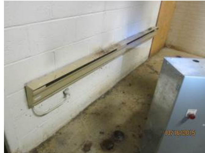
ME-002 – Electric baseboard heater (basement).
