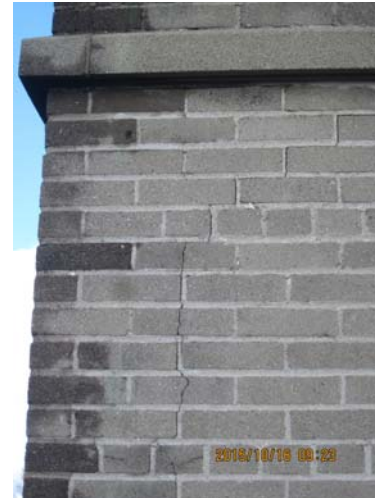
AR-018 – Crack through upper portion of masonry wall.
