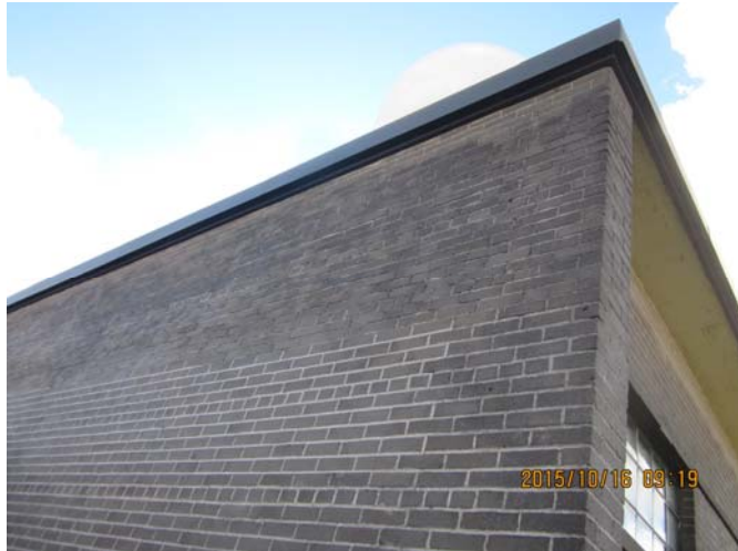
AR-017 – Deteriorated mortar joints at north elevation (area above classroom ceiling).
