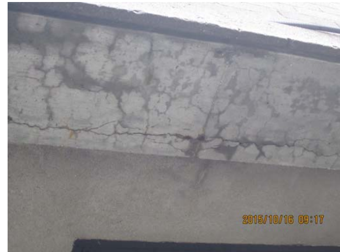
AR-016 – Deteriorated concrete at underside of loading dock canopy.
