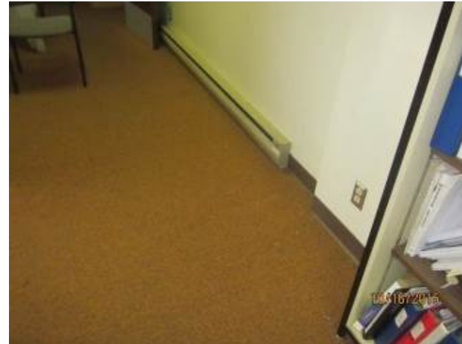
ME-006 - Electric baseboard heater (hallway).
