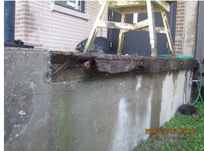
AR-010 – Deteriorated wood bumper at loading dock edge.
