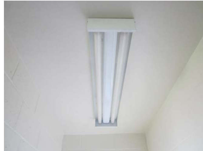
EL-018 – Typical older type lamps/no lens.
