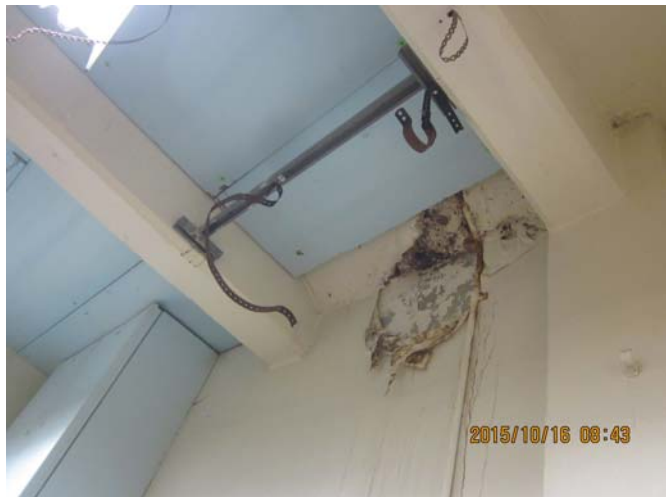
AR-035 – Leakage and damaged finishes in electrical room below exterior stair. Also, inconsistent application of insulation.
