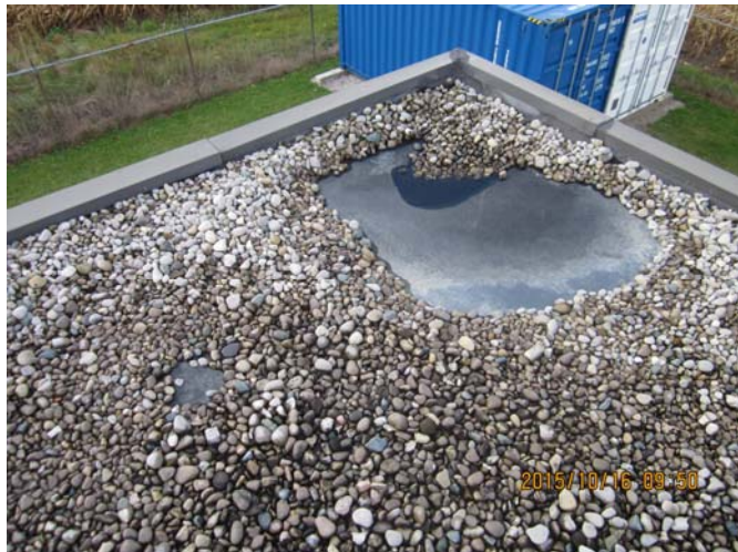
AR-031 – Ballast scouring at southwest corner of upper roof area.
