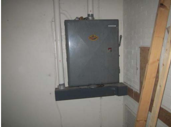
EL-001 – Main electrical 400A disconnect.
