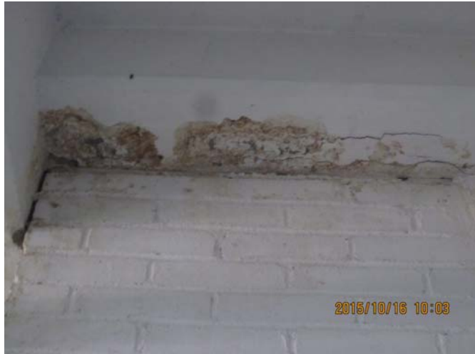
AR-037 – Water damage at underside of penthouse.
