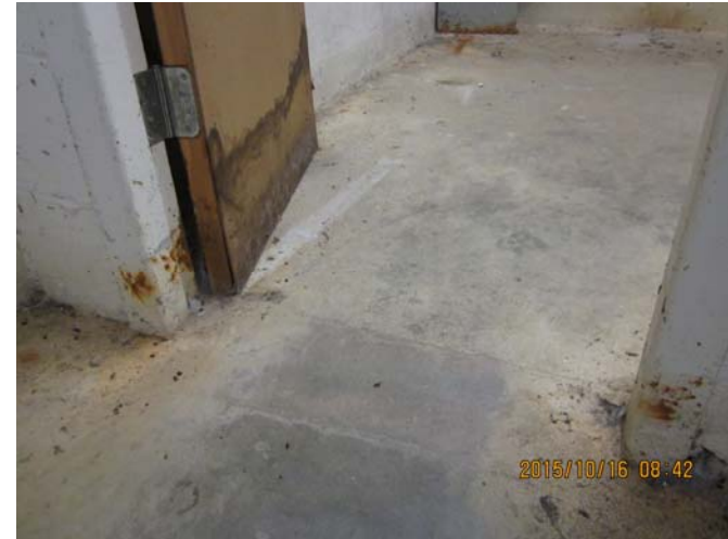
AR-034 – Water damaged door, frame, finishes and electrical equipment at basement electrical room adjacent to access ramp.
