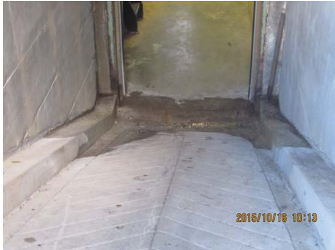
AR-033 – Leakage/seepage at bottom of basement access ramp.
