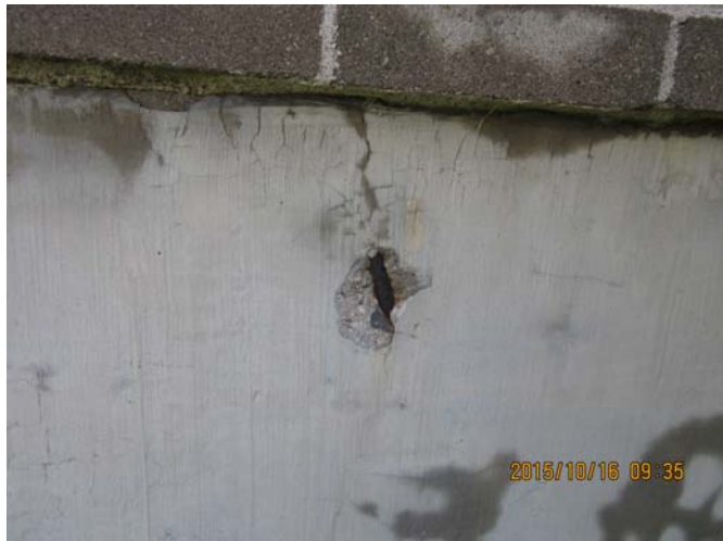
AR-007 – Spalled concrete and exposed rebar with corroded surface at foundation.
