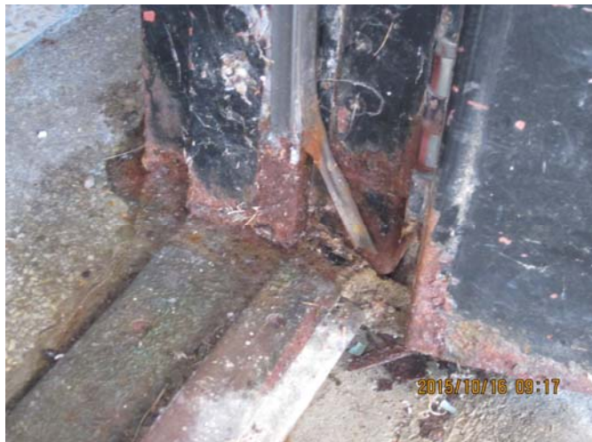
AR-027 – Deteriorated metal at bottom of door and frame.
