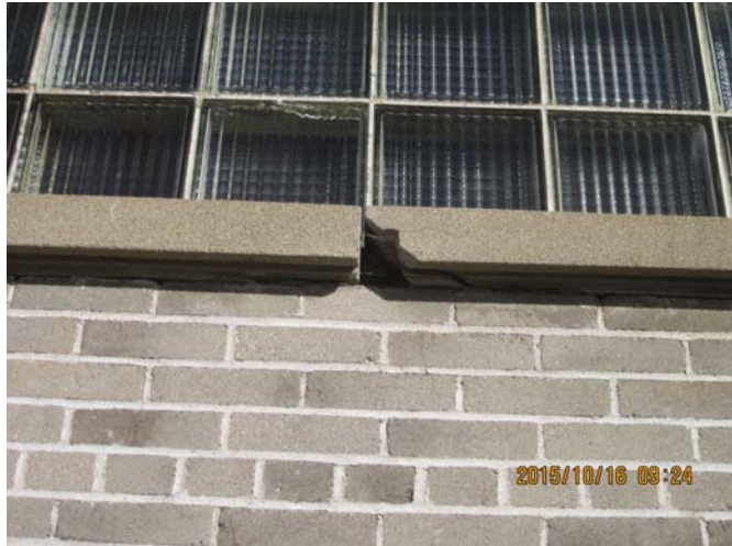
AR-021 – Broken concrete window sill.
