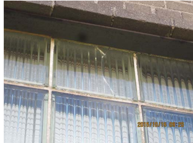
AR-026 – Cracked glass block.
