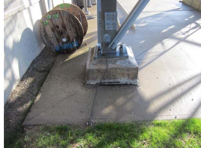
EL-010 – Typical lightning grounding/protection installation.
