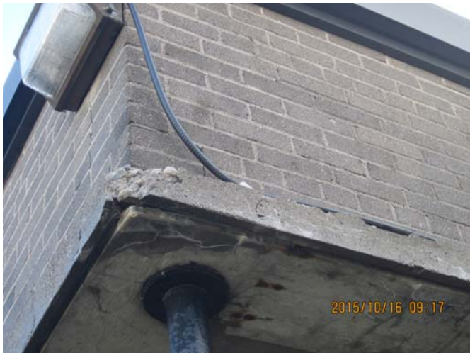
AR-015 – Deteriorated concrete along top edge of loading dock canopy.
