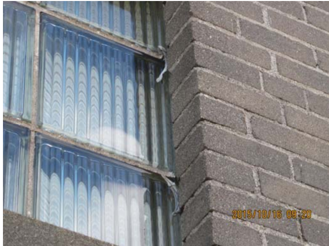
AR-025 – Deteriorated sealant at glass block jamb.
