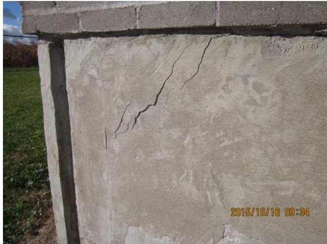
AR-005 – Spalling concrete at foundation.
