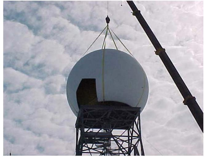
This is how radome was put on. Taking it off intact with one (or two) panels removed is easiest way to take it down. Further breakdown of radome at ground level.
