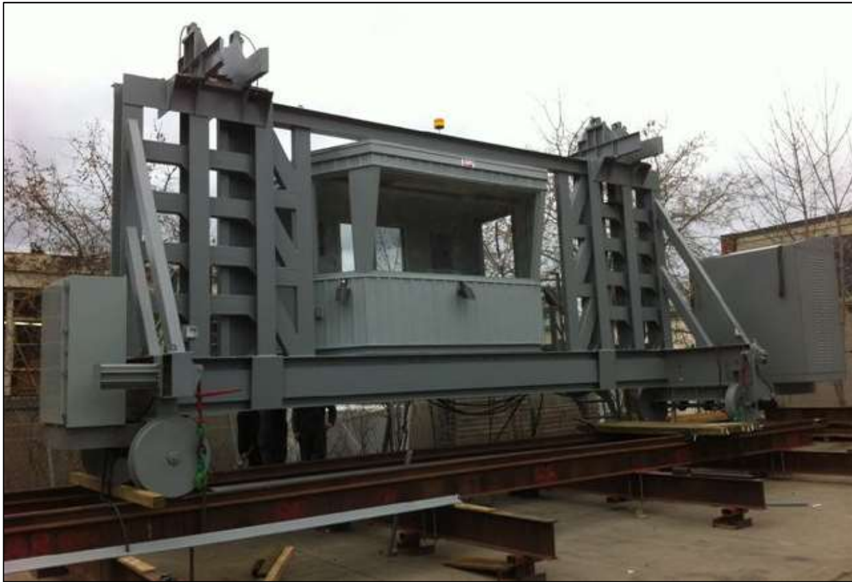
Figure 17 - Frame of stoplog lifter under construction, before booms were installed. Photo: J. L. Richards 2011.
