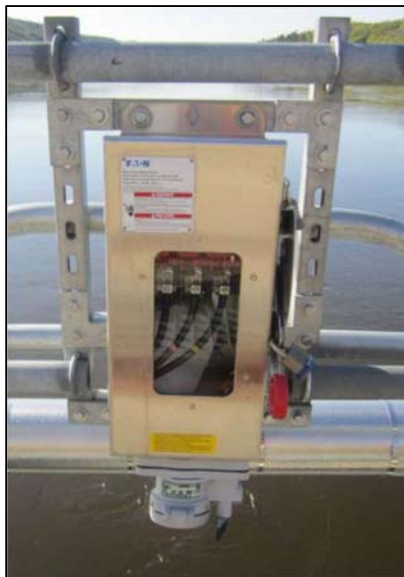
Figure 21 - Stoplog lifter is powered through 600V outlets located at intervals along the railing on the upstream edge of the operating deck. The power cable is plugged into the bottom of these outlets.
