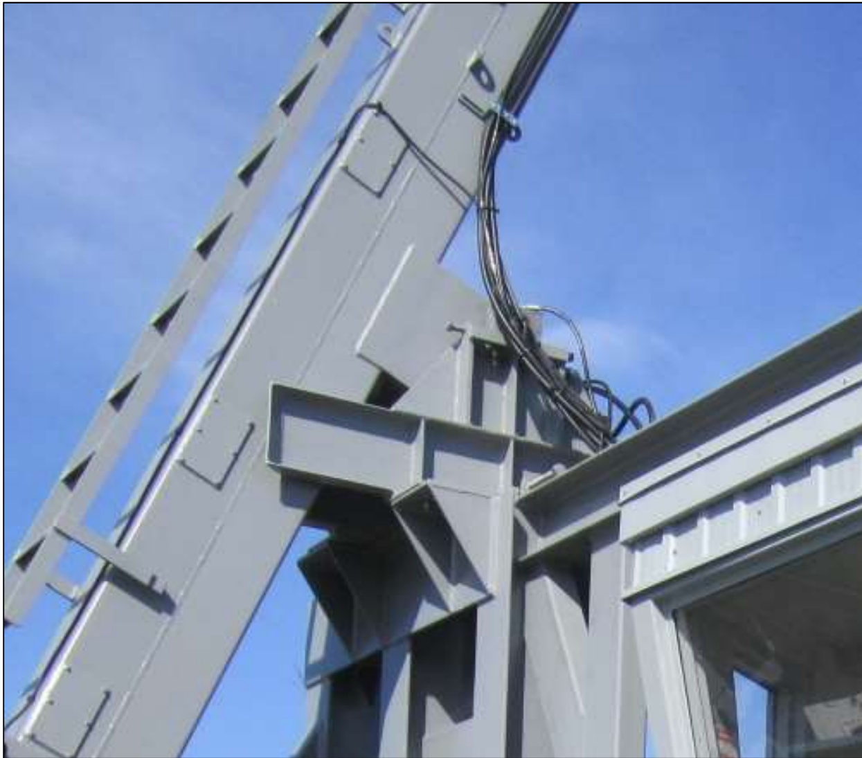
Figure 11 - Detail of connection between boom and frame. This is a detail of the boom currently having problems.
