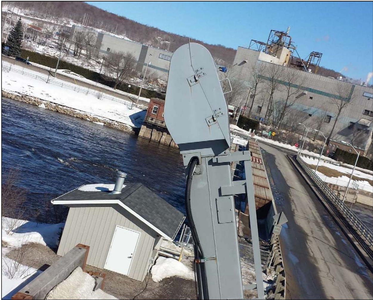
Figure 14 - Detail of housing on top of booms for hydraulic hose reel and electric cable reel. Photo: Garage PEM Barrette, 2015.
