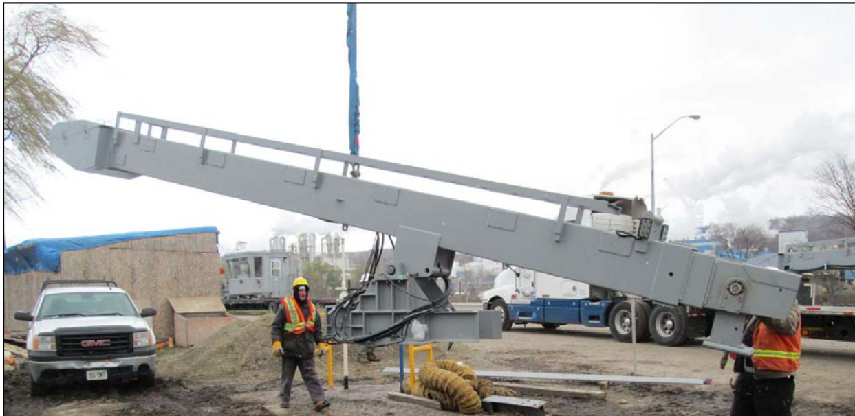
Figure 18 - Boom being installed at the dam in 2012. Photo: J. L. Richards.
