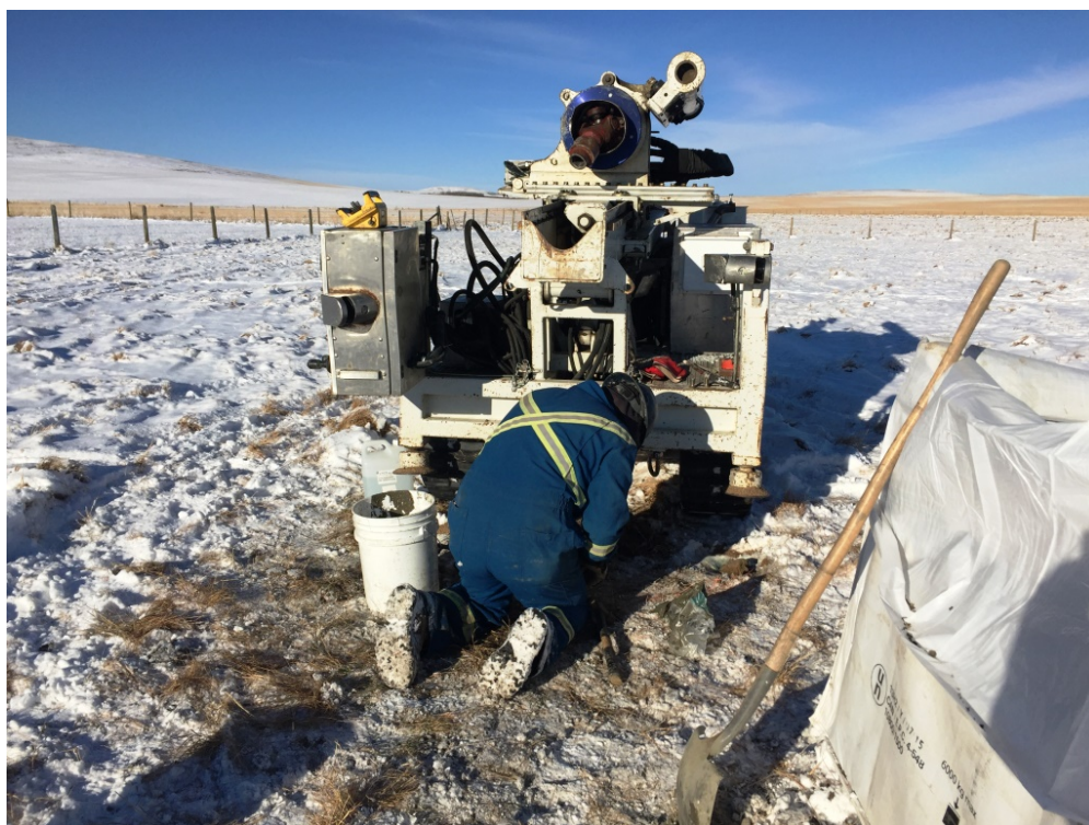
Photograph 8: Northern view of drill rig crew completing installation of background monitoring well GMW18.
