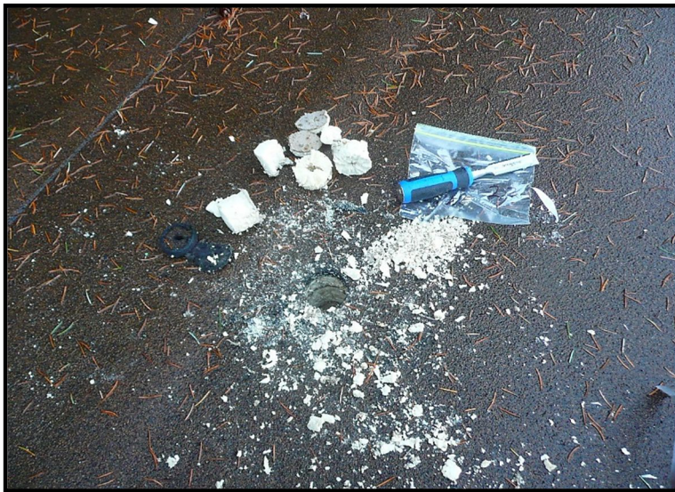
Roofing materials core layer Sample 17A-TSB-22 collected from the northeast portion of the Technical Services Building.
