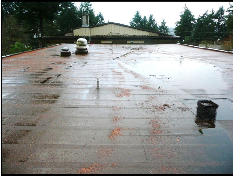
Looking southward over the roof of the Technical Services Building.
