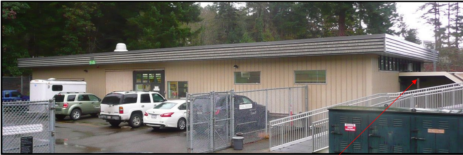
Technical Services Building west and south elevations with south staircase canopy (looking northeast).
