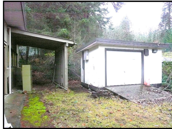
The east attached open ended canopy and detached storage shed (looking north).
