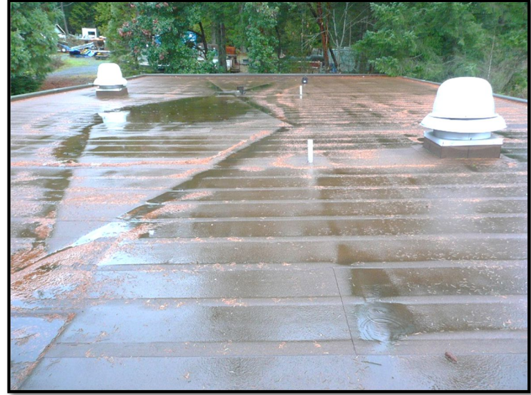
Looking northward over the roof of the Technical Services Building.
