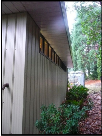
Technical Services Building north elevation (looking westward).
