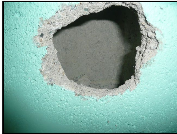
Exploration of the south concrete masonry unit wall of the Metal Storage Room #10. No indication of potential vermiculite insulation was found.
