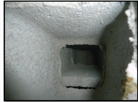
Exploration of the south concrete masonry unit wall of the Metal Storage Room #10. No indication of potential vermiculite insulation was found.
