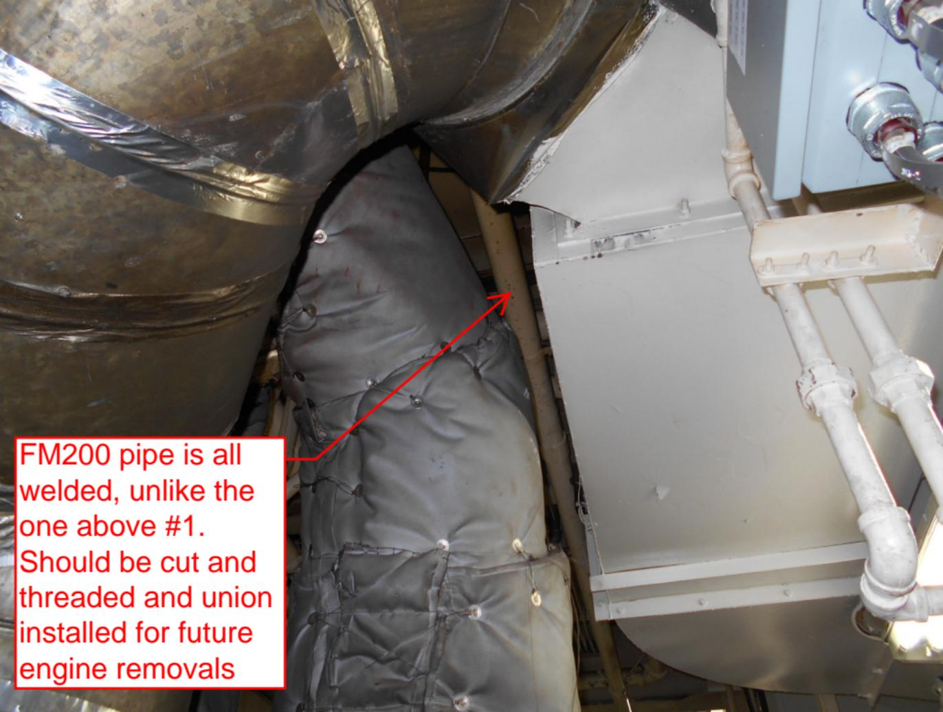
FM200 pipe is all welded, unlike the one above #1. Should be cut and threaded and union installed for future engine removals
