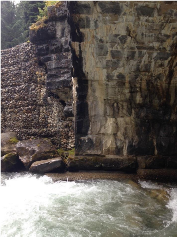
Left inlet: Stake gone. Water @ foundation level.
