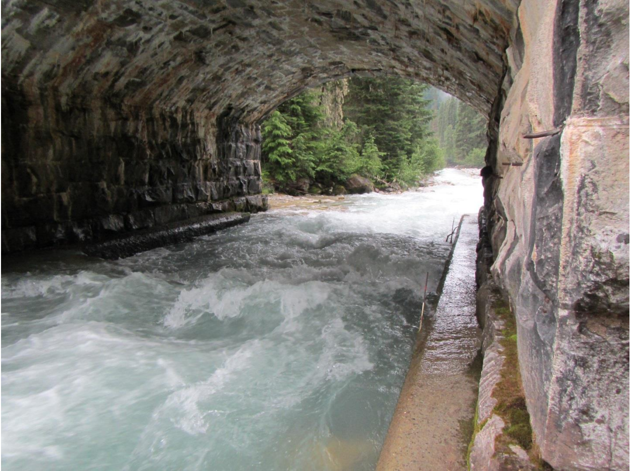
Figure 2: Right inlet August 2, 2016
