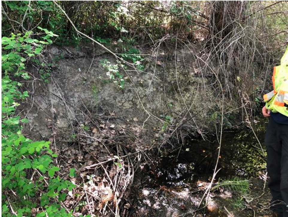
Photo 35: Eroded bank along south side of Reach 3 tributary channel, looking southwest.
