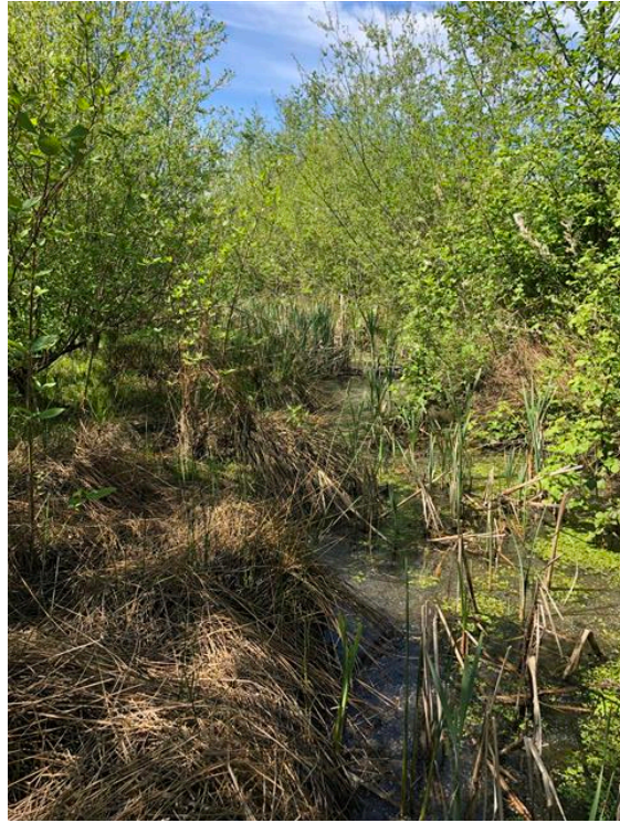
Photo 25: Reach 1B typical channel condition, looking west.
