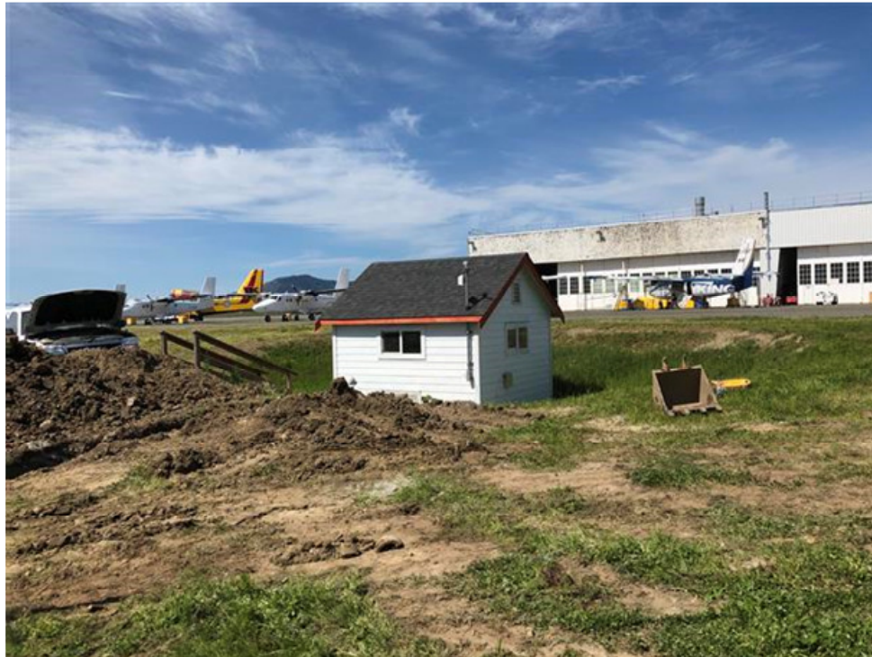
Photo 17: Pumphouse along north side of Reach 1A at upstream end, looking northwest.
