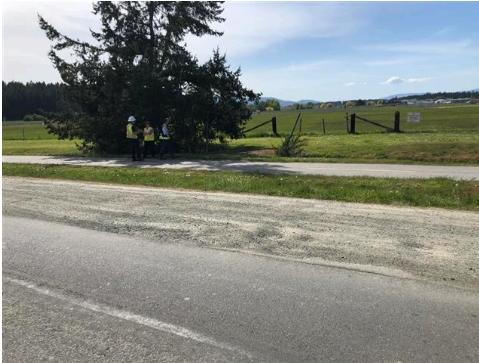
Photo 7: Access to potential alternate stockpile or laydown area, looking west. Cycling / Pedestrian path visible between Canora Road (foreground) and field. Access gate visible in background.
