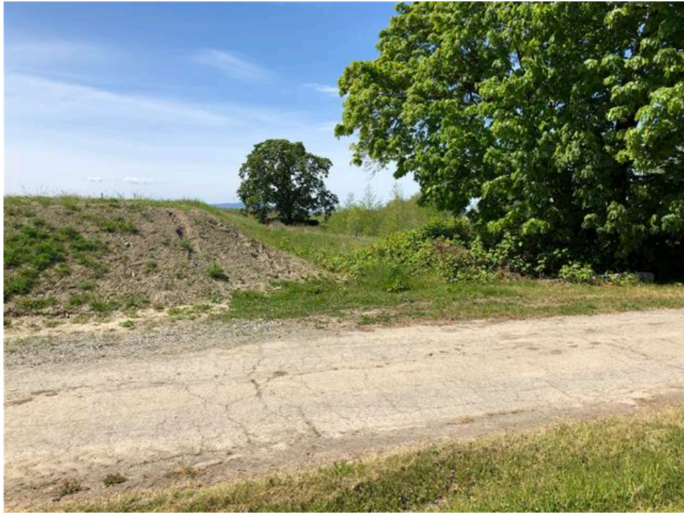
Photo 29: Potential access to Reach 1B, looking northwest. Relocation of end of berm on left may be required for significant tree protection.
