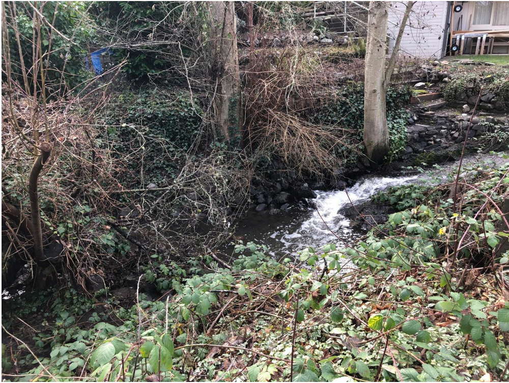
Photo 13: Spillway to the southwest of Reay Creek Pond Dam, looking west.
