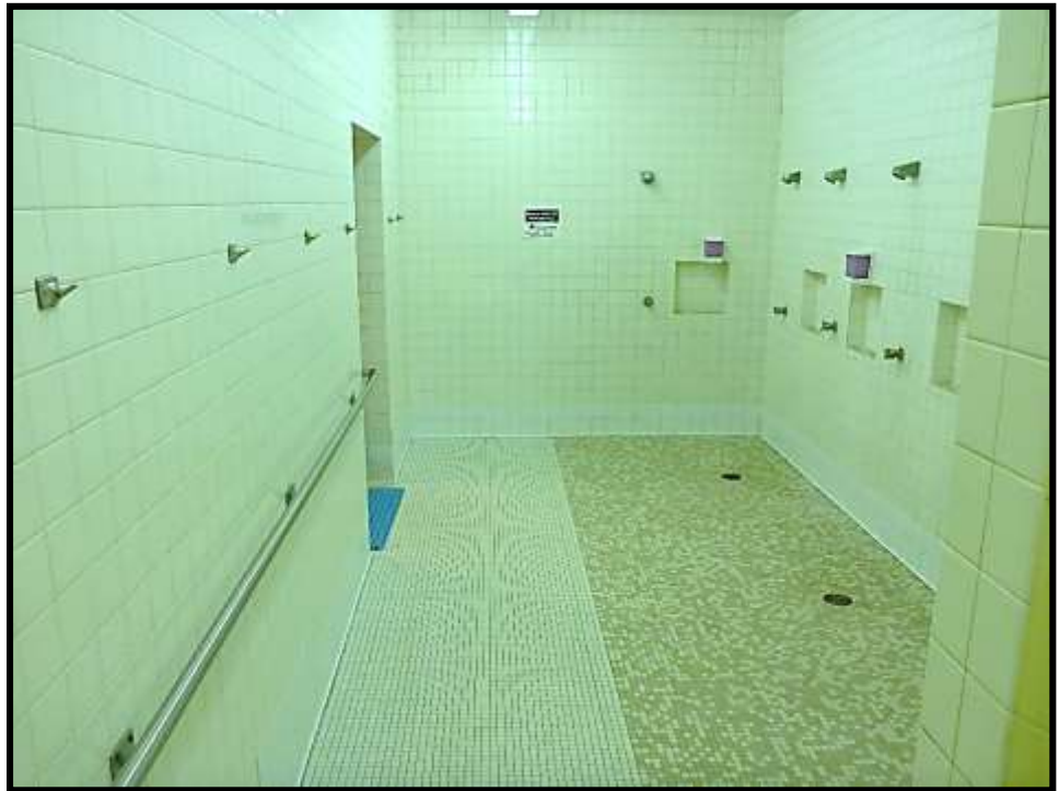
Photograph #2 – Asbestos-Containing Tile Thin Set Mortar under Brown & Beige Tiles – Room 100 107 (Reference Sample A8b)
