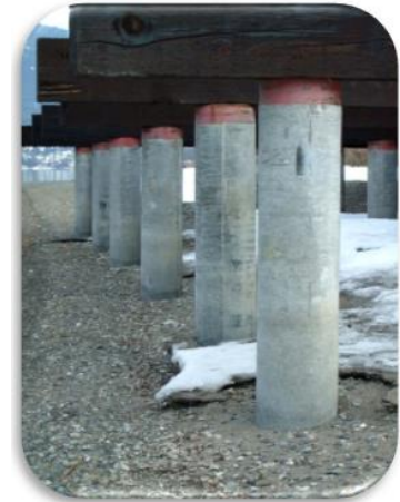
(Burton Marine Pile Driving Inc. 2017)
