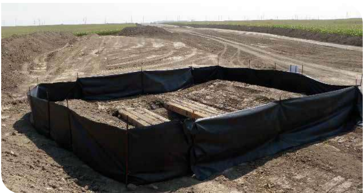
Cleaning station at construction site.
