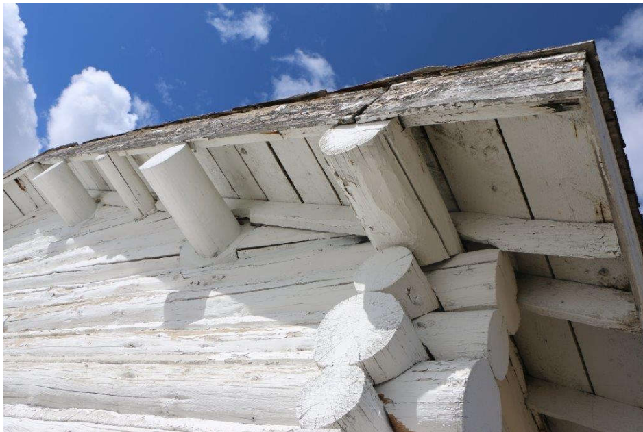
Stable – Exterior Elevations & soffit/fascia closeup at gable end. (March 2019)
