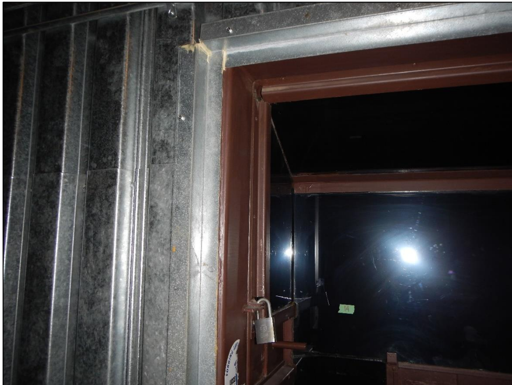
Photograph #6: Lead-based grey wall paint – Main catwalk (east and west)
