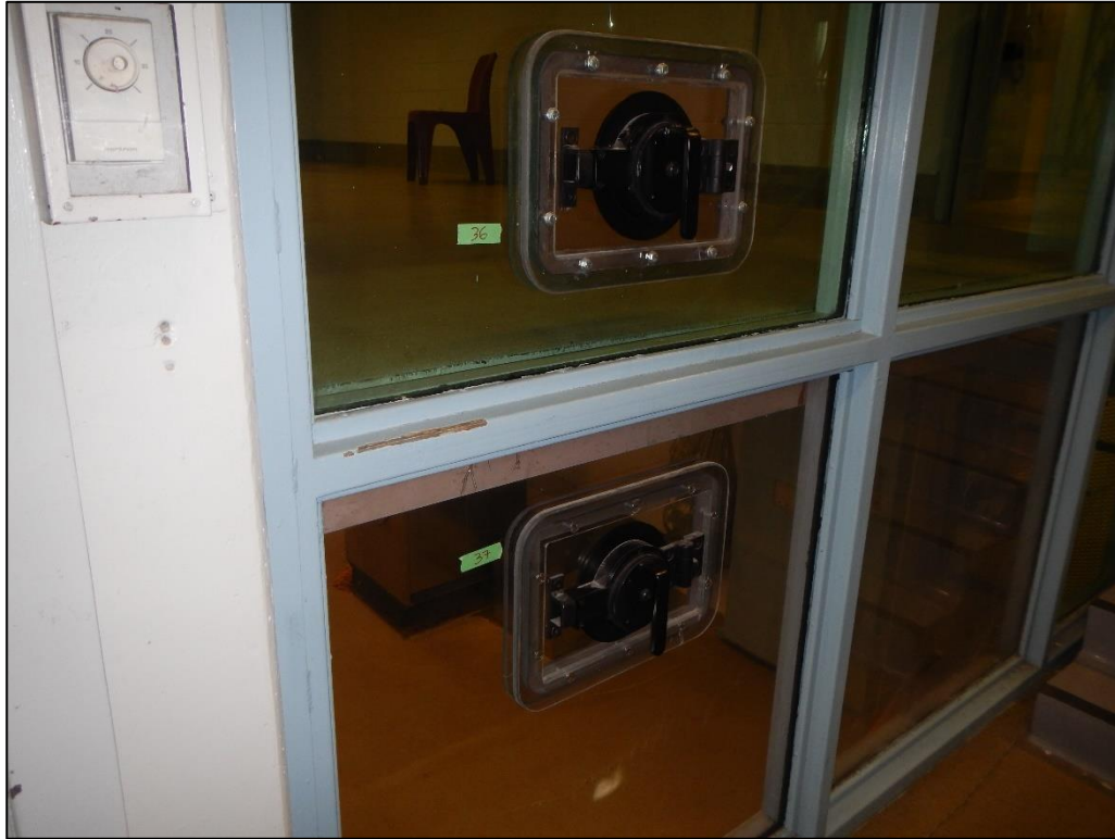
Photograph #7: Lead-based light blue trim/door paint – Corridors 102 & 104
