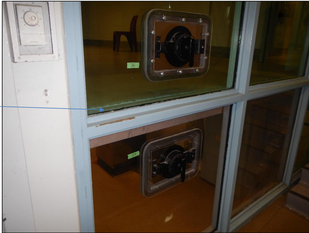
Photograph #5: Asbestos-containing black window pane mastic (b/t pane and frame) – D-Block guard unit/office and Corridors 102 & 104
