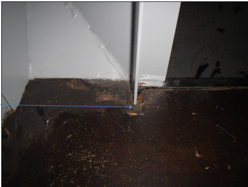
Photograph #2: Asbestos-containing brown window frame mastic (b/t frame and ledge) – Main Catwalk (East & West)
