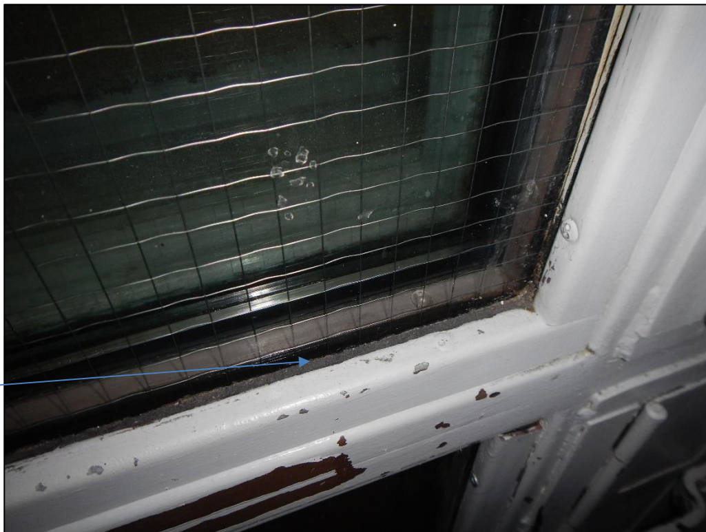
Photograph #4: Asbestos-containing black window pane mastic (b/t pane and frame) – D-Block guard unit/office and Corridors 102 & 104
