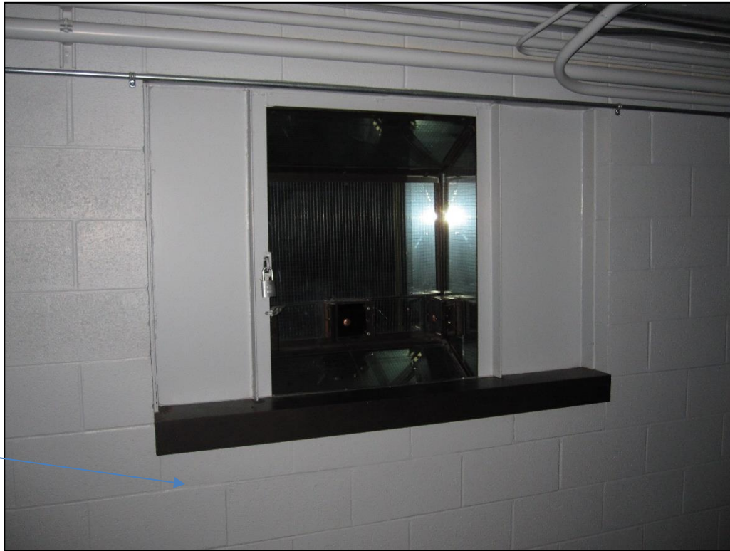
Photograph #1: Asbestos-containing vermiculite block wall insulation in block walls – Main Catwalk (East)
