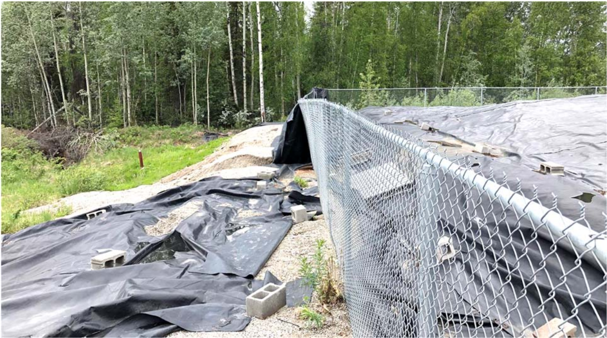
Photo 3: View of Iron Creek southern berm repair area, looking west.
