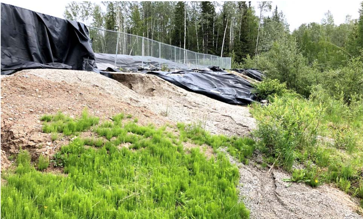
Photo 6: View of Iron Creek southern berm repair area facing east.
