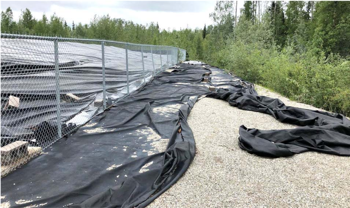
Photo 1: View of Iron Creek western berm disturbed cover, facing south.
