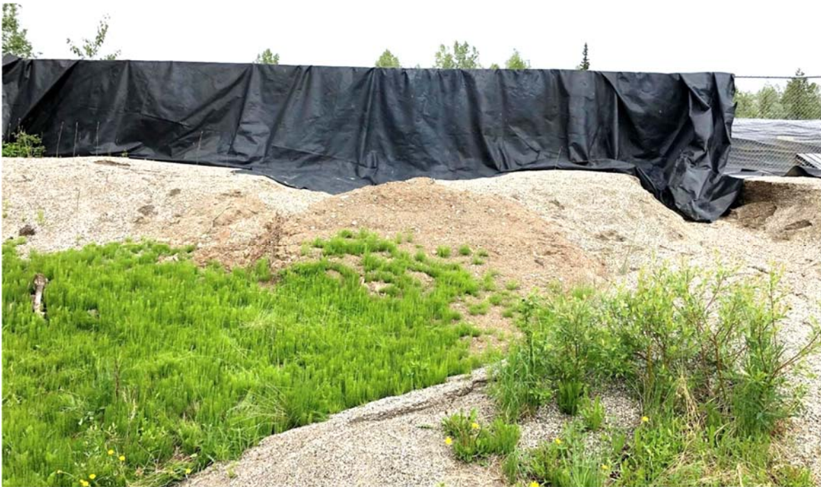
Photo 5: View of Iron Creek southern berm repair area, facing north.
