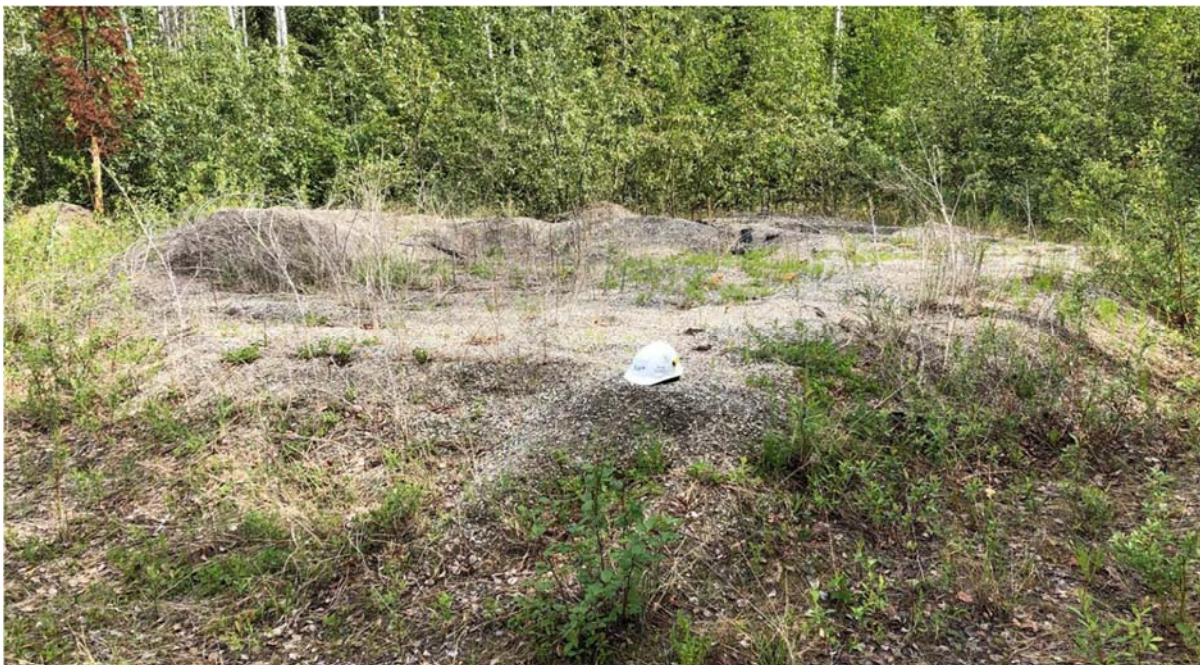
Photo 8: View of Owner supplied berm repair material, if required, located northeast of the Iron Creek STF.
