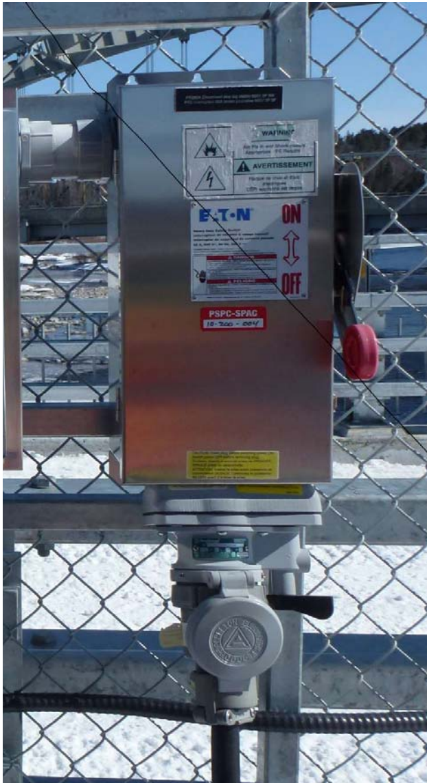
Figure 8 - Electrical outlet for stoplog lifter
