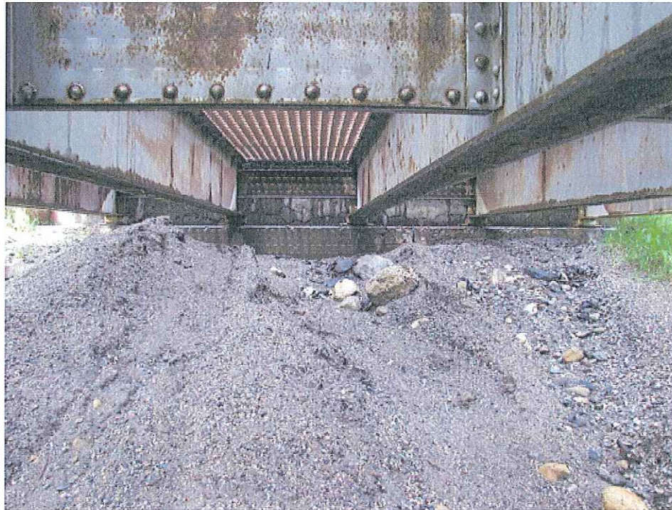
Photo 11 – South Abutment and Approach Span
