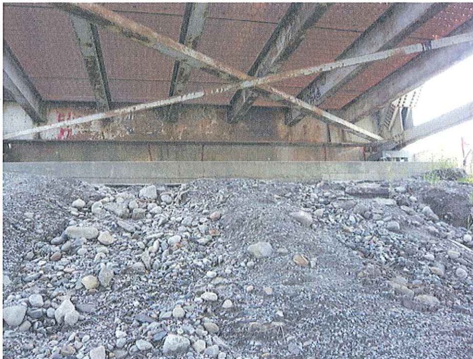
Photo 12 – South Abutment and Embankment
