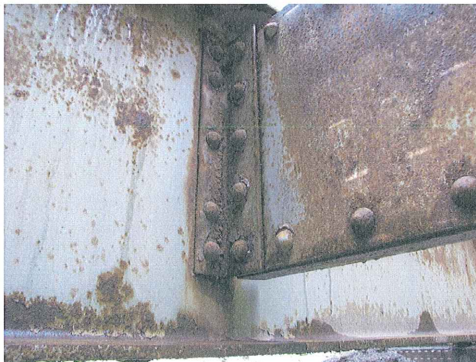
Photo 12 – Connection of Diaphragm at Girder Web
