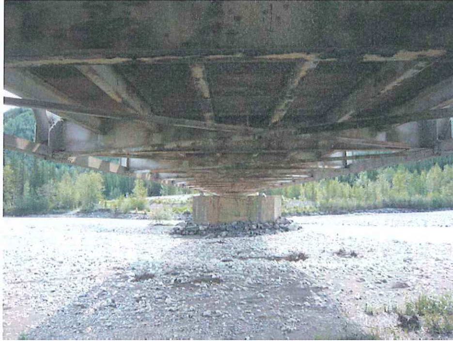
Photo 9 – Floor Beams, Stringers and Pier
