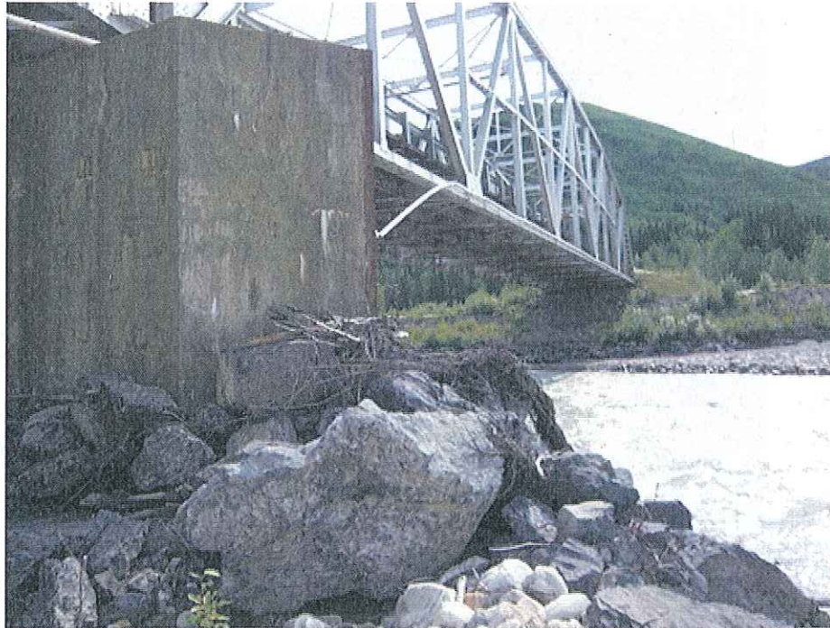
Photo 11 – Riprap Protecting Pier in River
