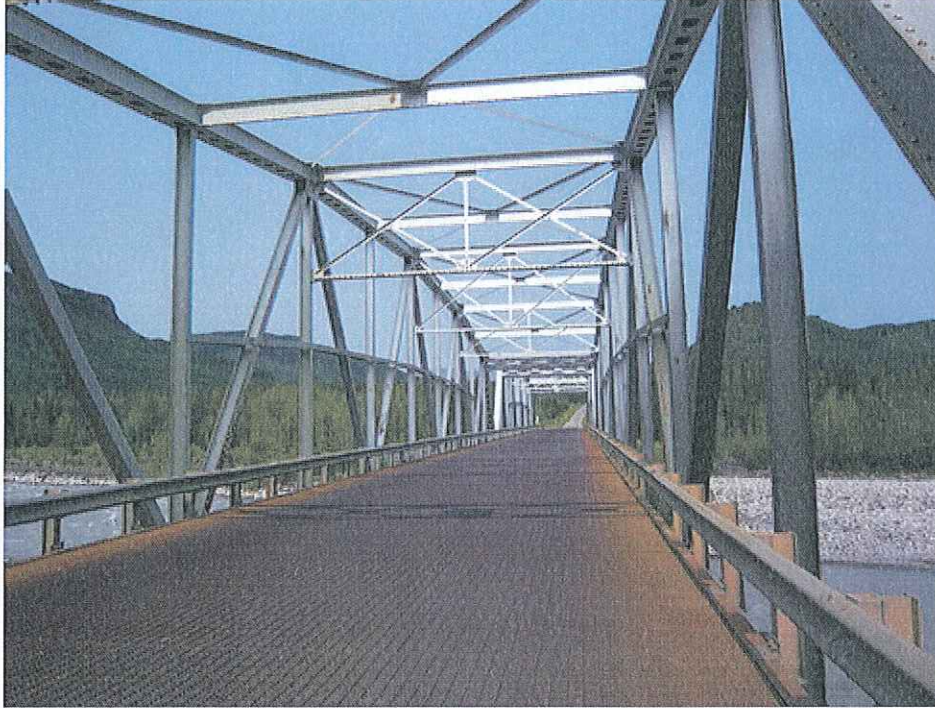
Photo 3 – Steel Grating Deck and Trusses
