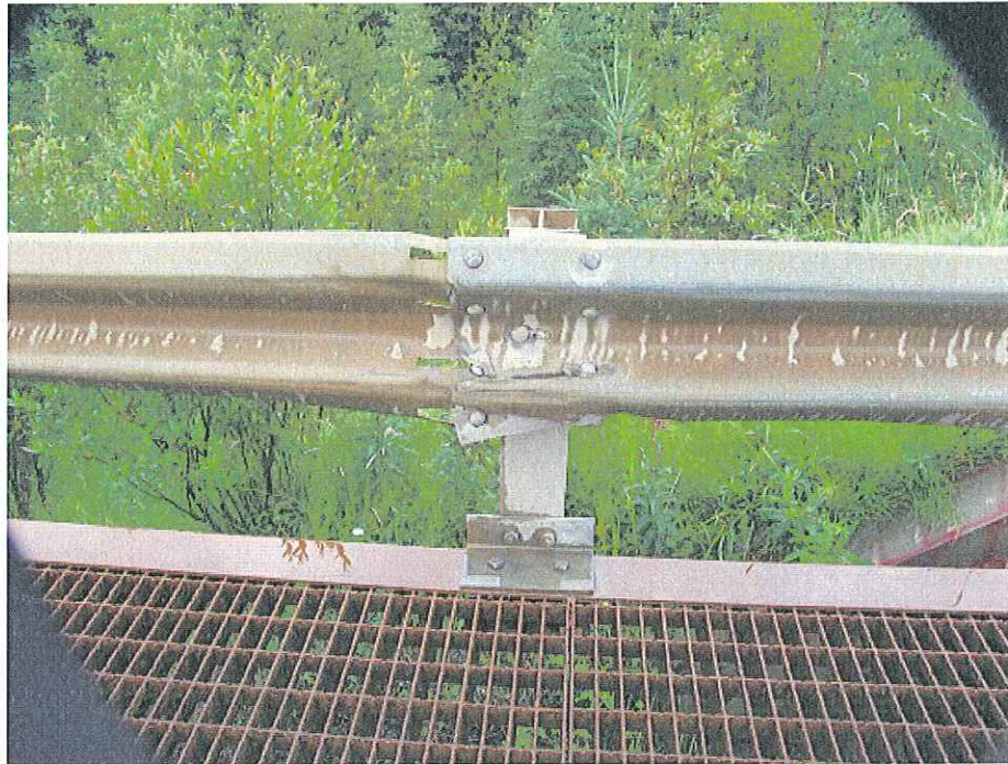
Photo 3 – Felxbeam - Bridge Barriers
