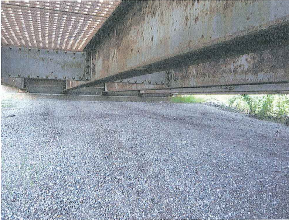
Photo 7 – North Abutment and Approach Girders
