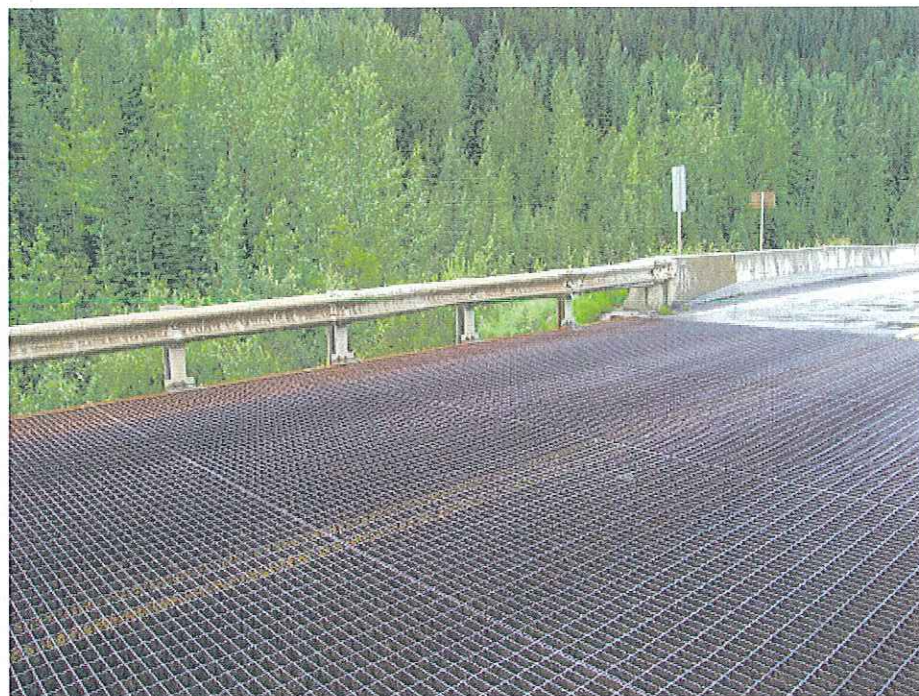
Photo 4 – Open Steel Grating Deck
