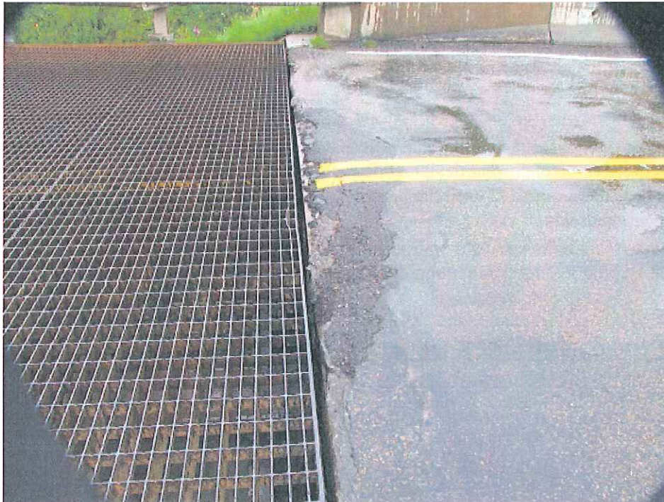
Photo 2 – South Deck Joint
