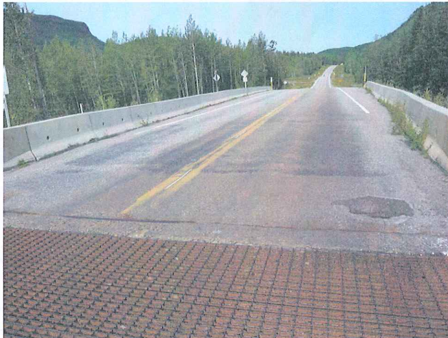
Photo 6 – North Approach and North Deck Joint
