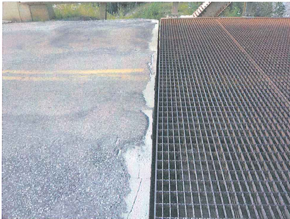
Photo 2 – South Deck Joint
