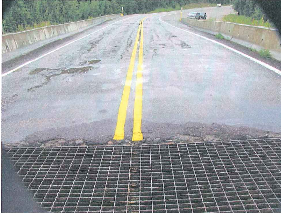
Photo 1 – South Approach and South Deck Joint
