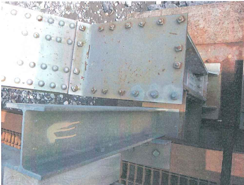
Photo 14 – Vertical Post – Missing Bolts Installed on Top Plate
