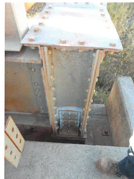
PIER 2 WEST VERTICAL END POST
