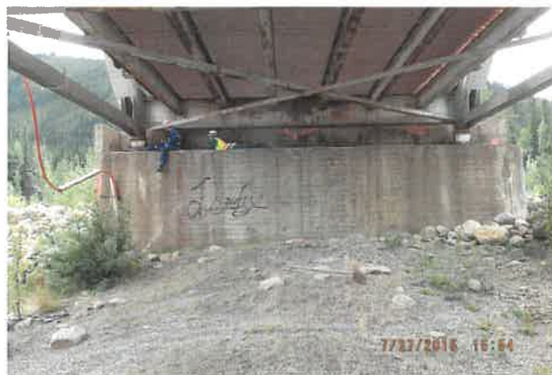
SOUTH FACE OF PIER 4
