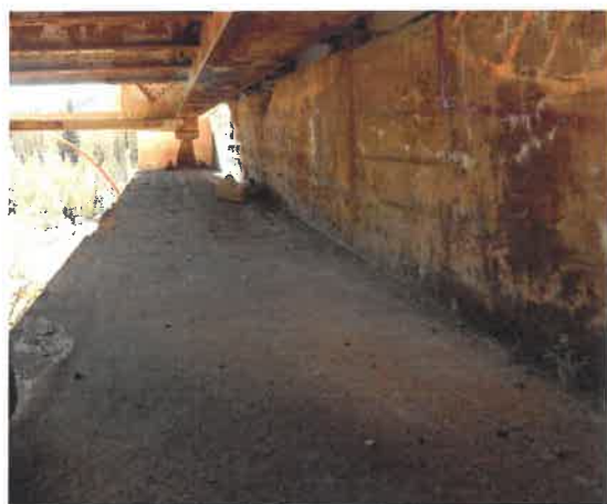
PIER 4 BEARING SEAT
