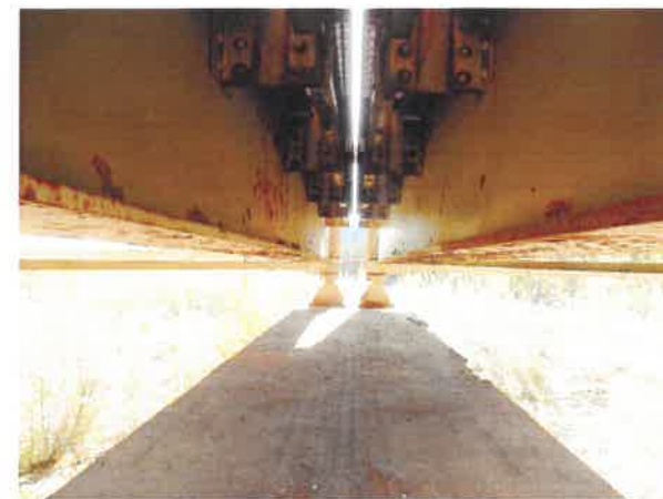
PIER 3 BEARING SEAT
