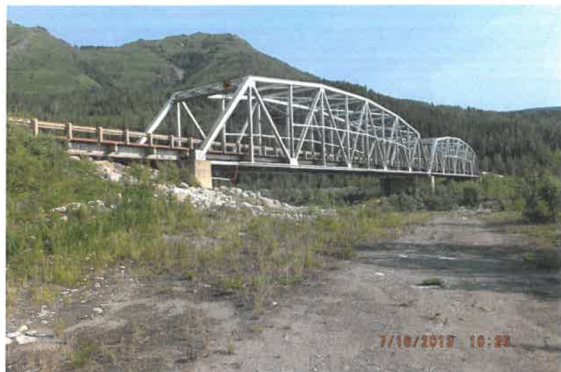
EAST ELEVATION OF STRUCTURE
