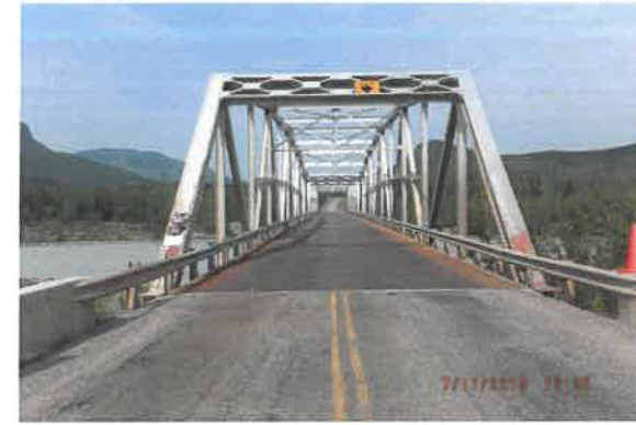
EAST END OF STRUCTURE
