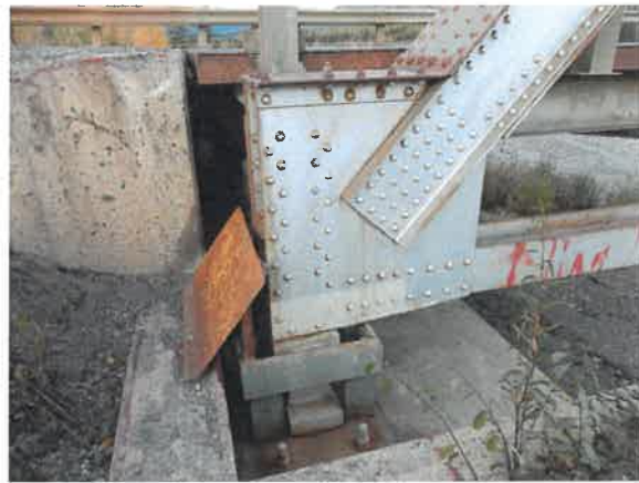
PIER 2 NORTH BEARING LOCATION - 225 ft SPAN
