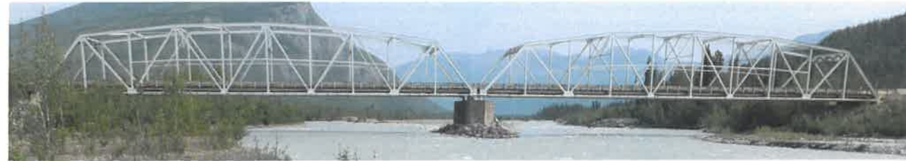
WEST ELEVATION OF STRUCTURE
