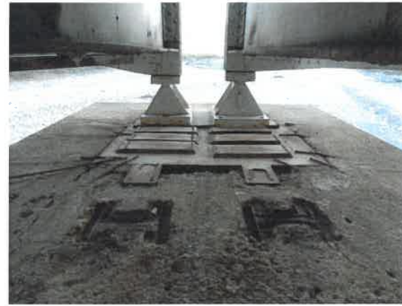
PIER 3 BEARING SEAT-EXISTING STEEL COMPONENTS EMBEDDED IN BEARING SEAT
