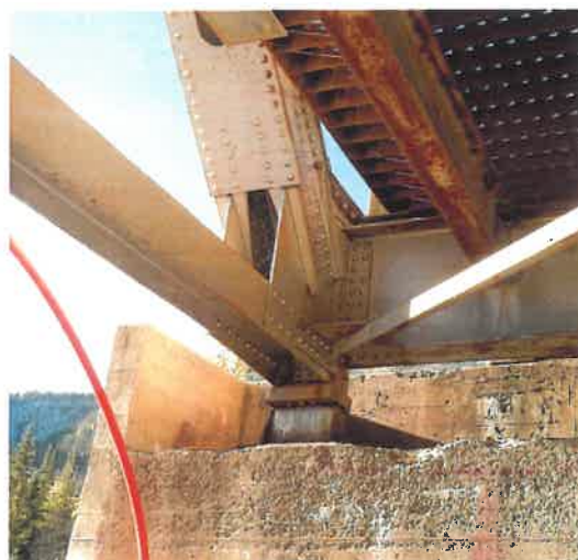
TYPICAL TRUSS END CONNECTION AT BEARING
