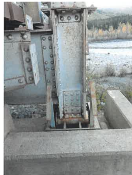
PIER 4 SOUTH VERTICAL END POST - 200 ft SPAN
