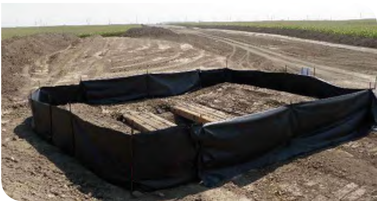
Cleaning station at construction site.
