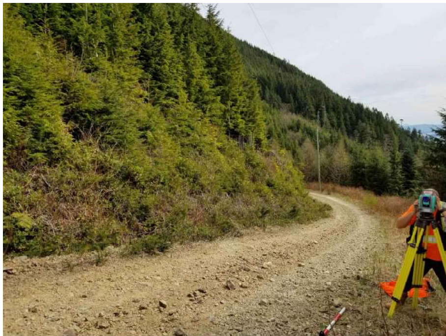
Facing Down Ozzard Road at Design CL
