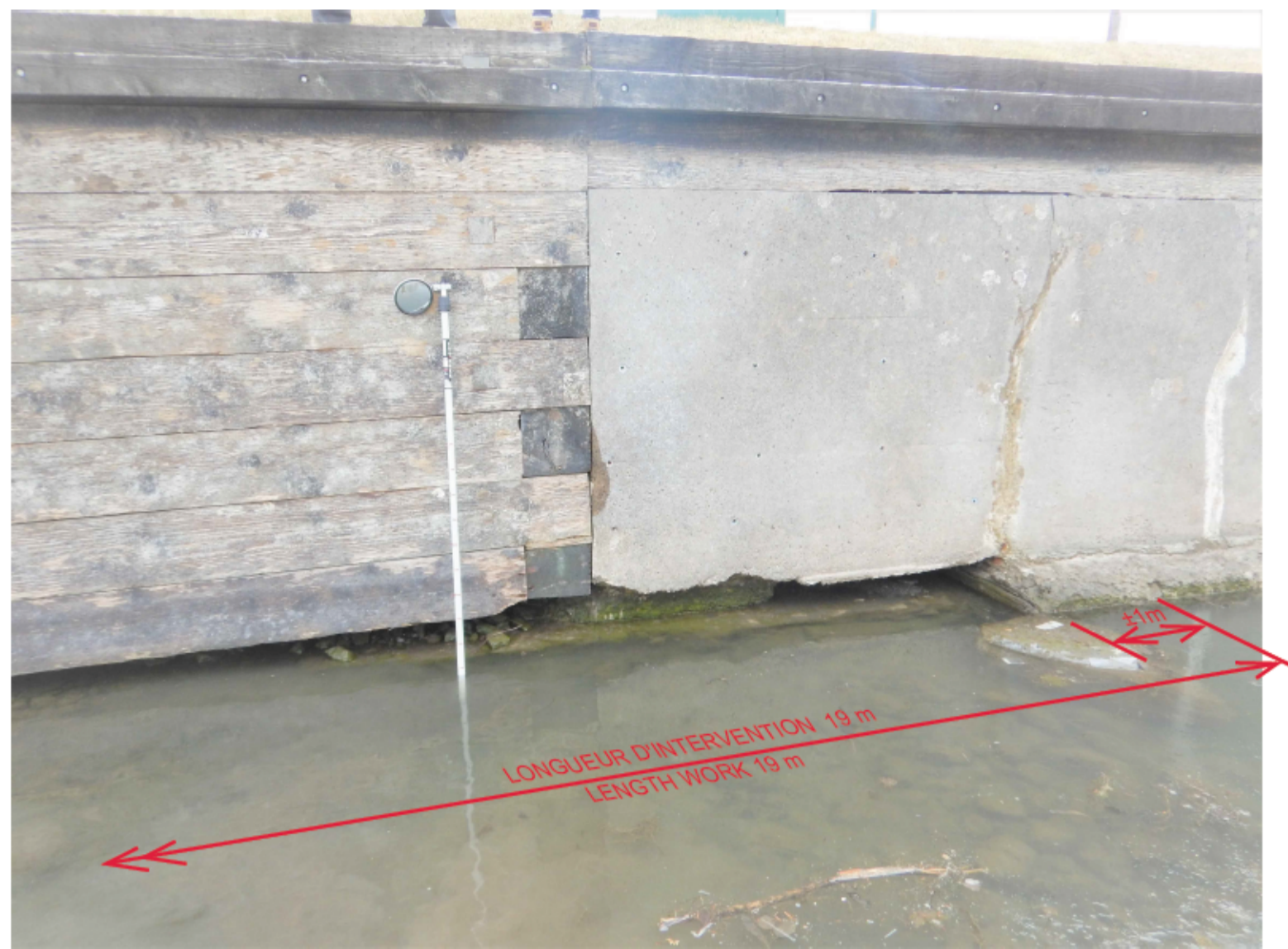
PHOTO 09-7841 MUR DROIT - AVAL PICTURE 09-7841 RIGHT WALL - DOWNSTREAM
