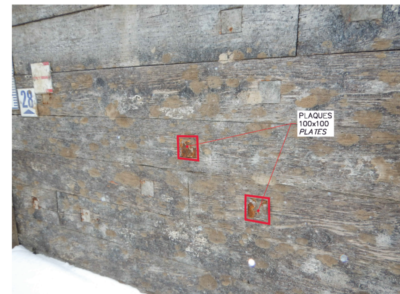
PHOTO 11-7208 MUR DROIT - AMONT PICTURE RIGHT WALL - UPSTREAM
