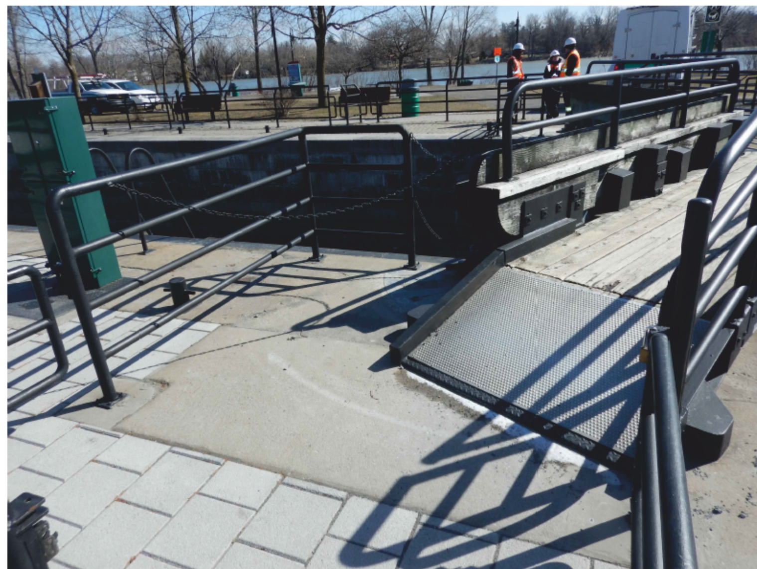
PHOTO 28-7726 PASSERELLE EN SERVICE PICTURE 28-7726 FOOTBRIDGE IN OPERATION
