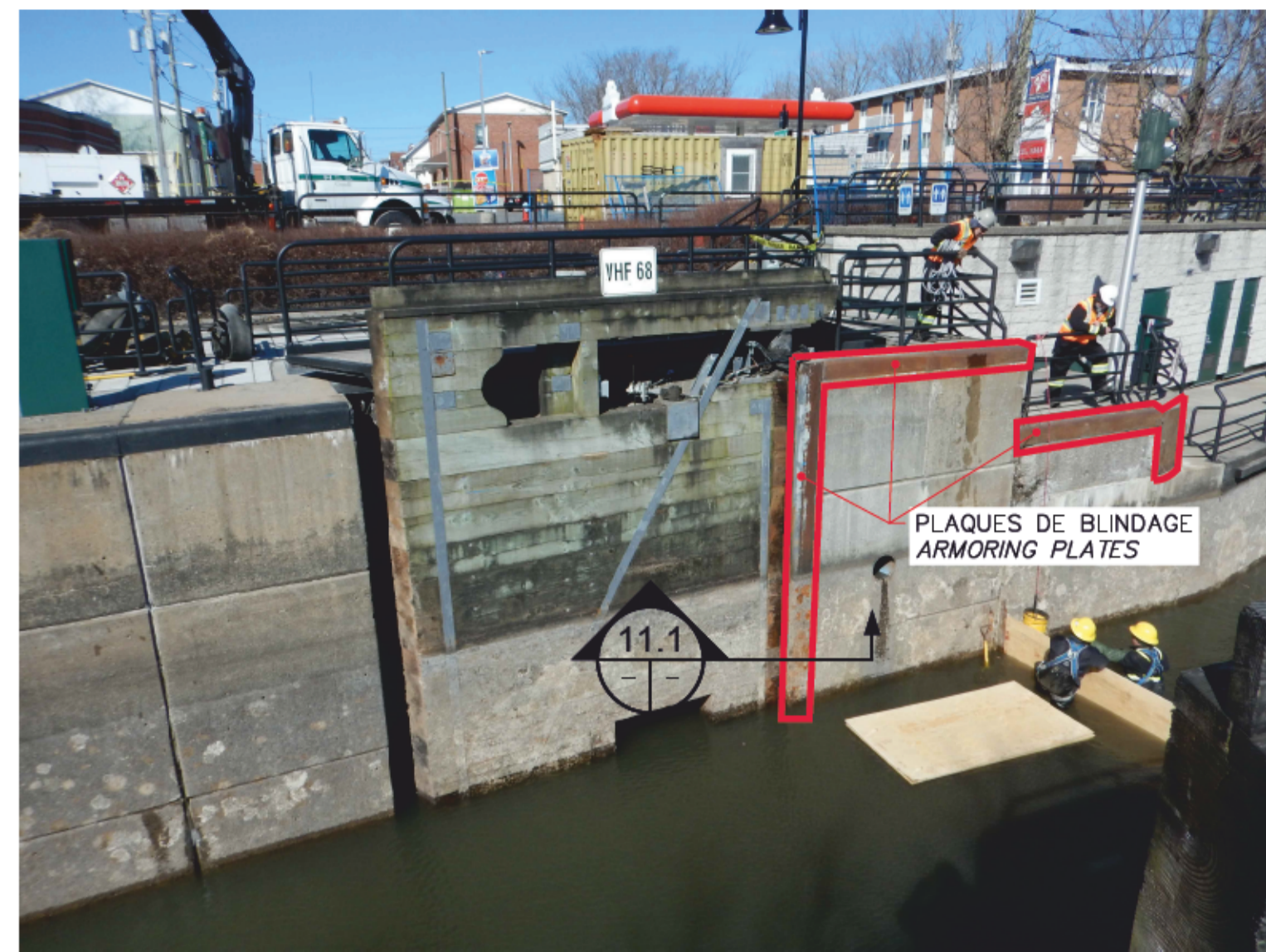
PHOTO 11-7722 MUR GAUCHE - AVAL PICTURE LEFT WALL - DOWNSTREAM
