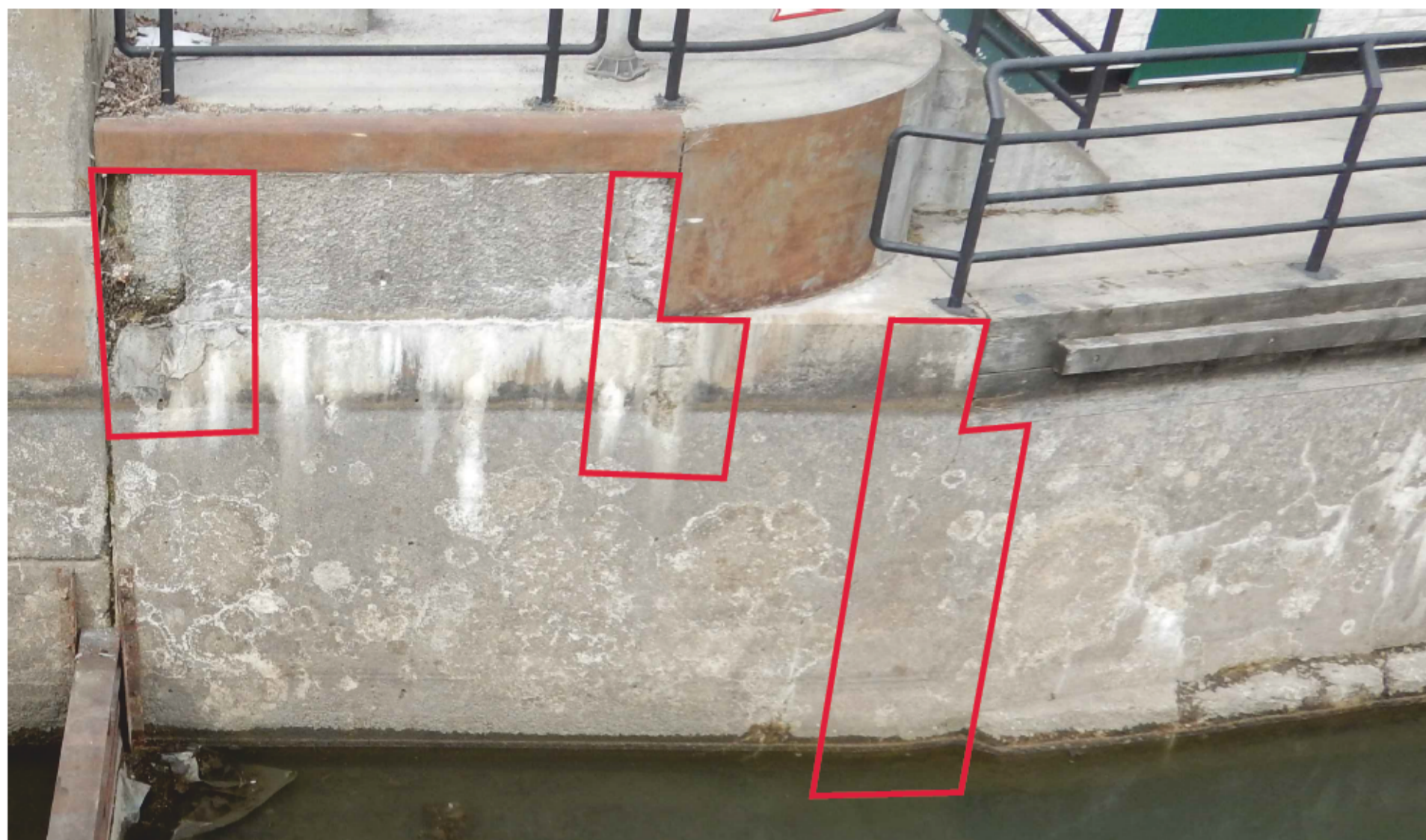
PHOTO 13-7874 MUR GAUCHE - AVAL PICTURE LEFT WALL - DOWNSTREAM
