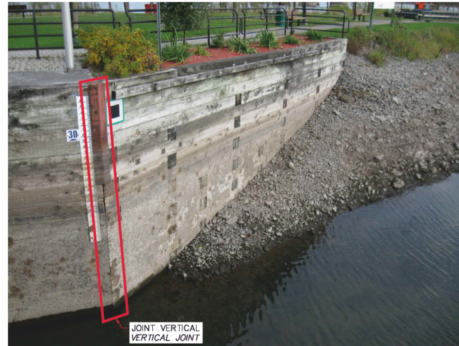
PHOTO 07-0492 MUR DROIT - AMONT PICTURE RIGHT WALL - UPSTREAM
