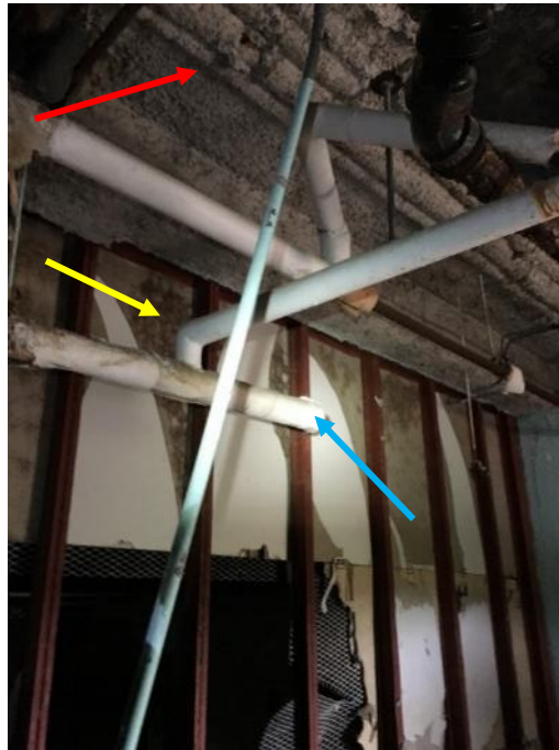
Photo 11: View of asbestos-containing fireproofing (red arrow, DST Sample 29911-3-02A), pipe fittings (blue arrow, DST Sample 29911-3-03A), and mould-impacted drywall (yellow arrow) on the main floor at Building 3.
