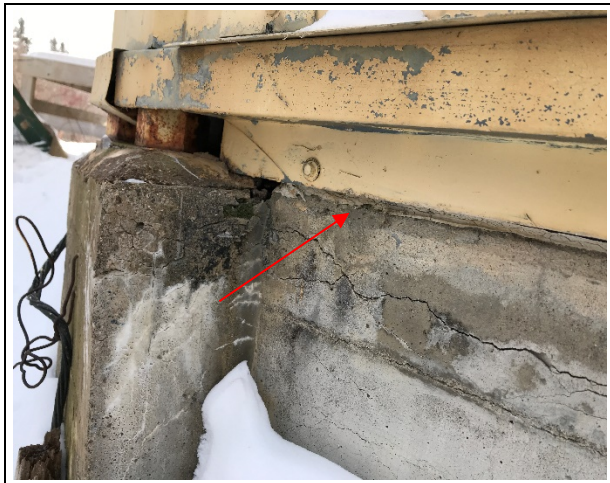
Photo 3: Building 1 – asbestos-containing (5% chrysotile) exterior caulking – grey
