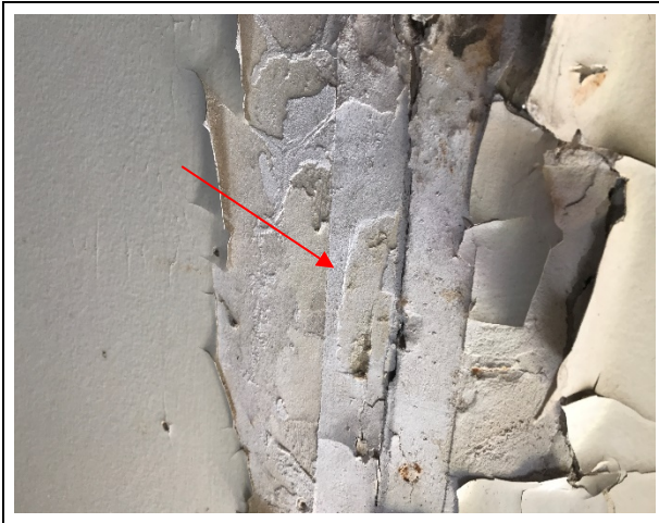
Photo 15: Building 2 – asbestos-containing (3% chrysotile) drywall joint-fill compound located in room 2
