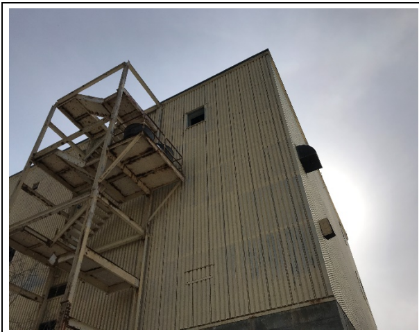
Photo 31: Building 3 – lead-containing (200 ppm) yellow/off-white coloured paint located on the exterior metal cladding
