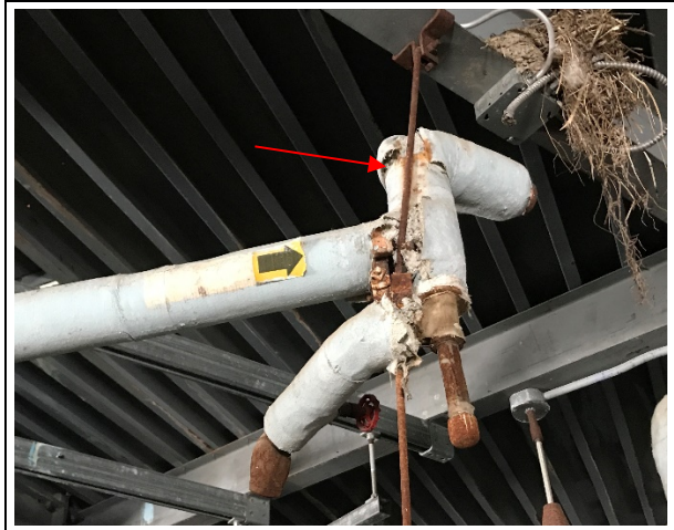
Photo 6: Building 1A – asbestos-containing (65% chrysotile) insulating cement on pipe fittings
