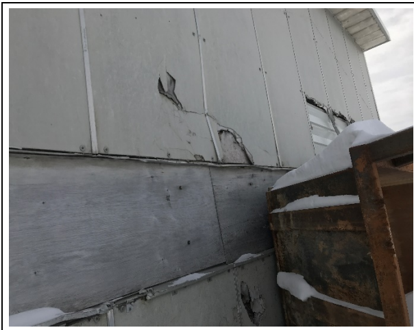
Photo 39: Building 4 – asbestos-containing (20% chrysotile) cement board panels located on the exterior of the building (north wall)
