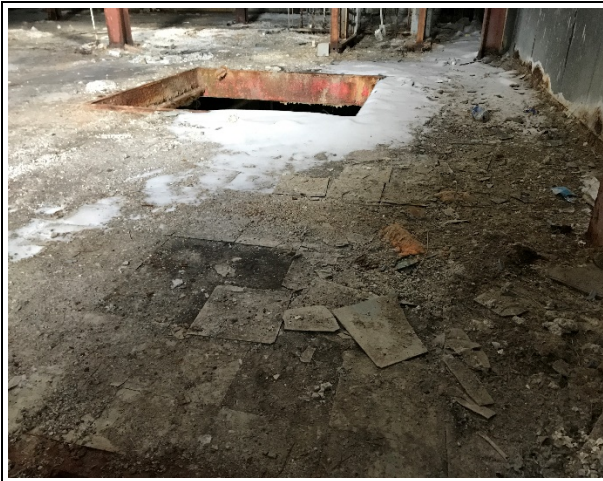
Photo 27: Building 3 – asbestos-containing (2% chrysotile) 9"x9" vinyl floor tile – grey located on the second floor
