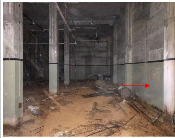
Photo 33: Building 3 – lead-containing (2,100 ppm) green coloured paint on the interior walls of the storage room
