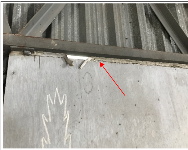
Photo 11: Building 1A – asbestos-containing (15% chrysotile) interior joint caulking – grey
