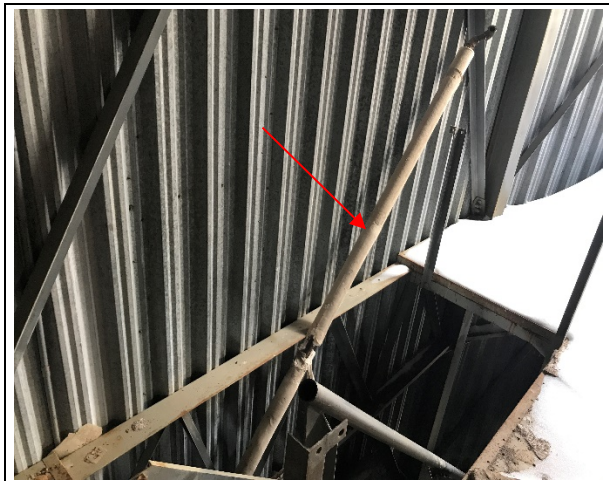
Photo 8: Building 1A – asbestos-containing (30% chrysotile) pre-formed pipe straight insulation
