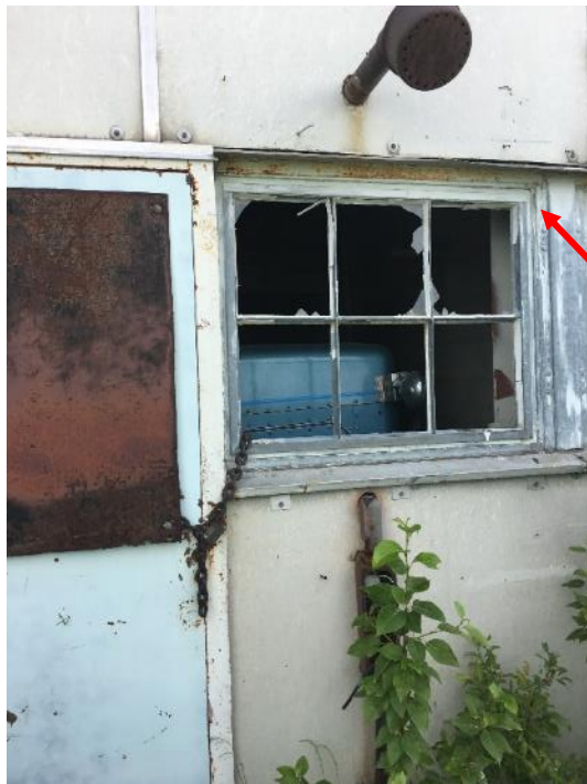
Photo 17: Asbestos-containing grey caulking (DST Sample 29911-4-05A) observed on the exterior windows throughout Building 4.
