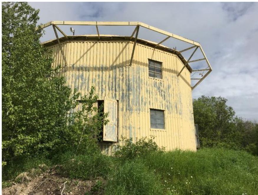
Photo 1 : Exterior view of Building 1 with yellow/grey paint on metal cladding (DST 2006, 353-01-LP-01). This paint was not identified as leachate hazardous with respect to lead.
