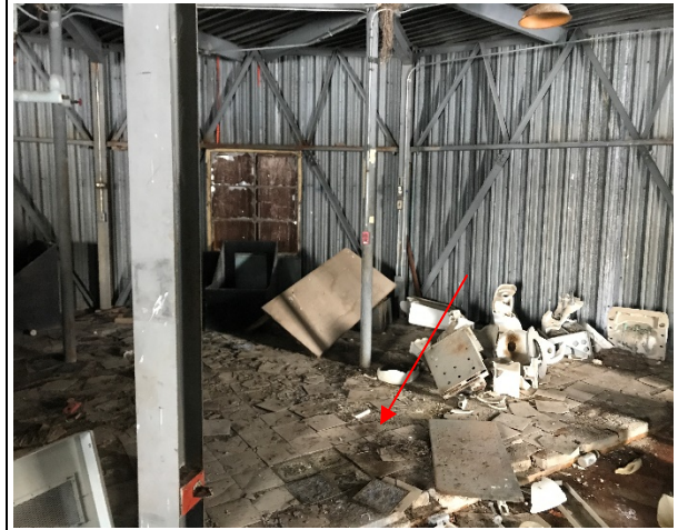
Photo 10: Building 1A – asbestos-containing (1% chrysotile) 9"x9" vinyl floor tile – grey
