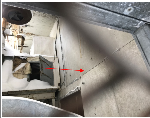
Photo 17: Building 2 – presumed asbestos-containing cement board panel located in room 1
