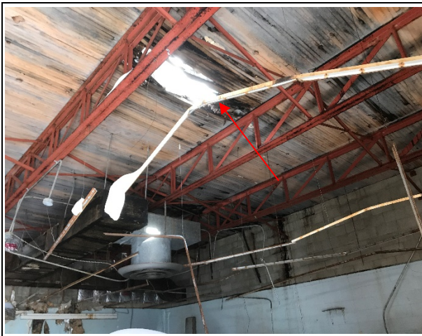
Photo 19: Building 2 – presumed asbestos containing roof insulation, roof caulking and roofing materials
