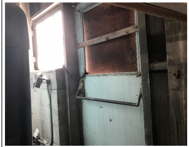
Photo 42: Building 4 – presumed asbestos-containing fire rated door located in bay 2 (west wall)
