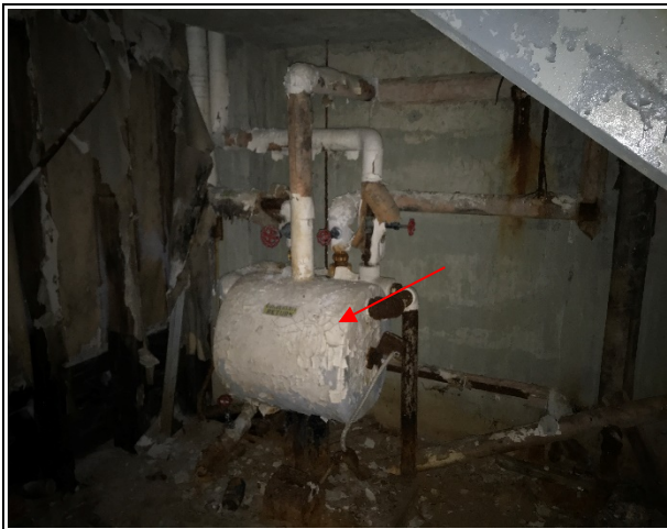
Photo 23: Building 3 – asbestos-containing (75% chrysotile) pre-formed tank/body insulation on the condensate return tank located in the storage room
