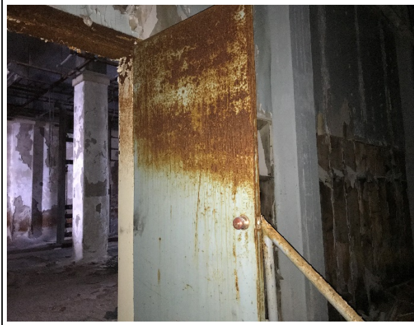
Photo 29: Building 3 – presumed asbestos-containing fire rated door located between communications and the storage room
