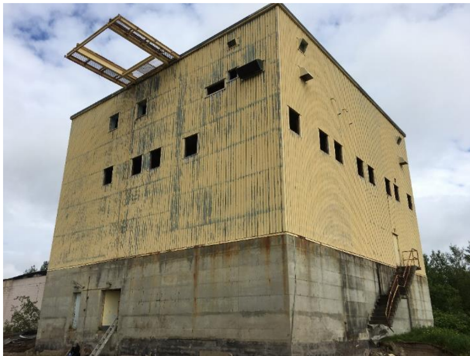
Photo 10: View of Building 3 with lead-containing yellow/Off-White paint on metal cladding (DST 2006, 353-3-LP-01). This paint has been identified as leachate hazardous with respect to lead.
