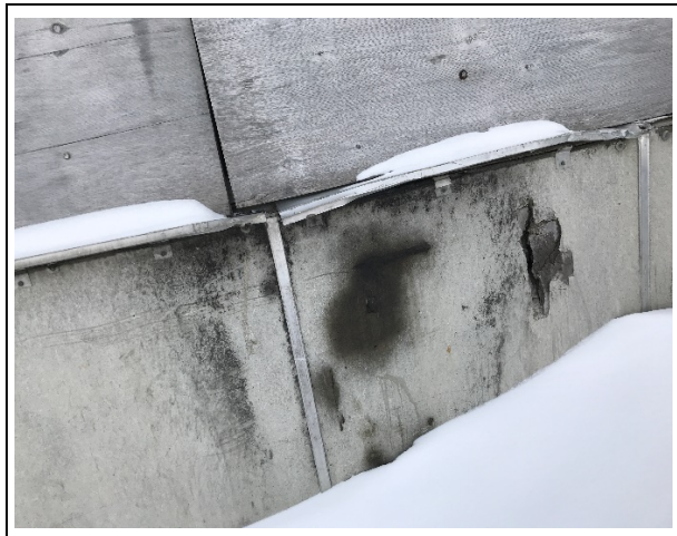
Photo 44: Building 4 – suspect mould located on the exterior north wall
