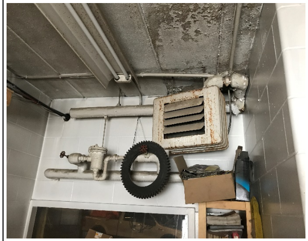
Photo 38: Building 4 – asbestos-containing (65% chrysotile) insulating cement on pipe fittings located in the storage room
