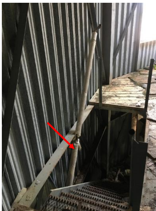
Photo 8: Asbestos-containing white pre-formed pipe insulation (Magblock) (DST Sample 29911-1A-04A), observed in stairwell of Building 1A.
