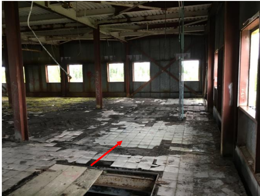
Photo 13: View of asbestos-containing blue 9"x9" vinyl floor tiles (DST Sample 29911-3-01A), observed throughout Building 3.
