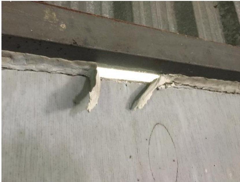
Photo 9: Asbestos-containing grey caulking (DST Sample 29911-1A-05A), noted between wood panels and the metal wall, on the 2 nd floor of Building 1A.
