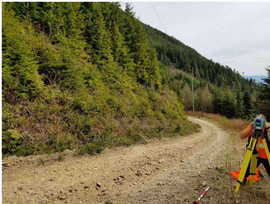
Facing Down Ozzard Road at Design CL
