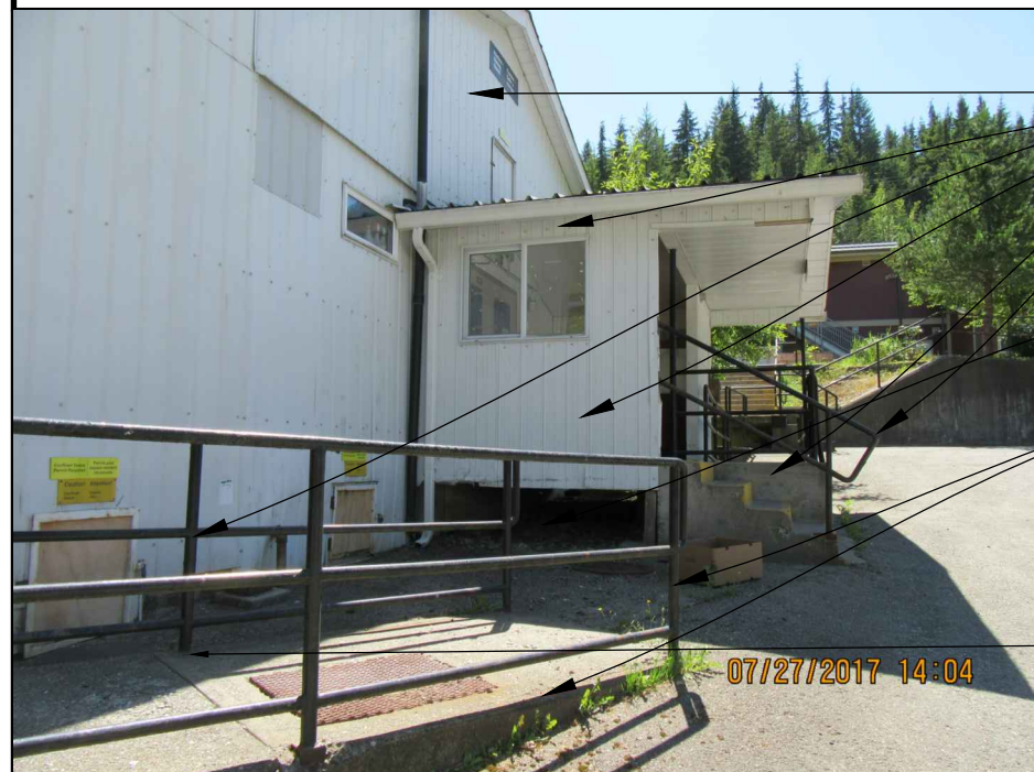
3 PHOTO OF EXISTING CONDITION
