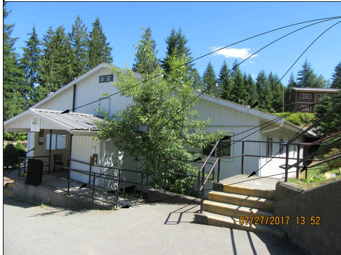
1 PHOTO OF EXISTING CONDITION
