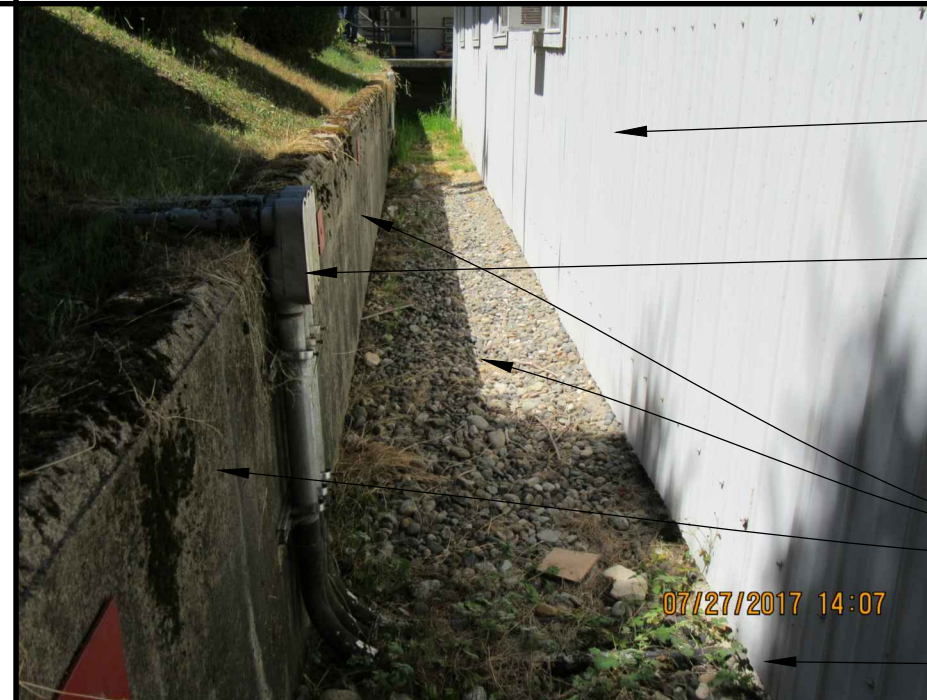
12 PHOTO OF EXISTING CONDITION
