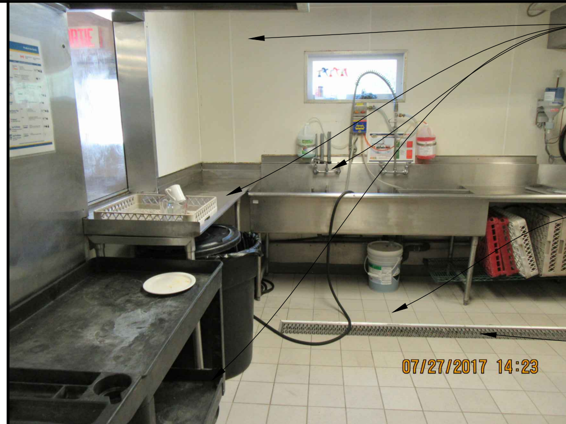
18 PHOTO OF EXISTING CONDITION
