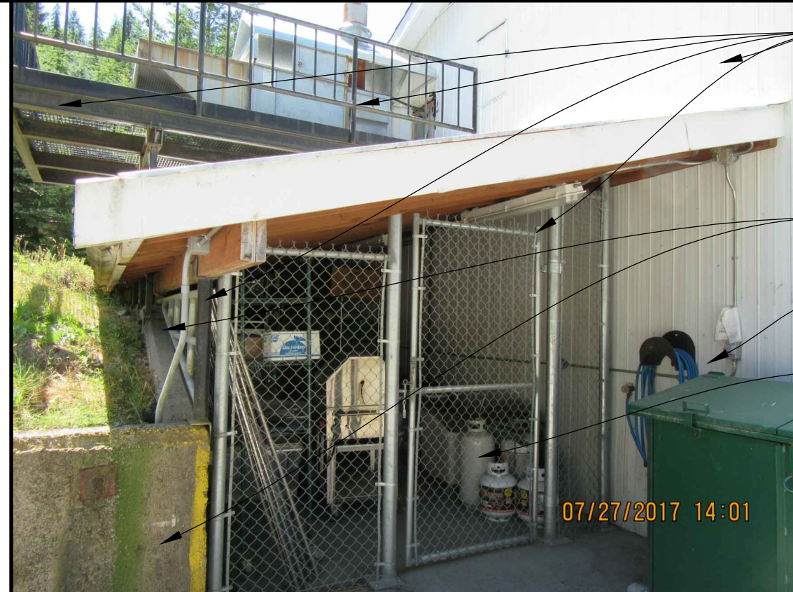
6 PHOTO OF EXISTING CONDITION
