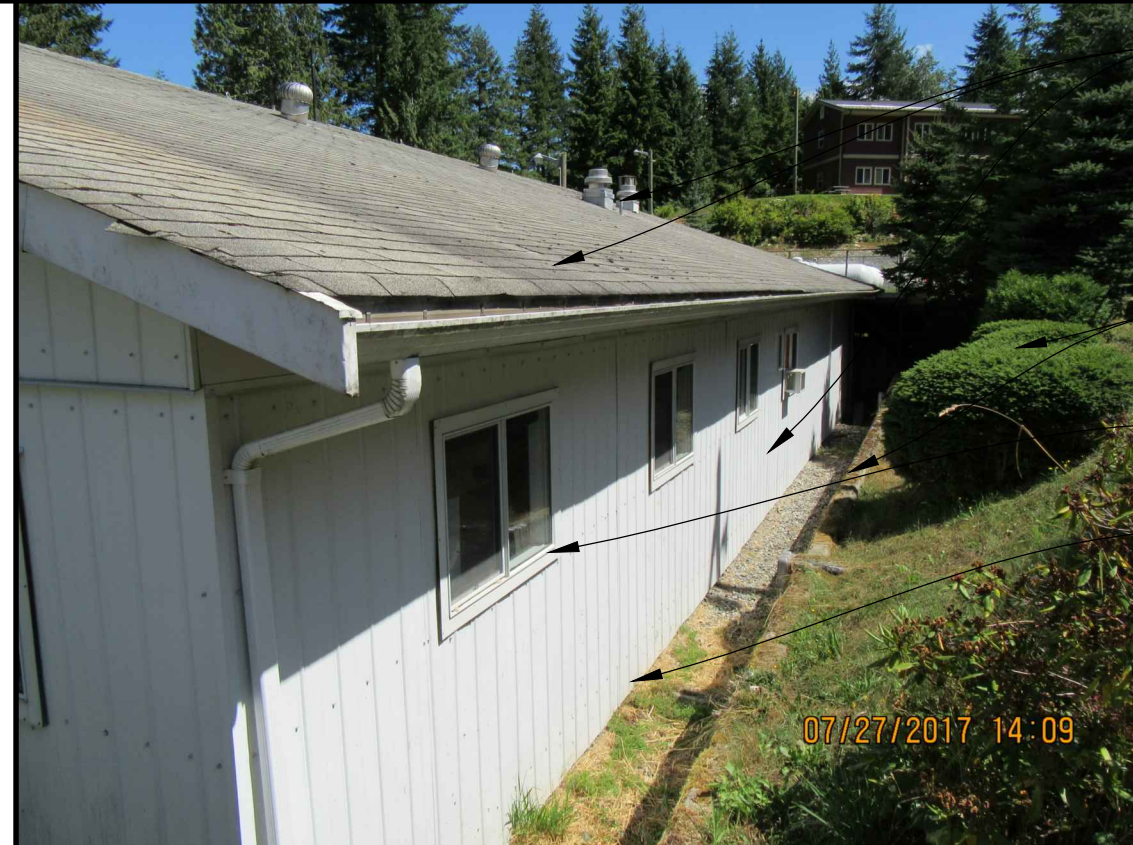
10 PHOTO OF EXISTING CONDITION
