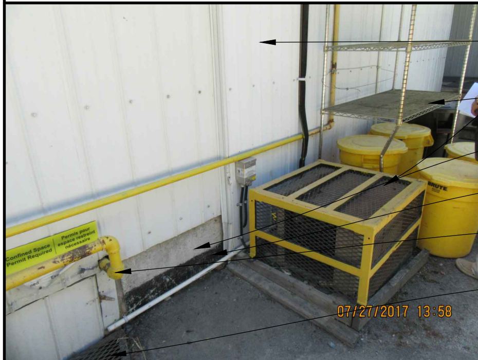
7 PHOTO OF EXISTING CONDITION
