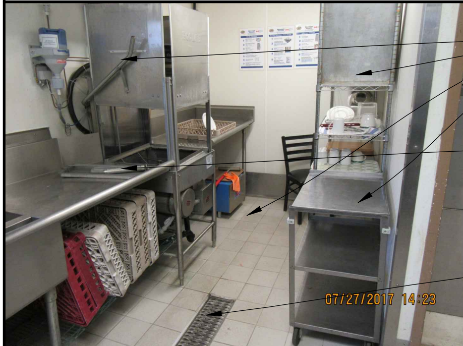
19 PHOTO OF EXISTING CONDITION
