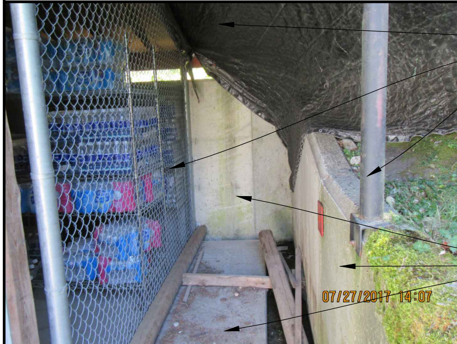
11 PHOTO OF EXISTING CONDITION
