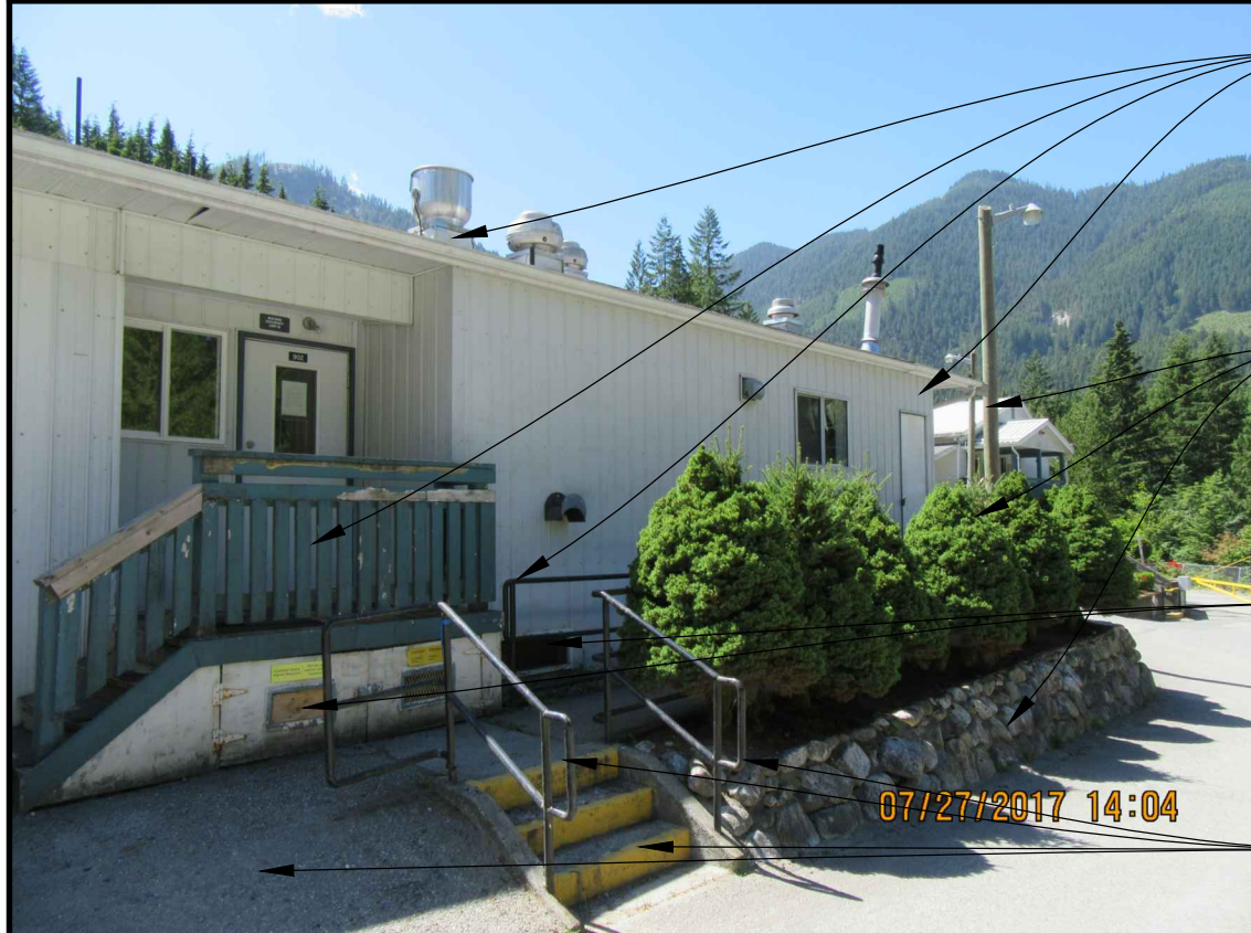
5 PHOTO OF EXISTING CONDITION
