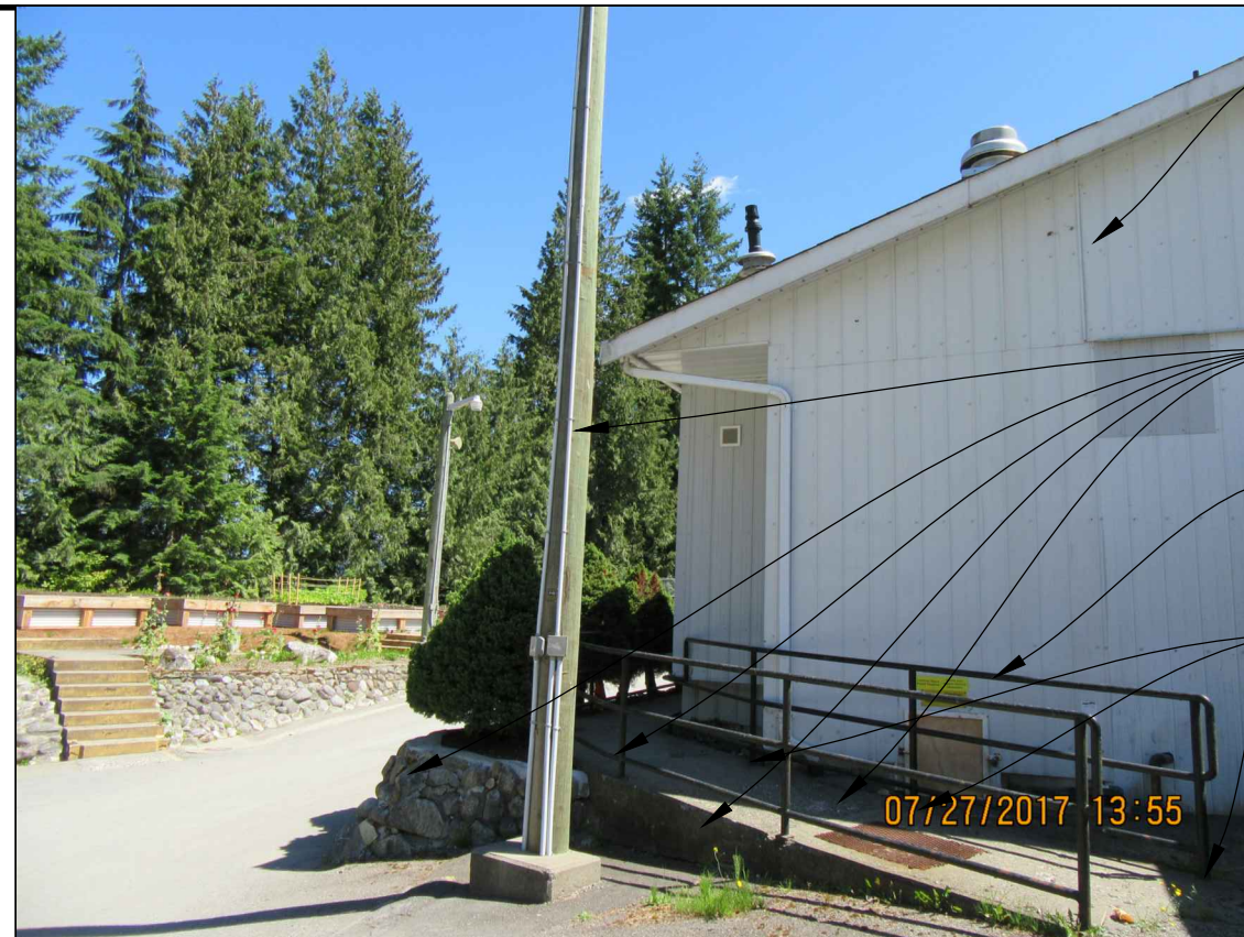
2 PHOTO OF EXISTING CONDITION
