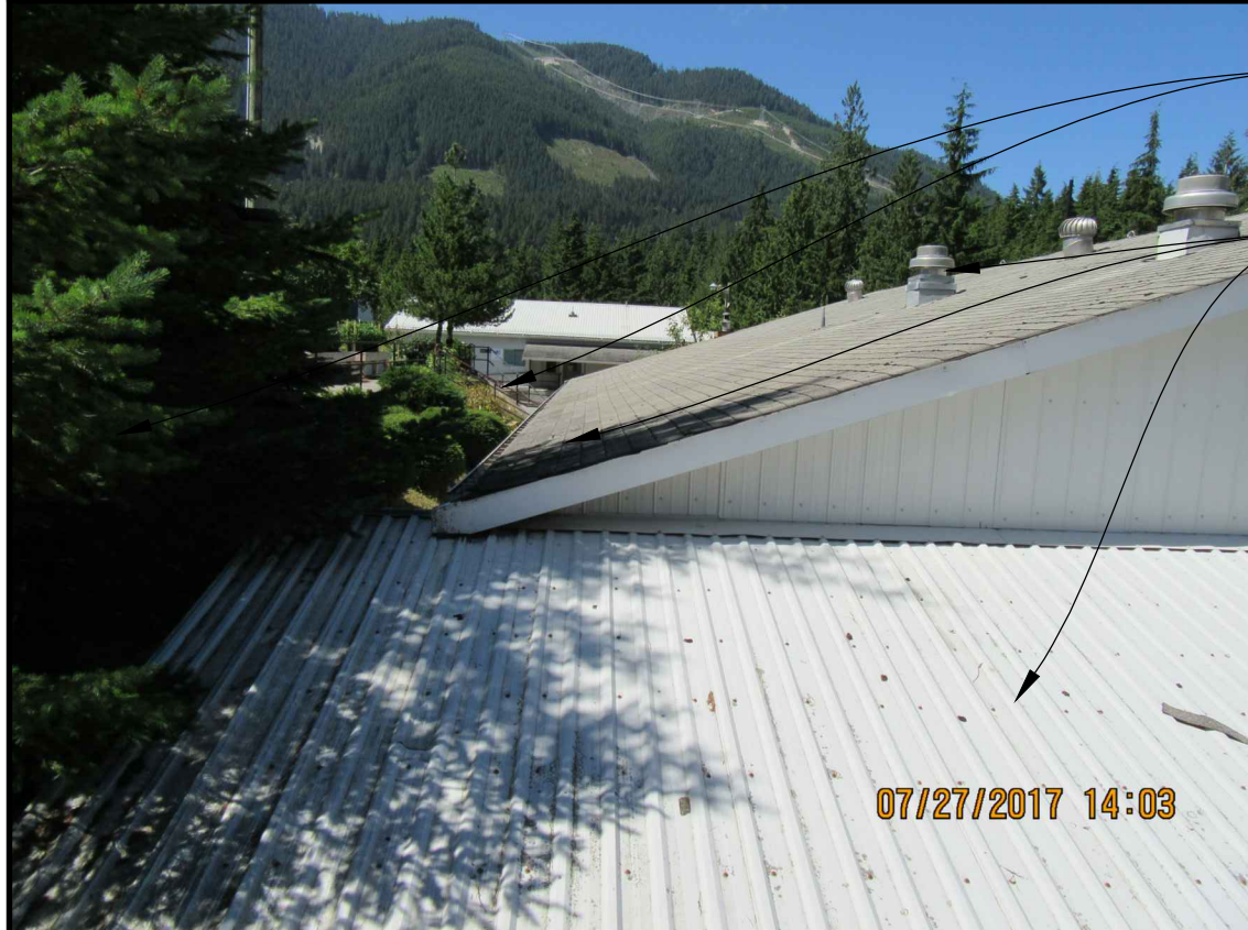
9 PHOTO OF EXISTING CONDITION
