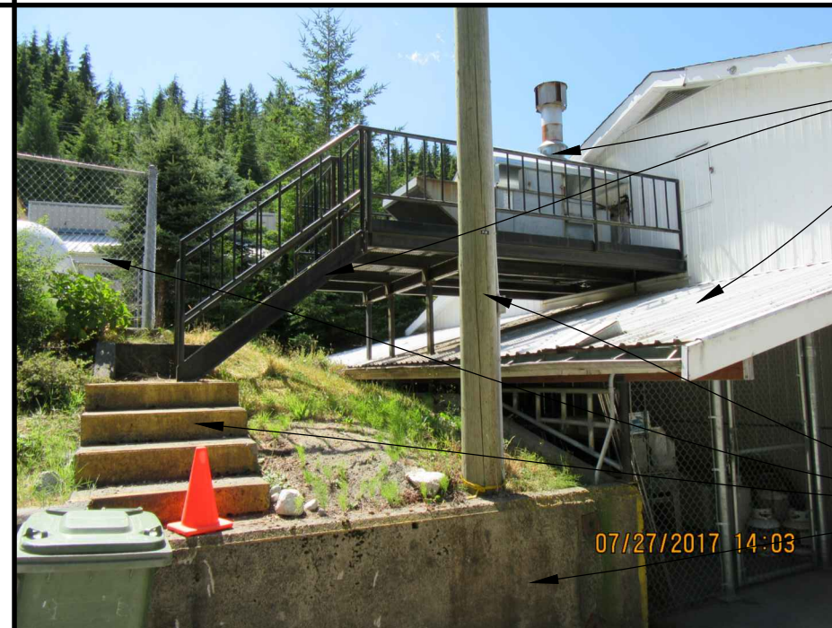
8 PHOTO OF EXISTING CONDITION
