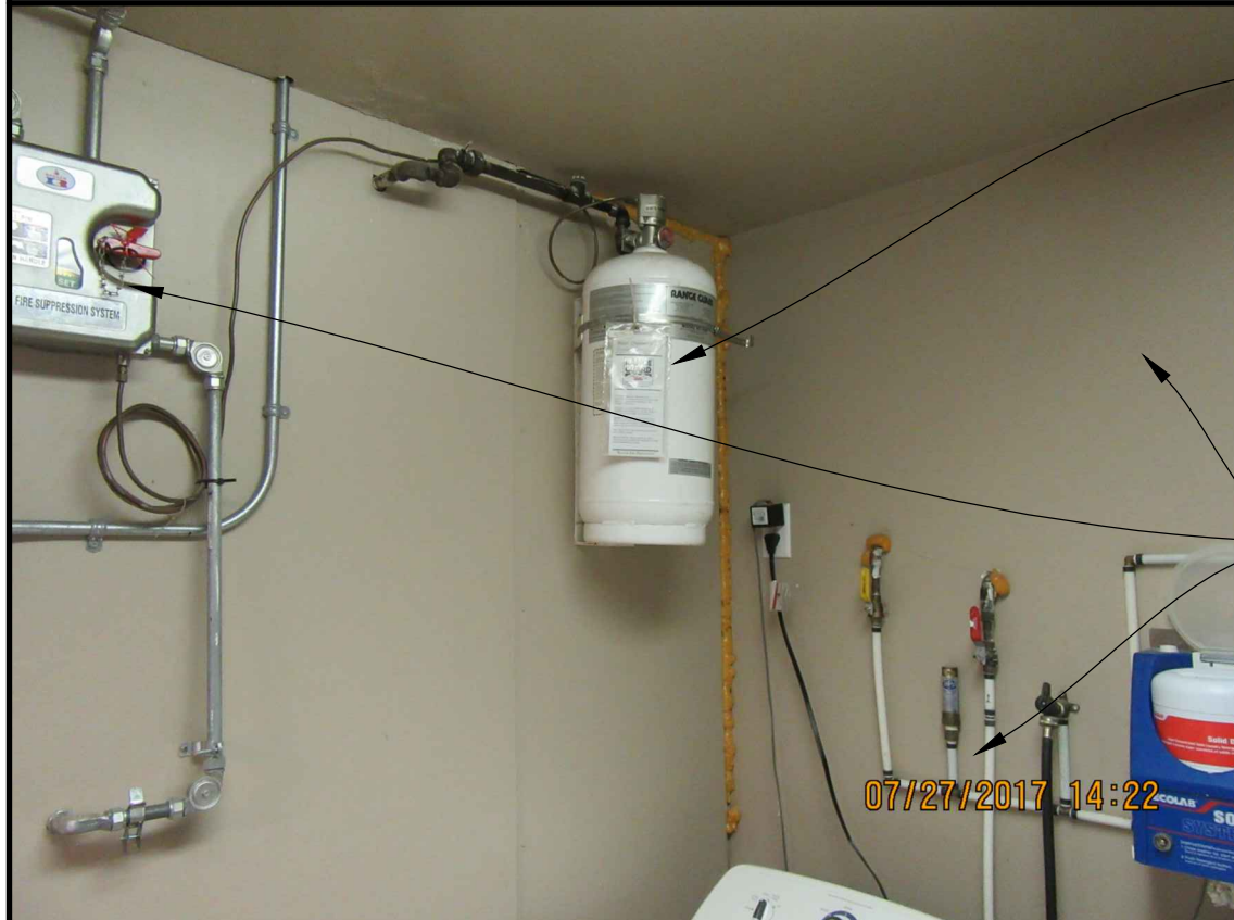
17 PHOTO OF EXISTING CONDITION
