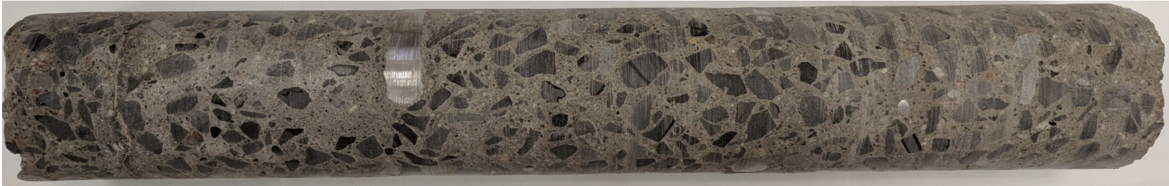
CH4-2 – East Abutment – 300 mm to 850 mm
