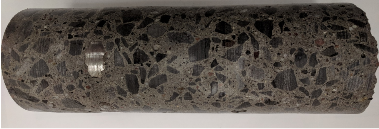
CH4-1 – East Abutment – 0 mm to 300 mm
