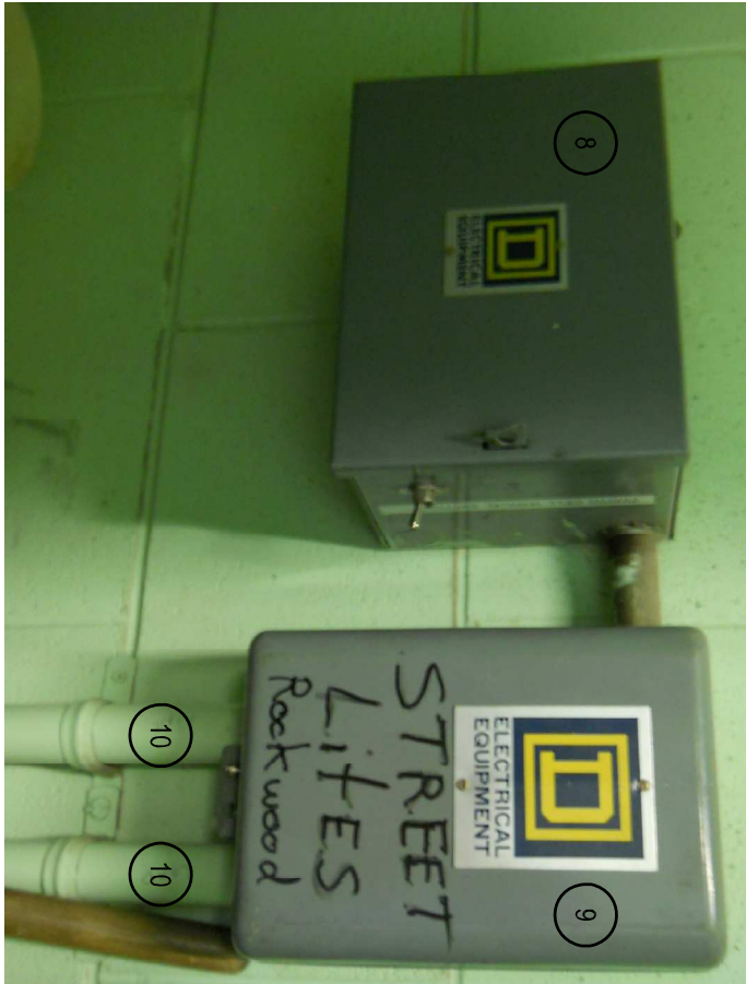
4 E2 N1.S C12 - POWERHOUSE STREET LIGHTS CONTROLLER AND CONTACTOR
