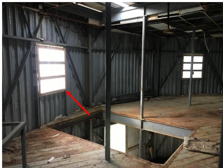
Photo 2: View of 2 nd floor of Building 1. Asbestos-containing grey caulking located around all windows (DST Sample 29911-1-01A) and grey floor paint (DST Sample 29911-1-LP-02).
