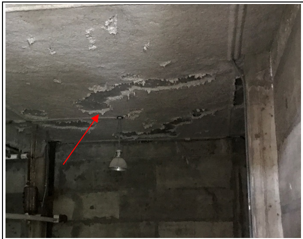
Photo 24: Building 3 – Asbestos-containing (10% chrysotile) sprayed fireproofing located in the storage room.
