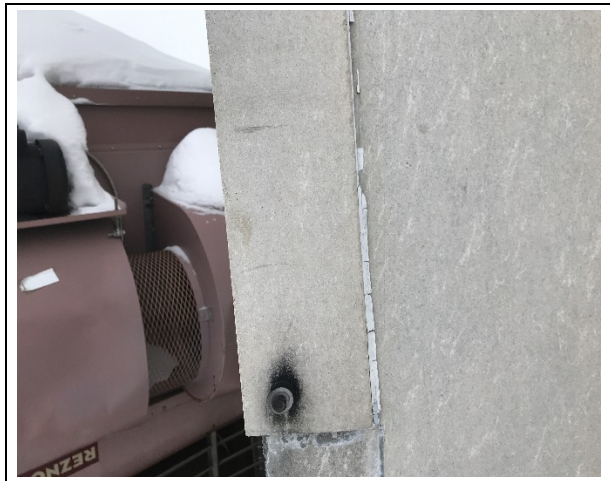
Photo 40: Building 4 – Asbestos-containing (5% chrysotile) exterior caulking – grey located on the exterior walls.
