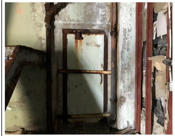
Photo 30: Building 3 – Presumed asbestos-containing fire rated door located in the entrance.
