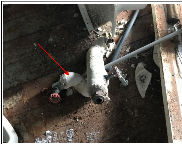
Photo 7: Building 1A – Asbestos-containing (65% chrysotile) insulating cement on pipe fittings observed debris on floor.
