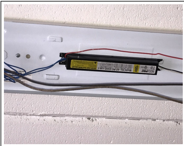
Photo 43: Building 4 – Non-PCB-containing electric ballast associated with the light fixture in office 1.
