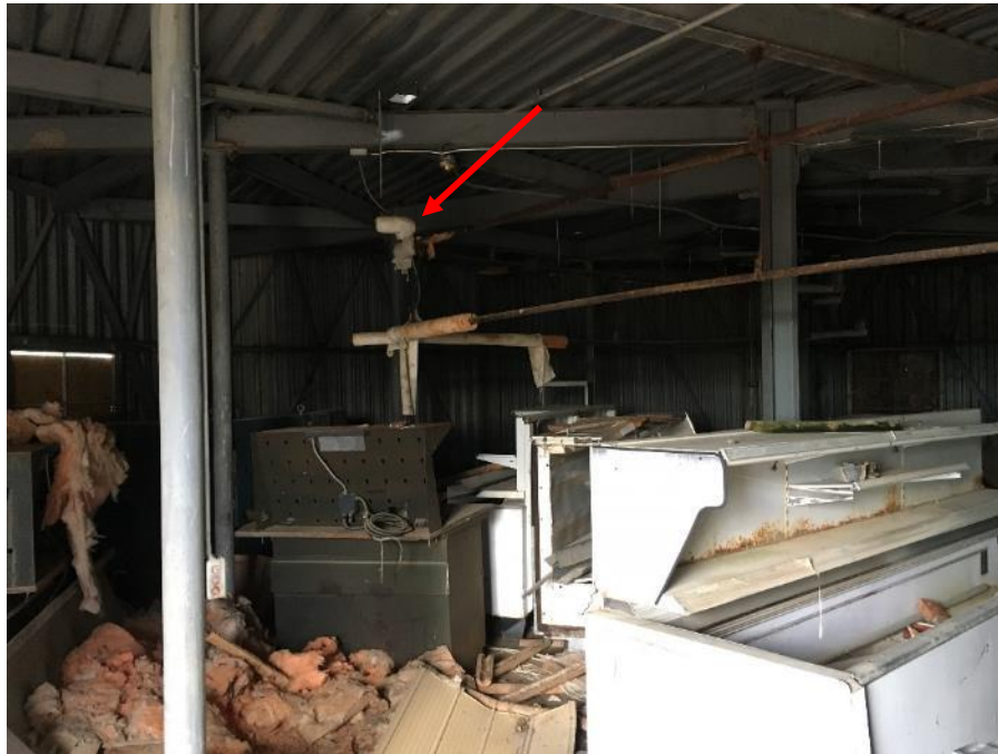
Photo 5: View of asbestos-containing grey cement compound on pipe fittings (DST Sample 29911-1A-01A) and old grocery display refrigeration units, located in Building 1A.
