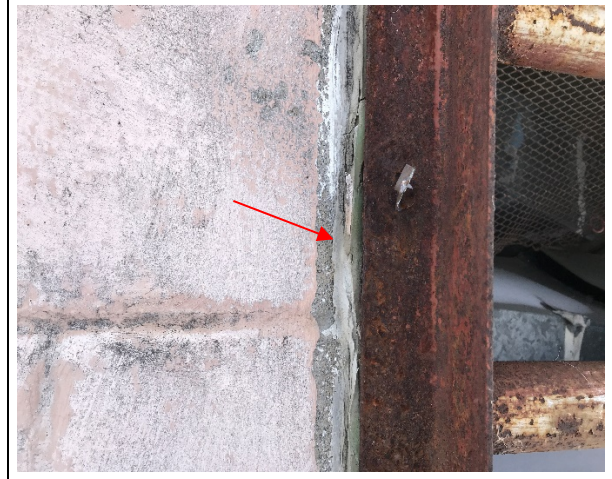
Photo 14: Building 2 – Asbestos-containing (1.7% chrysotile) exterior caulk – grey located on the exterior of the building (north vent).
