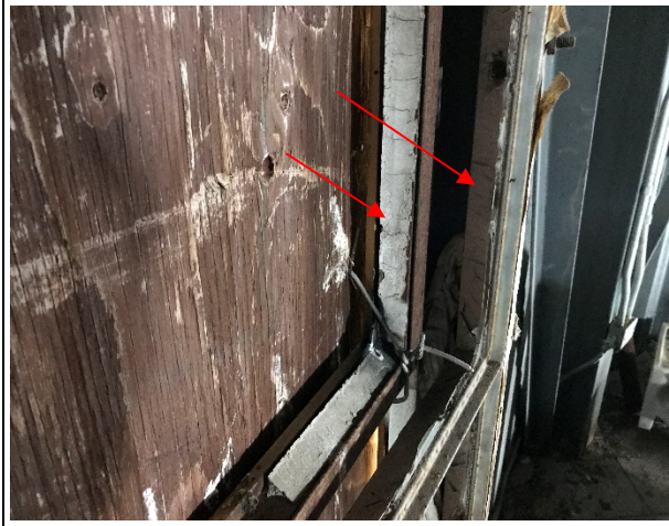
Photo 9: Building 1A – Asbestos-containing (2% chrysotile) interior window glaze compound – grey.
