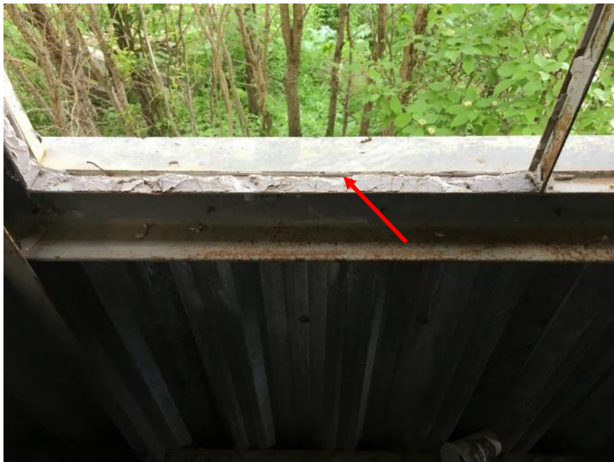
Photo 7: View of asbestos-containing grey window caulking (DST Sample 29911-1A-03A) observed around all windows throughout Building 1A.
