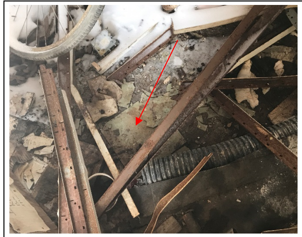
Photo 16: Building 2 – Asbestos-containing (1.2% chrysotile) mastic associated with 9"x9" vinyl floor tile – green located in room 2.
