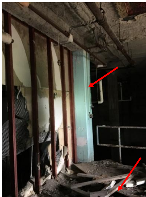
Photo 12: View of lead-containing blue paint (DST Sample 29911-3-LP-01, non-hazardous for disposal) and asbestos-containing fireproofing debris, observed on the Ground Floor of Building 3.
