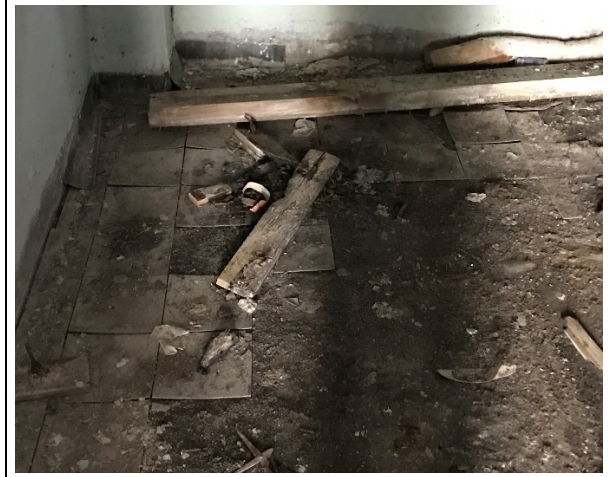
Photo 26: Building 3 – Asbestos-containing (2% chrysotile) 9"x9" vinyl floor tile – grey located in the entrance.
