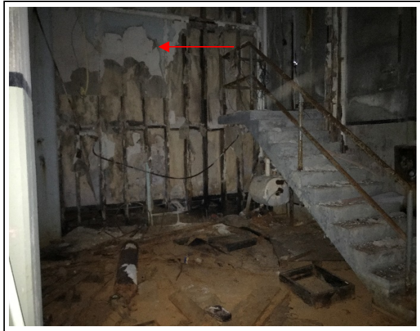
Photo 28: Building 3 – Asbestos-containing (2% chrysotile) drywall joint-fill compound located in the storage room.
