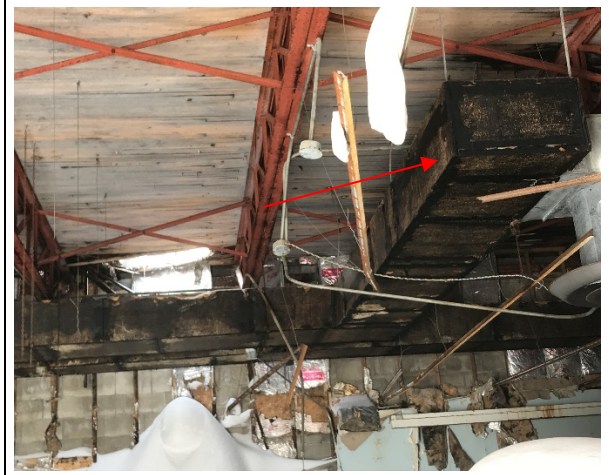
Photo 18: Building 2 – Presumed asbestos-containing duct insulation – black located in room 2.
