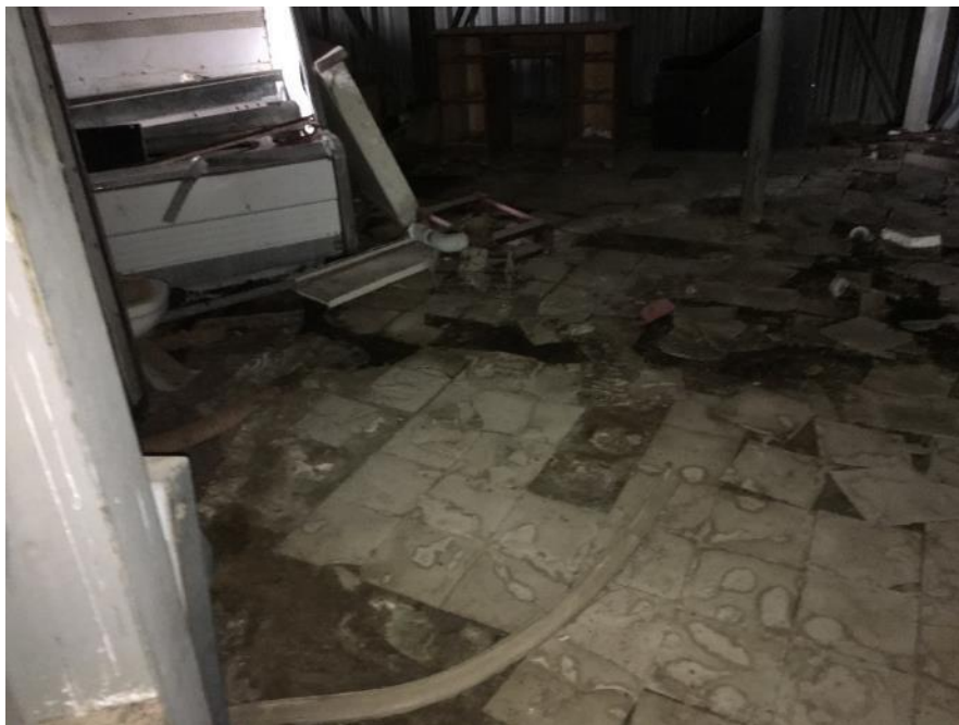
Photo 6: Asbestos-containing beige 9"x9" vinyl floor tiles (DST Sample 29911-1A-02A), observed on the main floor of Building 1A). The associated mastic was found to not contain asbestos.
