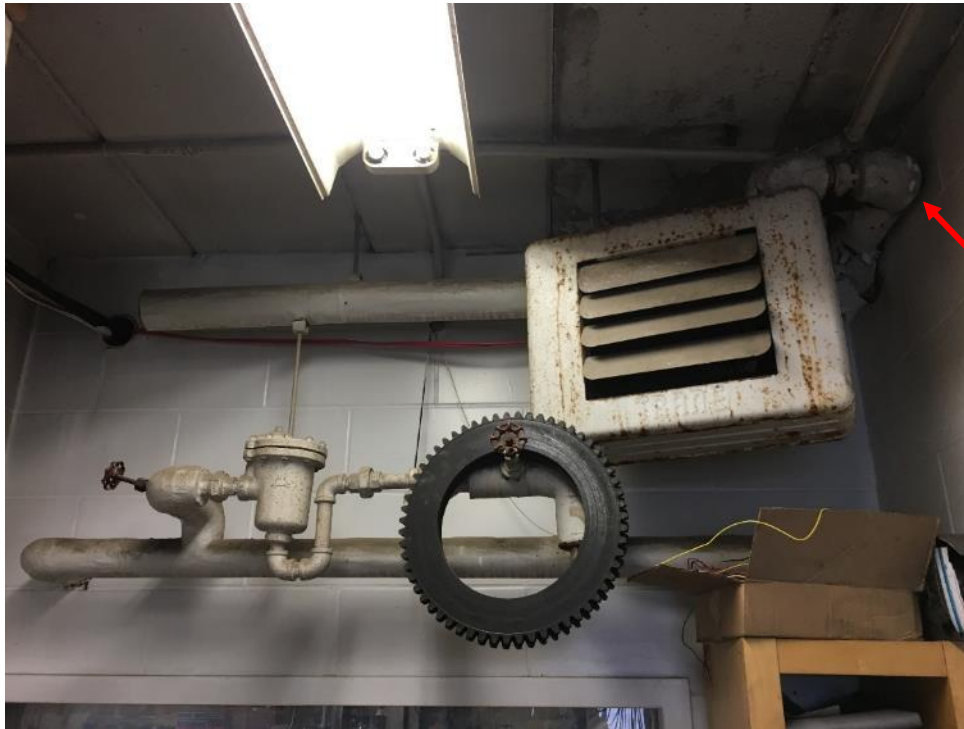
Photo 15: View of asbestos-containing grey cement compound on pipe fittings (DST 2006 Sample 353-04-MI-01) in a small workshop, observed throughout Building 4.
