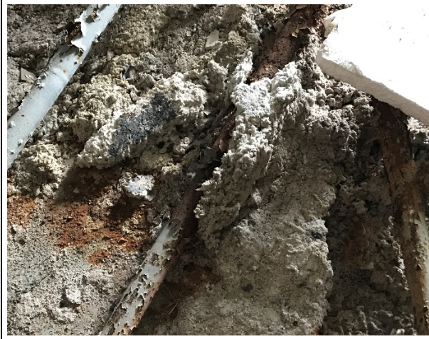
Photo 25: Building 3 – Asbestos-containing (10% chrysotile) sprayed fireproofing debris located on the floor in the entrance.
