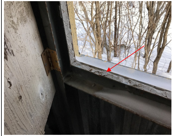
Photo 2: Building 1 – Asbestos-containing (2% chrysotile) interior window glaze compound – grey observed to be in poor condition (cracking).
