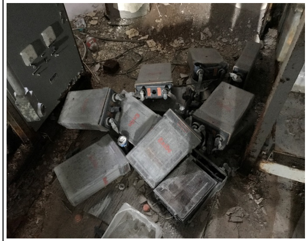
Photo 34: Building 3 – Suspect mercury containing batteries located in the communications room.
