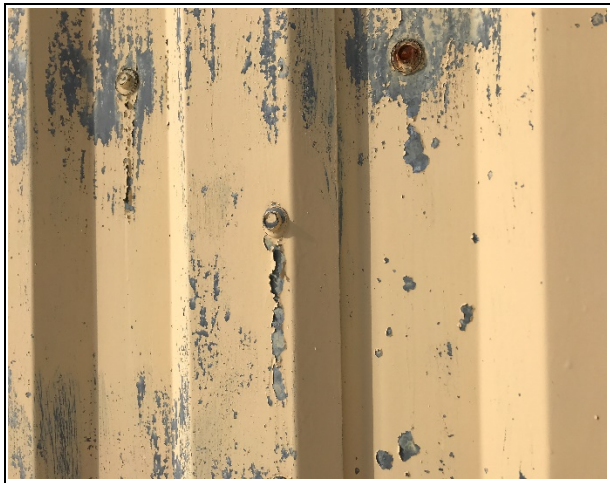
Photo 4: Building 1 – lead-containing (350 ppm) yellow/grey coloured paint on the exterior metal cladding.
