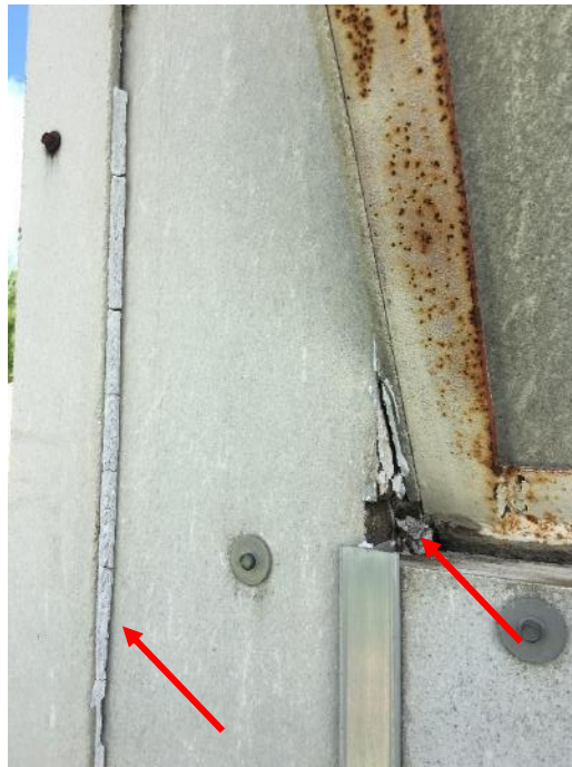
Photo 16: Asbestos-containing caulking (DST Sample 29911-4-04A) observed throughout the exterior of Building 4, between Transite paneling.
