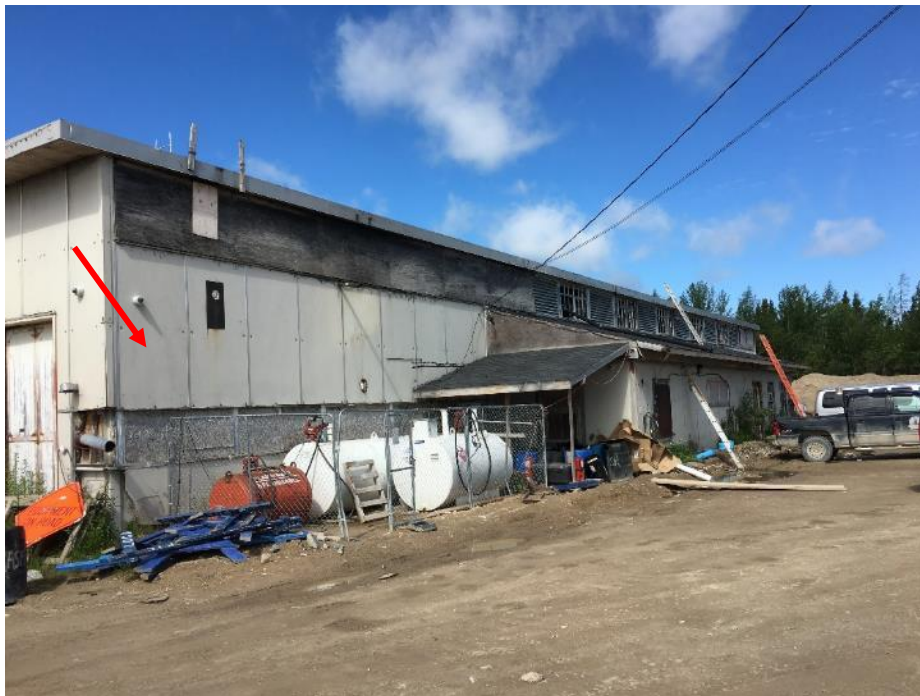
Photo 14: View of Building 4 with asbestos-containing Transite exterior wall paneling (DST Sample 29911-4-01A). One (1) 1,000-gallon diesel, one (1) 500-gallon gasoline and one (1) 250-gallon red re-fueling tank are present at the building's exterior.
