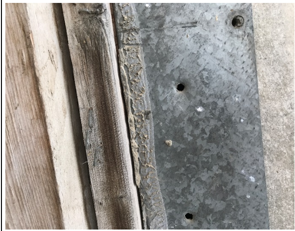
Photo 41: Building 4 – Asbestos-containing (2% chrysotile) exterior window caulking – grey located on the storage room window.
