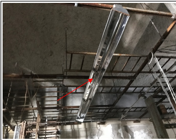
Photo 35: Building 3 – Suspect PCB-containing ballasts associated with light fixtures.
