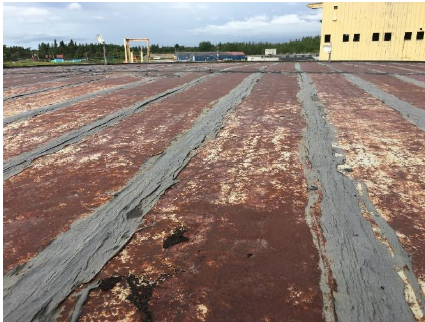
Photo 3: View of asbestos-containing black tar located on roof top of Building 1 (DST Sample 29911-1-03A).
