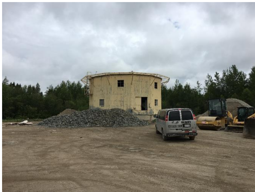
Photo 4: View of Building 1A with lead-containing yellow paint on metal cladding (DST 2006, 353-1A-LP-01). This paint has been identified as leachate hazardous with respect to lead.
