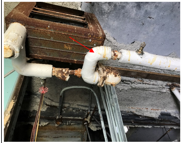
Photo 22: Building 3 – Asbestos-containing (65% chrysotile) insulating cement on pipe fittings located in the entrance.
