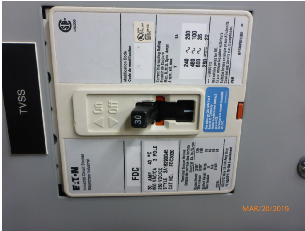
Image 5: Building A3 – Board A3-PL-002.N sample TVSS breaker
