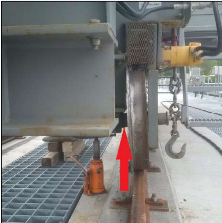
Figure 12 - Drive shaft of Ontario stoplog lifter, showing approximate location of crack. The crack on the Quebec lifter's shaft was in approximately the same place.
