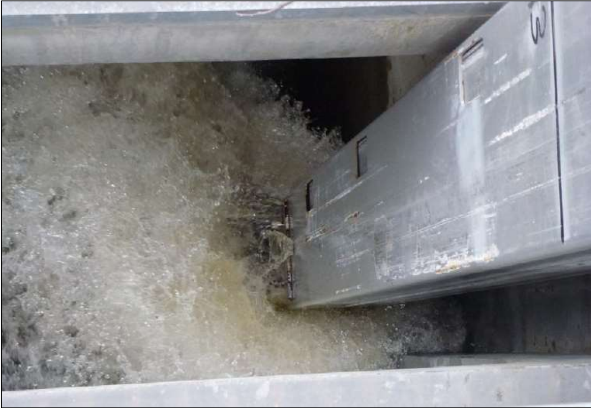
Figure 10 - Boom of Ontario stoplog lifter placing stoplog in sluice. Note turbulence.
