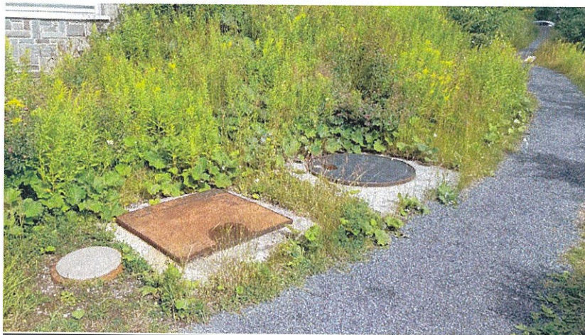
Figure 3. Existing fuel transfer station (left) and entrance/ manhole (right) to underground fuel storage tank that will be demolished and replaced.
