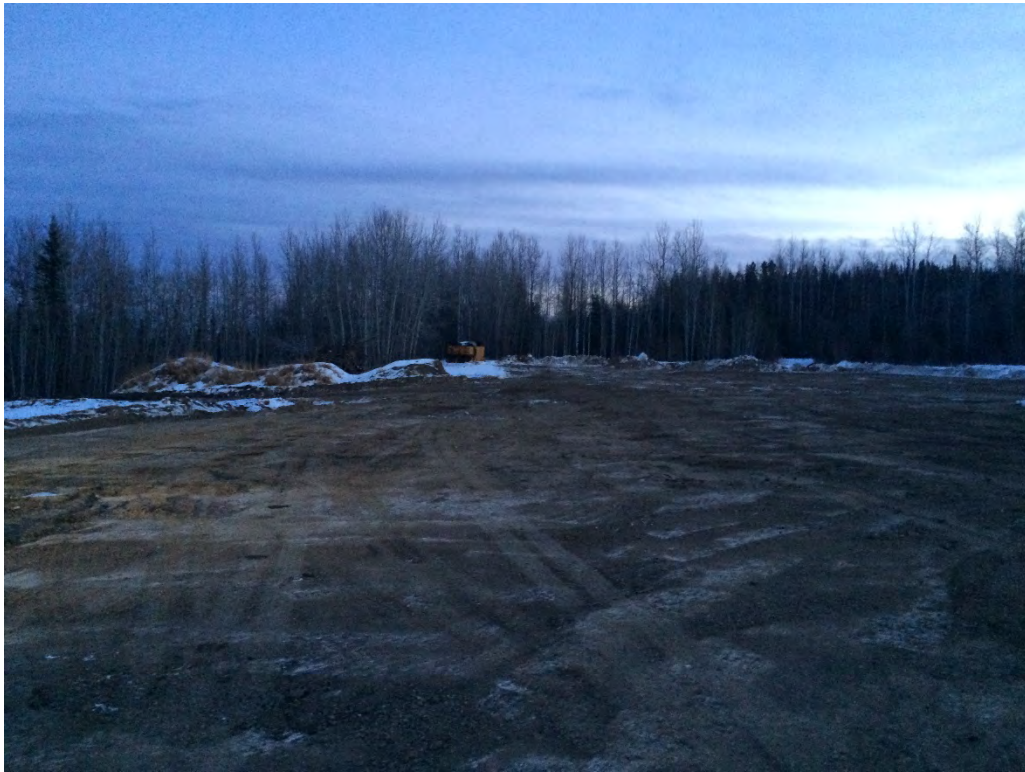
Photograph 2: View of K19 during stockpile removal (December 2018).
