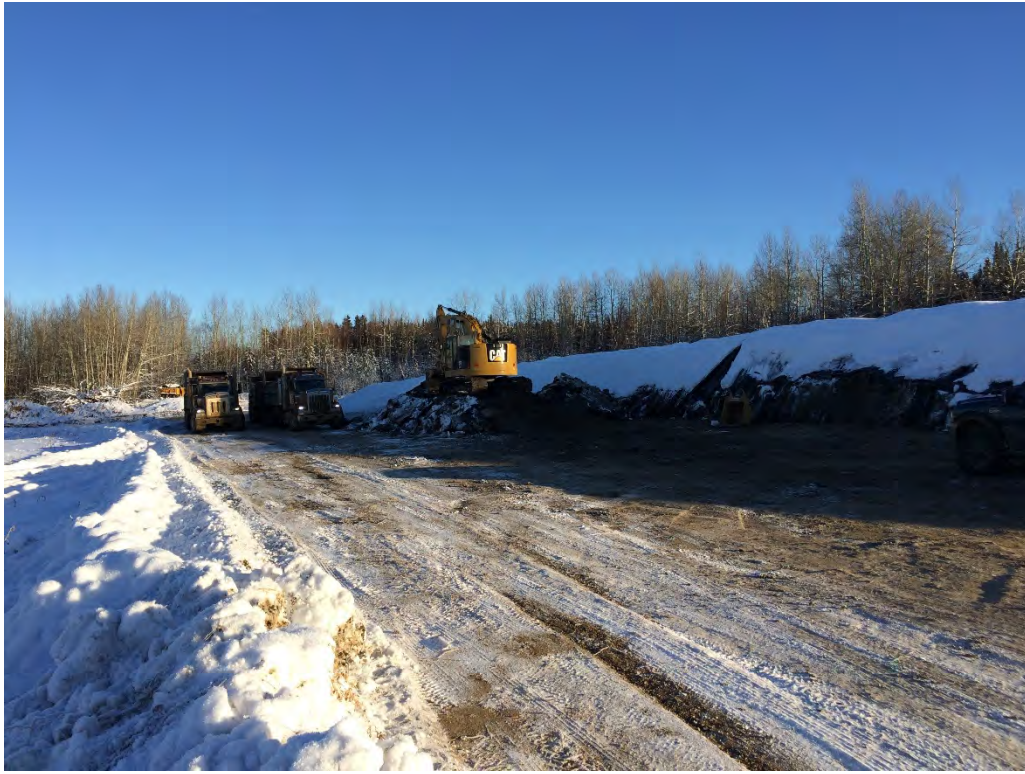
Photograph 1: View of K19 during stockpile removal (December 2018).
