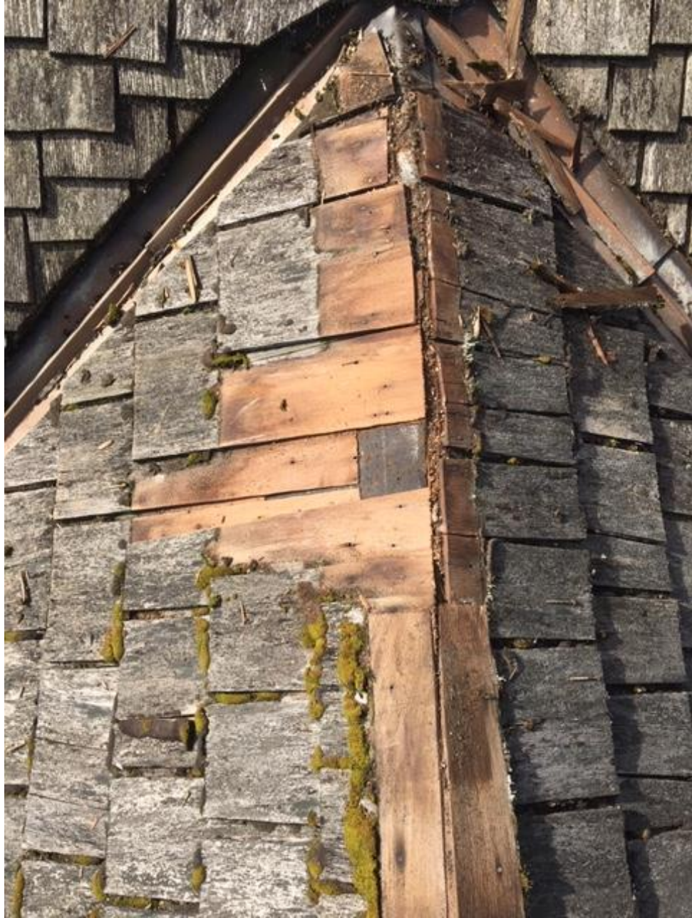
Lodge Building - Non-asbestos felt beneath cedar shingles.
