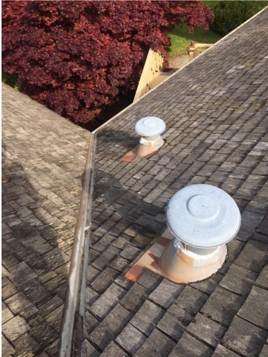
Lodge Building - Non-asbestos caulking on roof vents.
