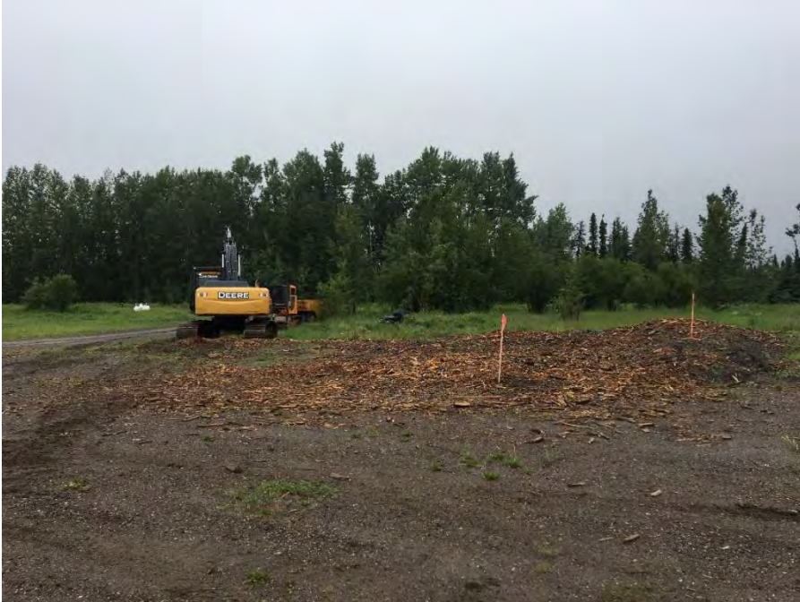
Photo 1: Backfilled test pit in AEC 1b, looking NW
