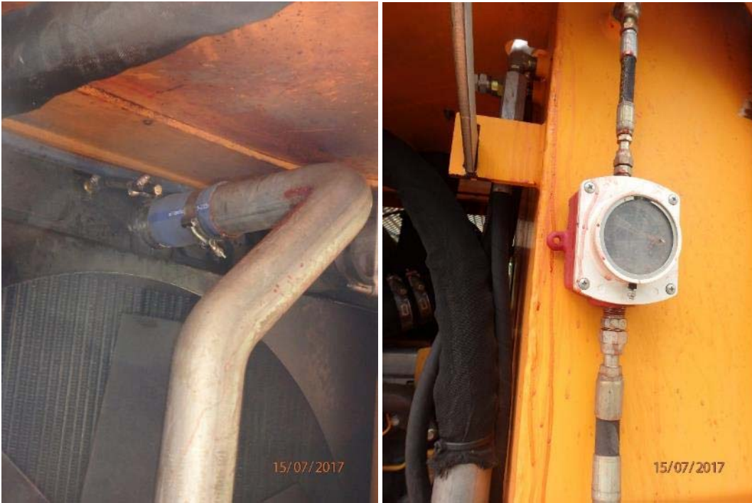
Photo 3: The pipe and hose that came loose in the mulcher causing antifreeze to leak (left photo) and antifreeze on the interior wall of the mulcher cage, which was able to contain the release(right photo).
