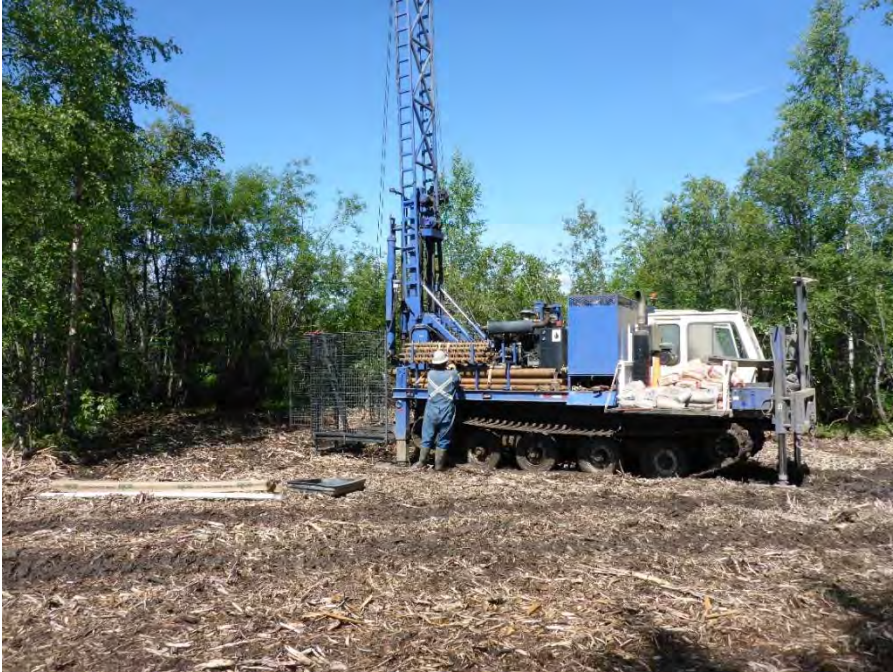
Photo 13: Drilling K19-MW17-17 AEC 26, Tundra Environmental Drilling
