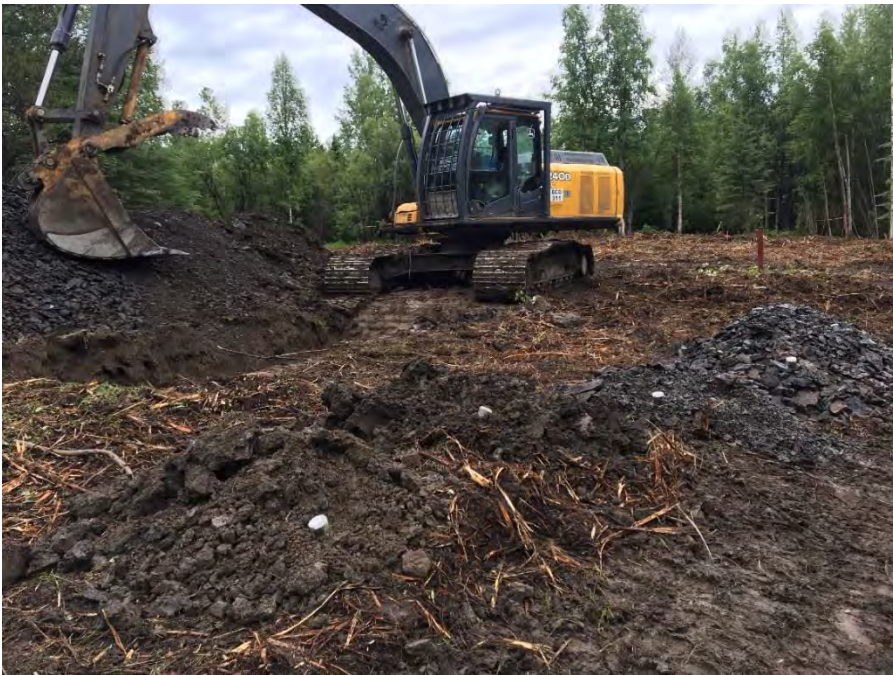
Photo 2: Test pitting activities at K19-TP17-61 APEC 13, looking S
