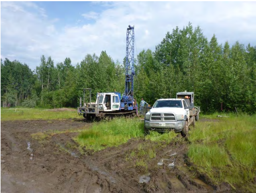
Photo 16: Monitoring well installation at K19-MW17-20 APEC 6, Tundra Environmental Drilling
