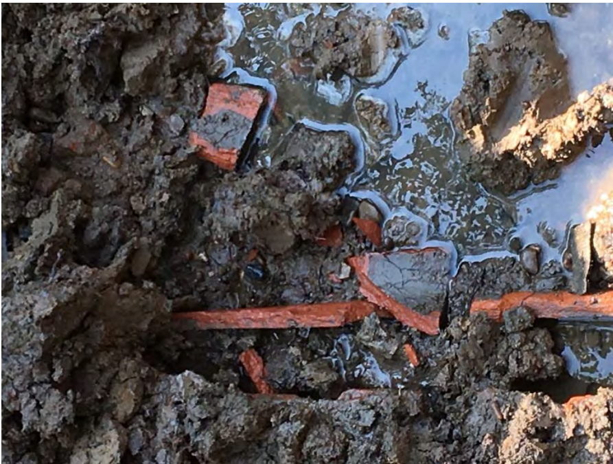
Photo 4: Clay pipe identified during the excavation of K19-TP17-57 APEC 4
