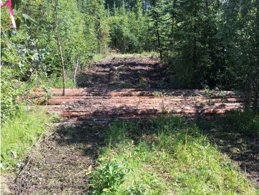
Photo 5: Completed log bridge for accessing APEC 26, looking NE
