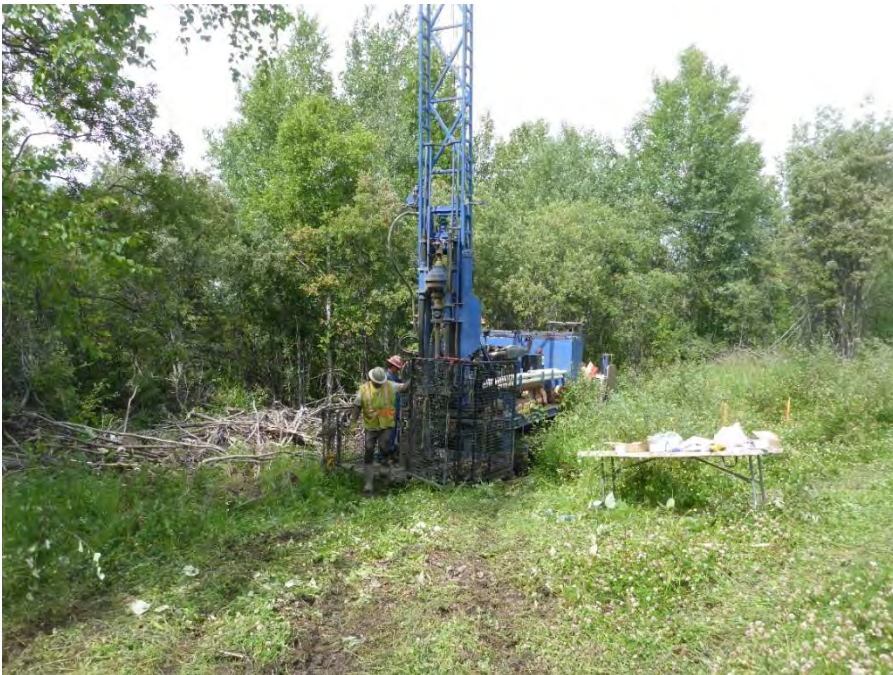
Photo 18: Drilling K19-MW17-33 APEC 14, Tundra Environmental Drilling
