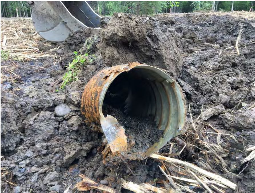
Photo 8: Culvert identified during the excavation of K19-TP17-86 APEC 13
