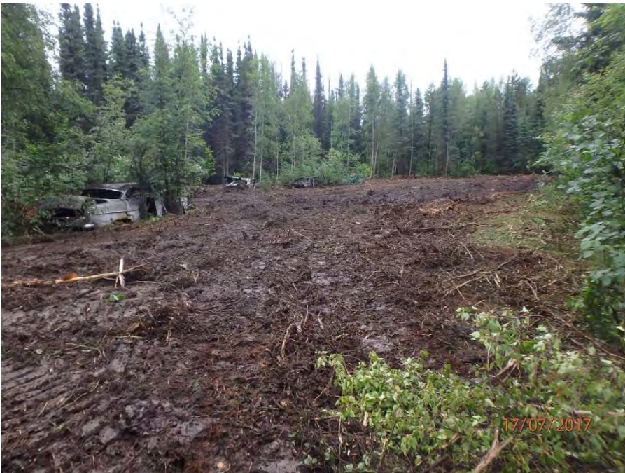
Photo 12: Partially mulched vegetation at APEC 12, looking N
