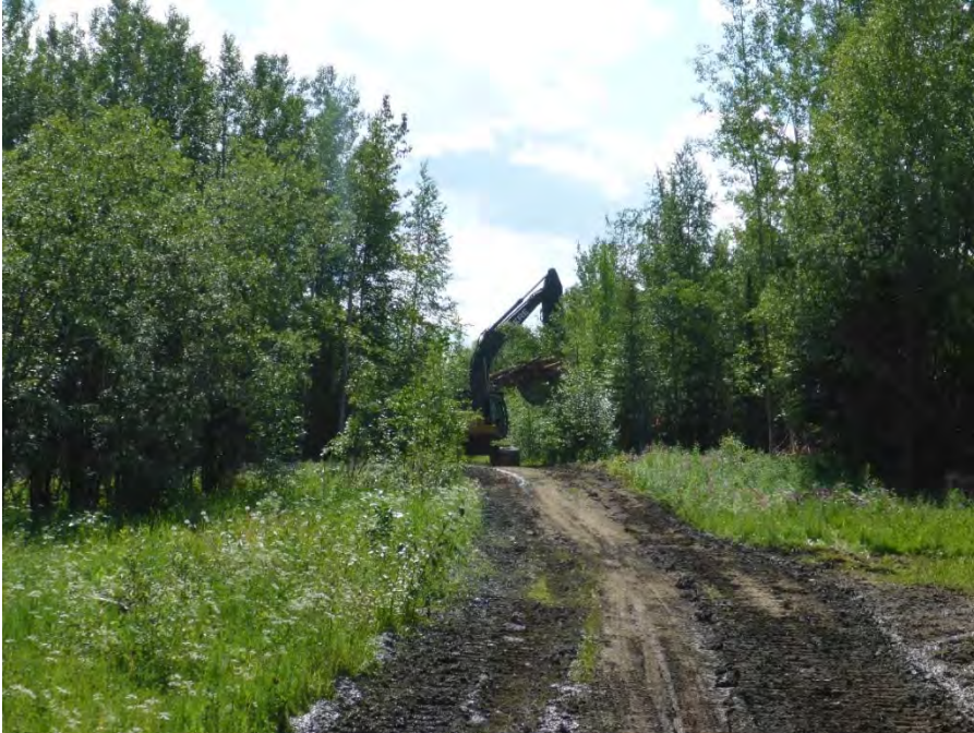
Photo 15: Excavator removing logs from Site onto neighboring property
