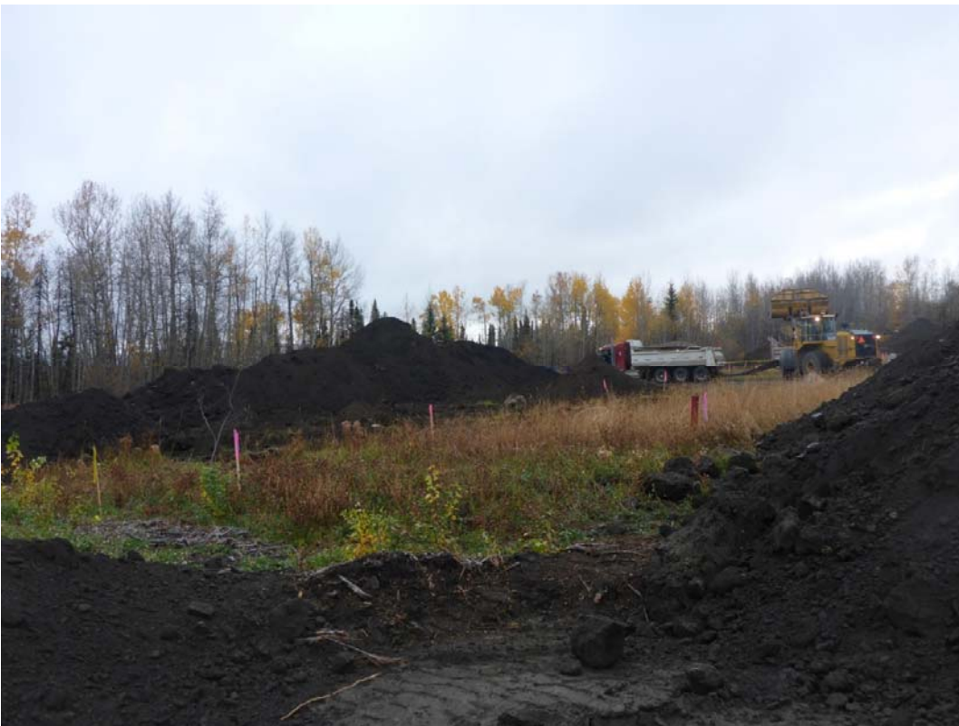
Photograph 2: Haul truck being loaded with material for off-Site disposal.
