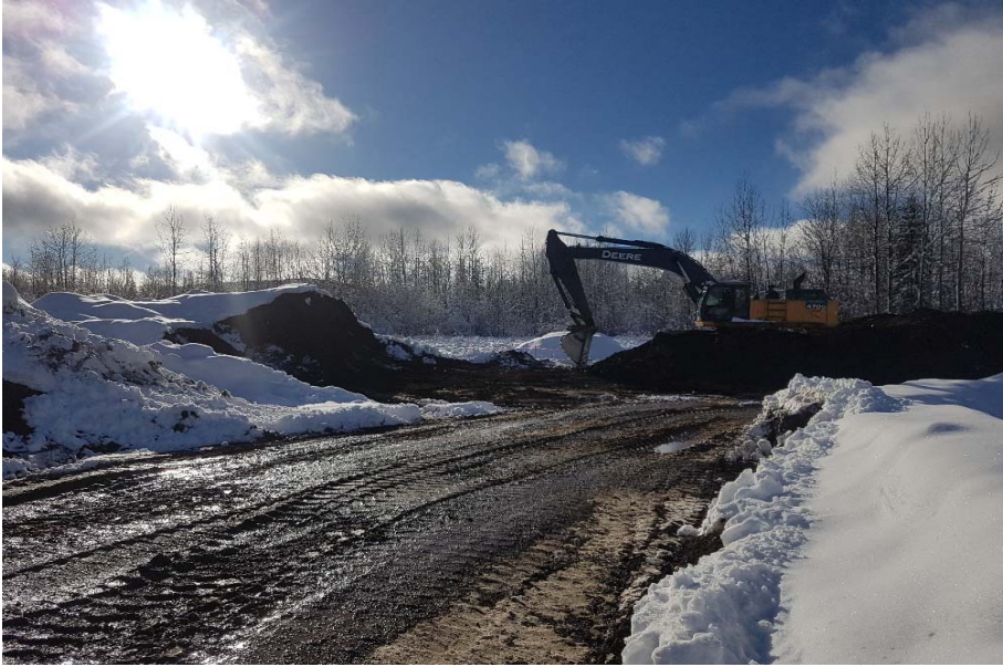
Photograph 1: stockpile management, moving the stockpiles in preparation to start AEC 1C
