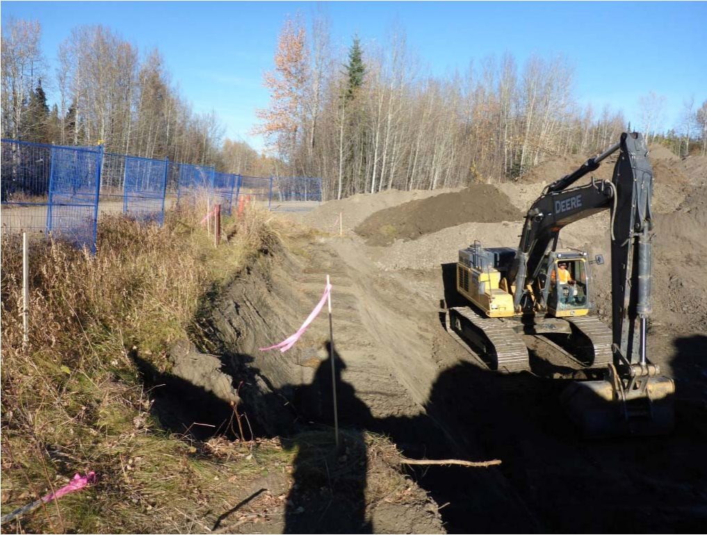
Photograph 3: Excavation of overburden in cells N2, O2 and P2, looking northeast.
