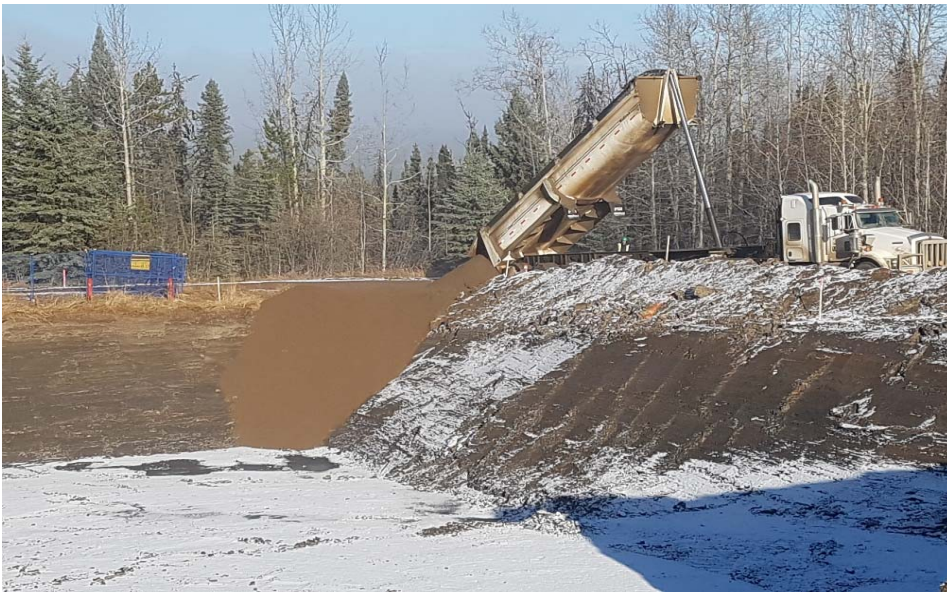
Photograph 2: Backfilling AEC 1B cell P2
