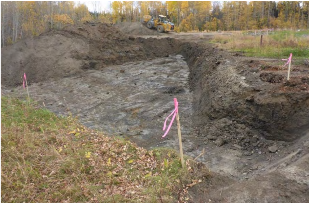
Photo 2: Excavation of overburden in northern section of AEC 1B looking north-east.
