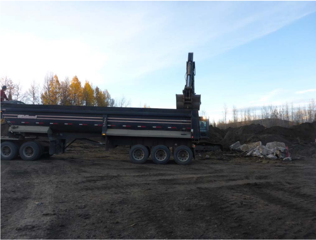
Photograph 1: Loading of oversize concrete material for off-Site disposal.
