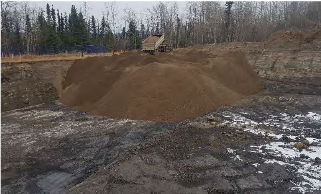
Photo 22: Continued backfilling of north-east of AEC 1B looking towards the north-west.
