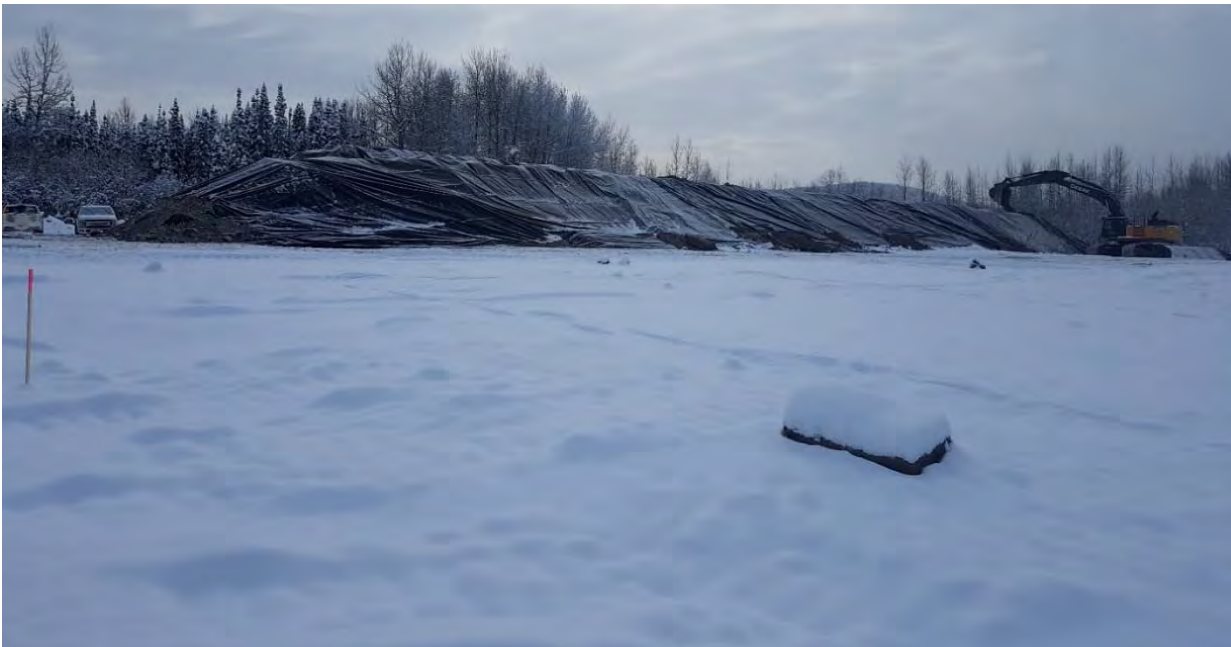
Photo 46: AEC 1C inferred impacted material stockpile covered with poly liner.
