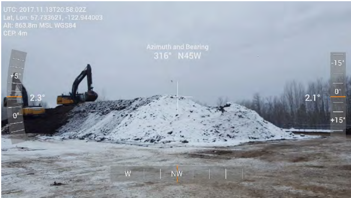
Photo 43: AEC 1C inferred impacted material windrowing.
