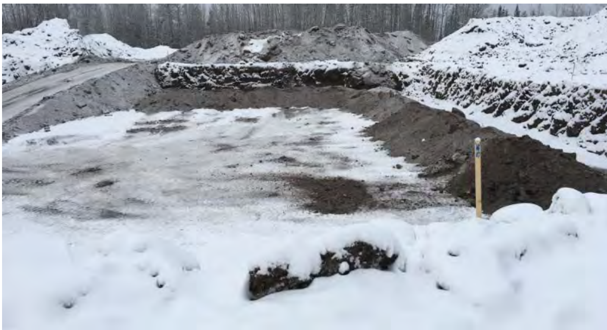
Photo 44: Backfilling of AEC 1C looking towards the west.
