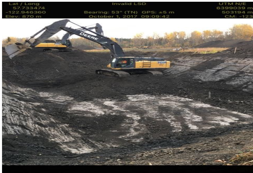
Photograph No. 1 – Photograph taken by Tervita personnel on-site at Trutch, British Columbia showing Tangle Ridge Custom Crushing Ltd. Clearing overburden material and cleaning up slope debris. – October 1 st , 2017.
