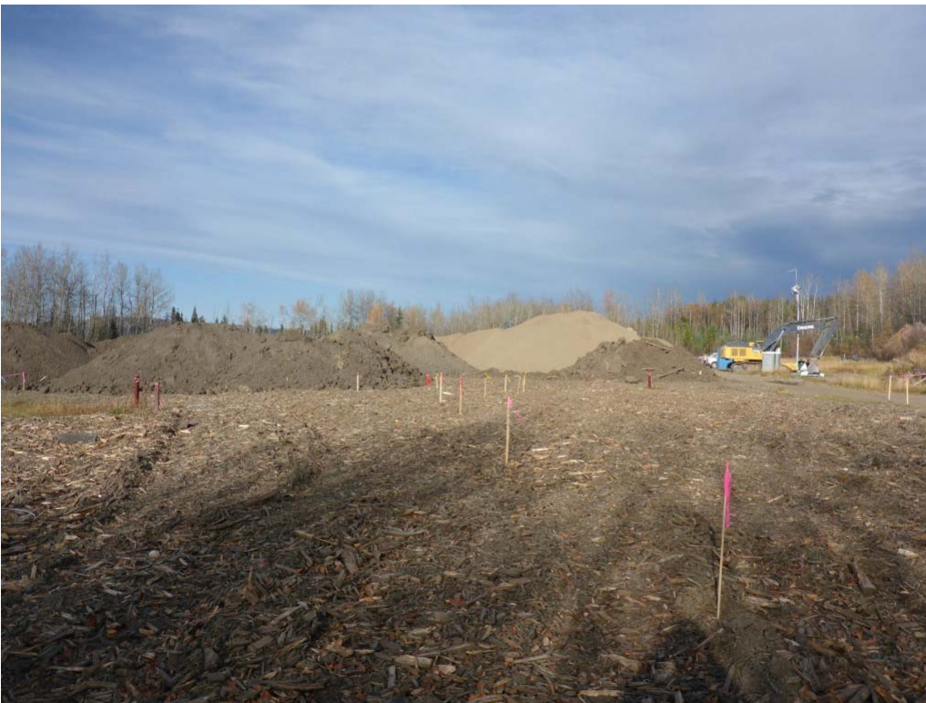
Photograph 4: On-Site stockpiled material, looking north.
