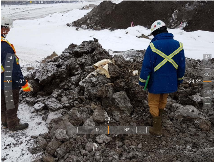
Photograph 1: Stockpiled material that was impacted from the hydraulic leak from the 470G LC excavator, looking north.
