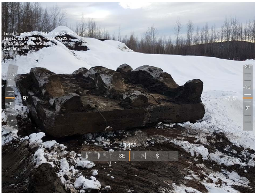
Photograph 2: Concrete removed near cells J2 and K2, looking southeast
