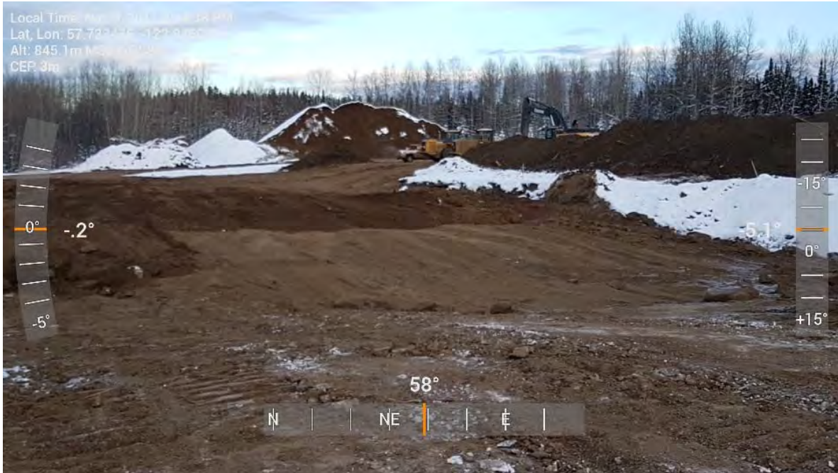
Photo 39: Continued backfilling of AEC 1B looking towards the north-east.
