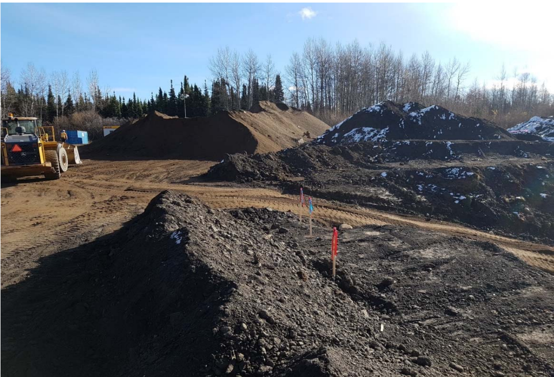
Photograph 2: Backfill stockpiled onsite looking South from Hazardous Waste Cell.
