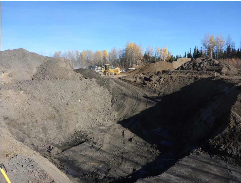
Photograph 4: Completion of ramp into cells G2 and H2, looking east.
