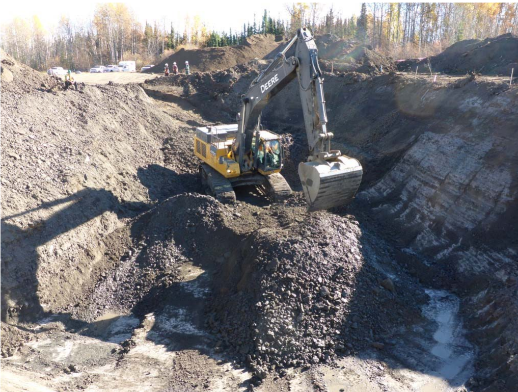
Photograph 2: Excavation in AEC 1b in cells H2 and H3, looking east.
