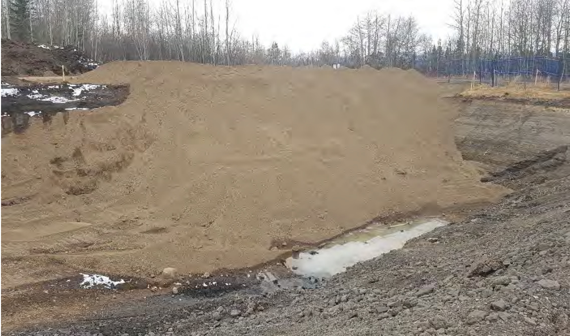
Photo 15: Completed haul road across excavation 1B looking towards the south-west.
