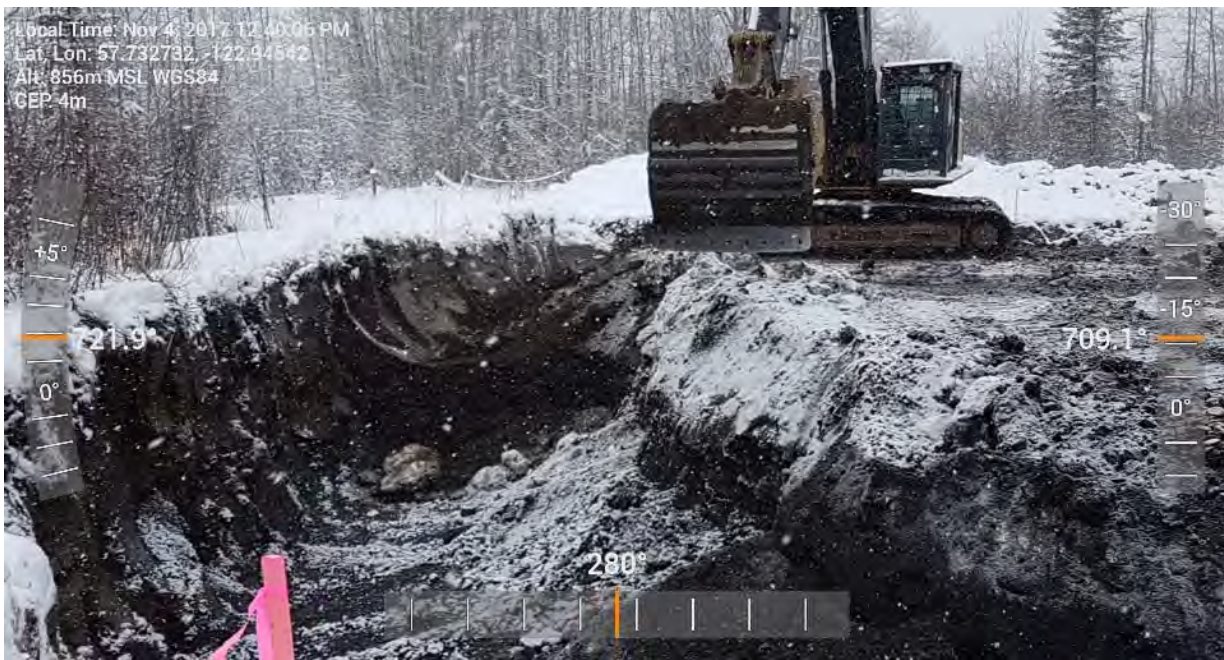
Photo 34: Excavation of inferred impacted material along the southern edge of AEC 1C looking towards the west.
