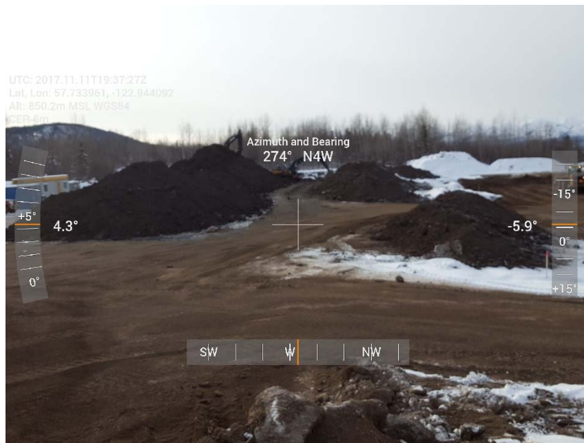
Photograph 2: Backfill progress in AEC 1b, looking west.
