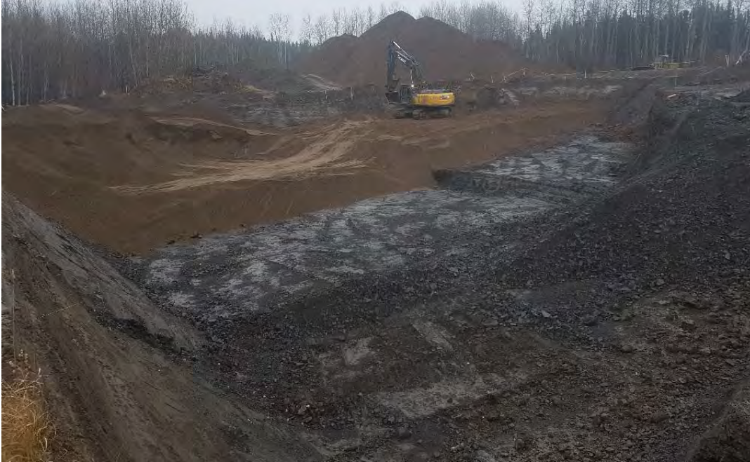
Photo 23: Backfilling north-east portion of AEC 1B looking towards the north-east.
