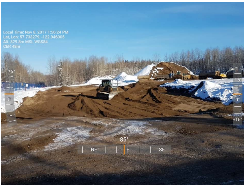
Photograph 2: Backfill progress of the excavation in AEC 1b, looking east.
