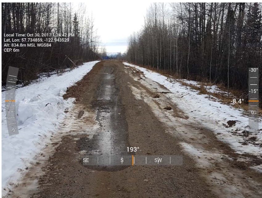
Photograph 2: Spill of engine coolant along the haul road approximately 50m northeast of the Site, looking south
