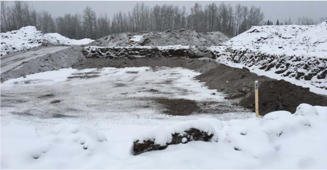
Photograph 1: View of backfill progression in AEC 1C
