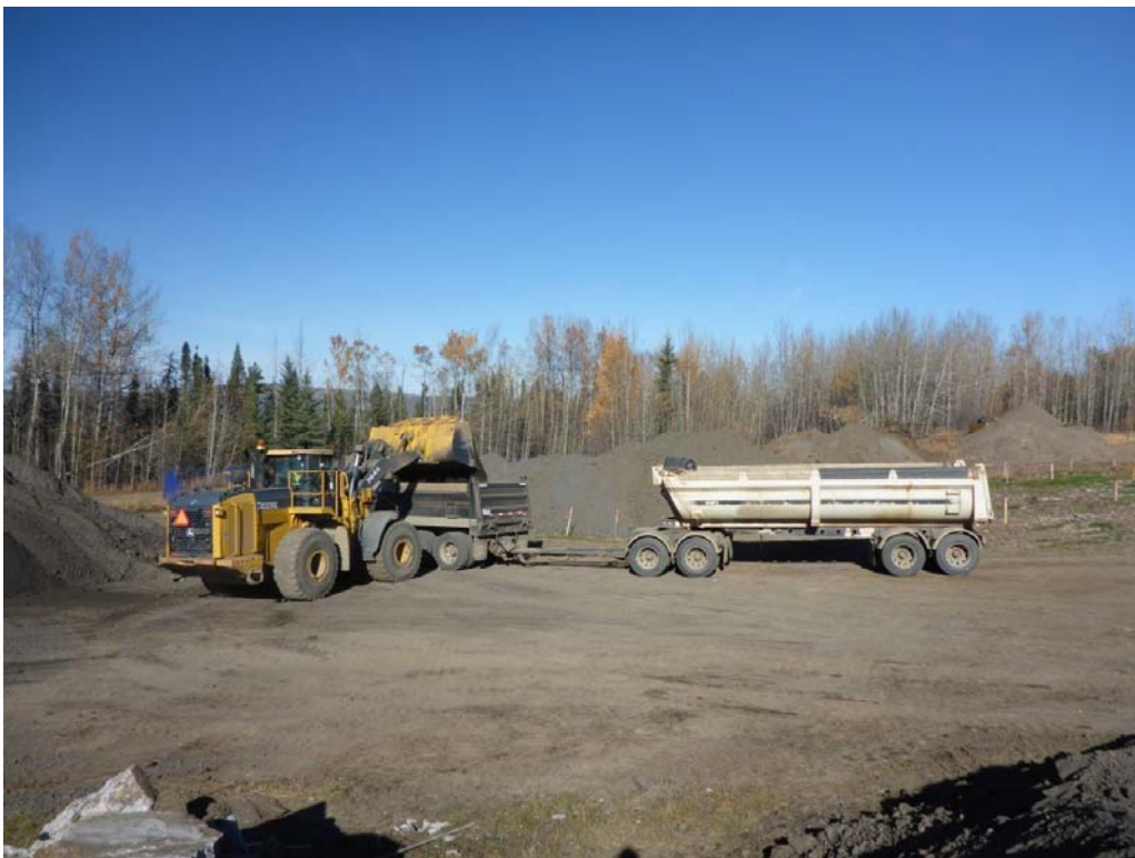
Photograph 2: Haul truck being loaded with material for off-site disposal, looking east .
