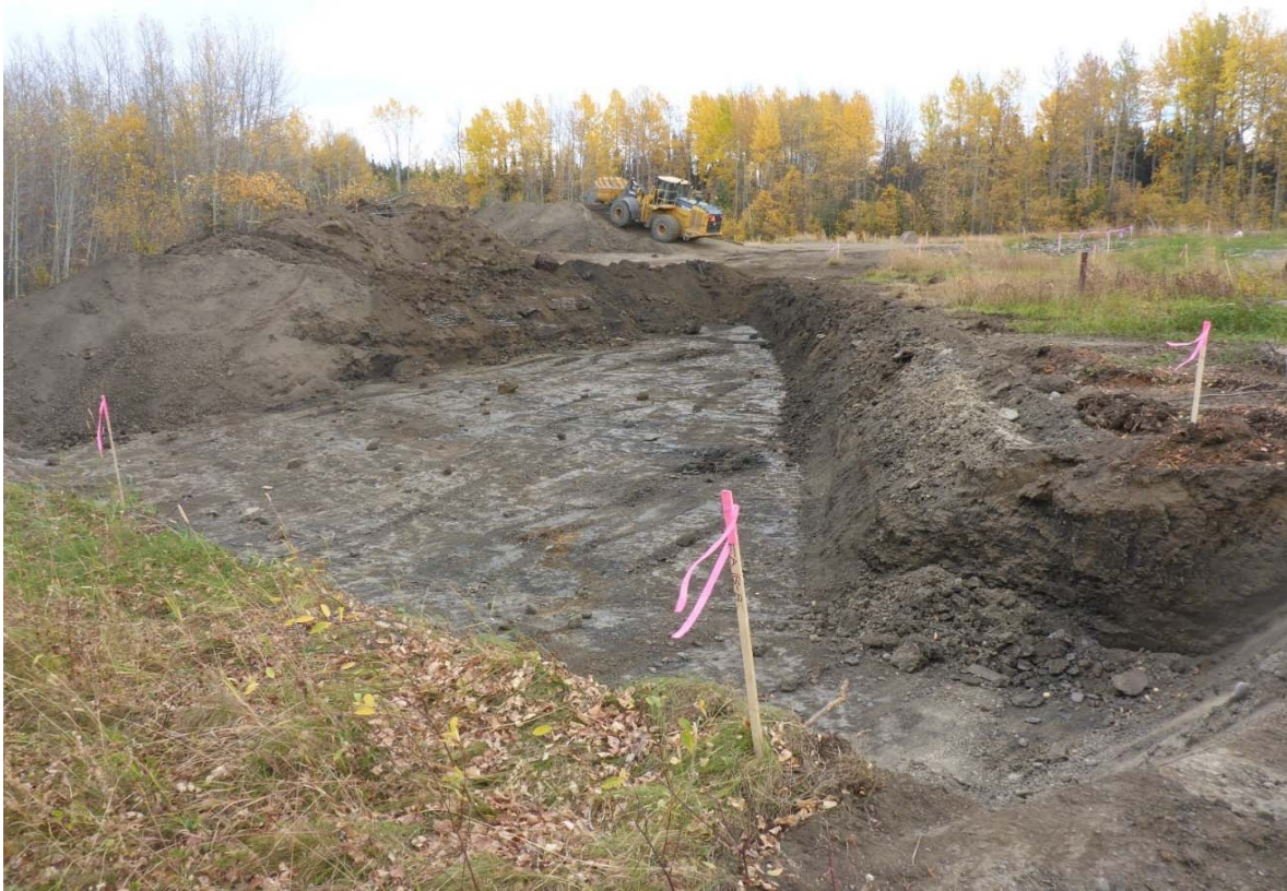
Excavated overburden in northern section of AEC 1b
