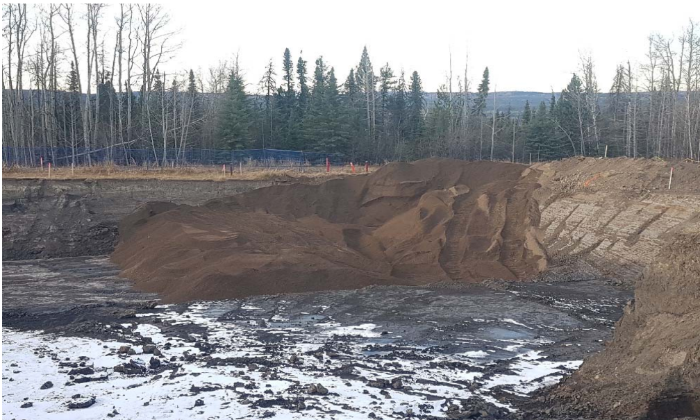
Photograph 2: Backfilling AEC 1b cell P2, P3, O2 and O3.
