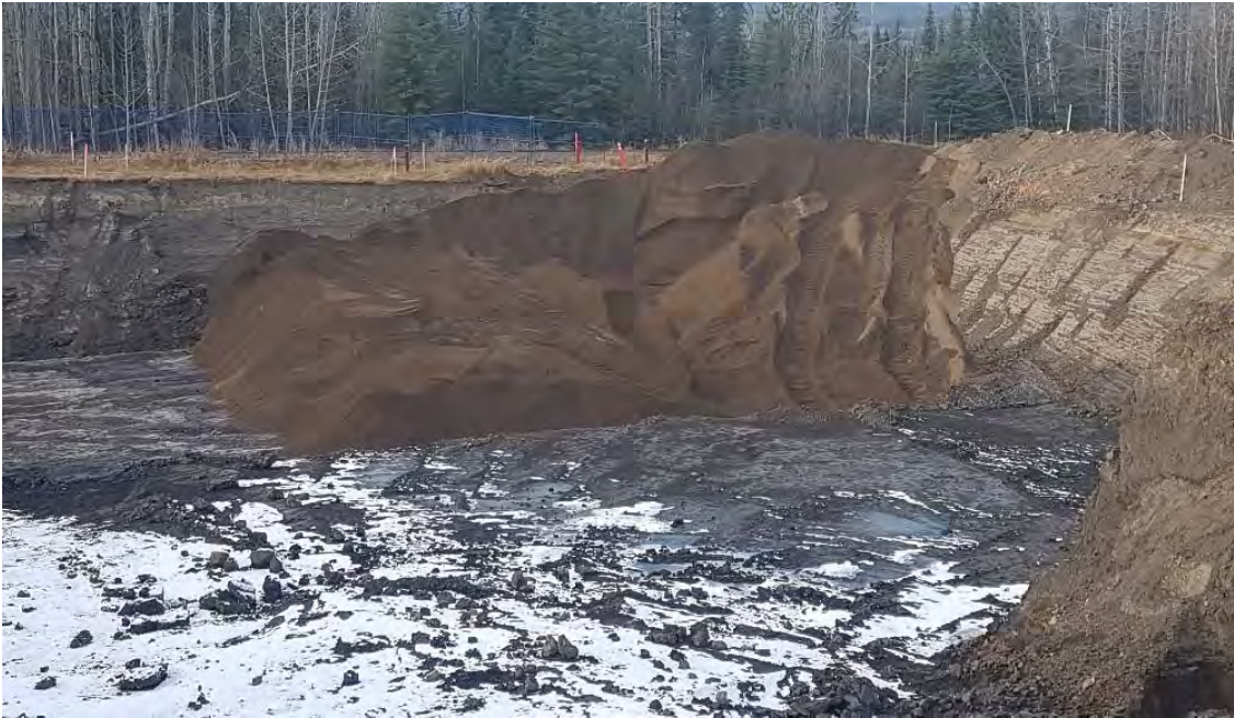
Photo 21: Continued backfilling of north-east of AEC 1B looking towards the north-west.
