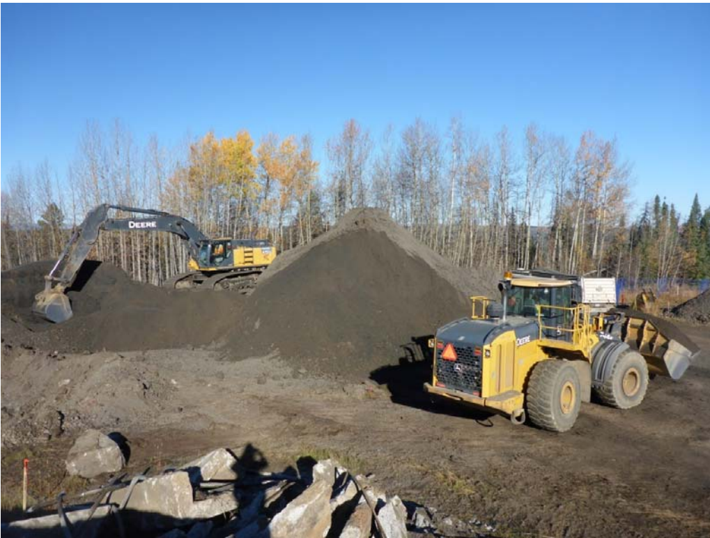
Photograph 4: Excavator stockpiling material in AEC 1b, looking northwest.
