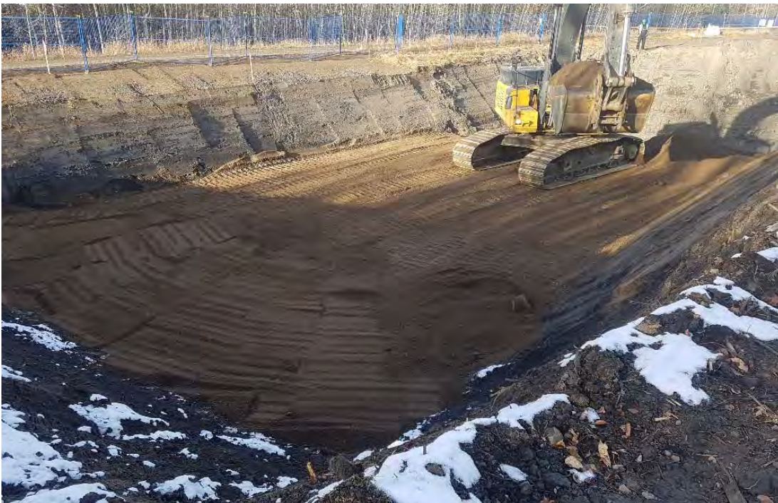
Photo 10: Backfilling southern portion of AEC 1B looking towards the north-west.
