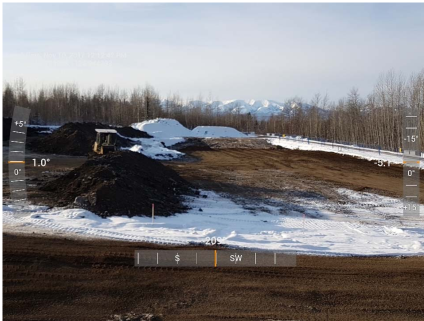
Photograph 2: Backfill progress in AEC 1b, looking southwest.
