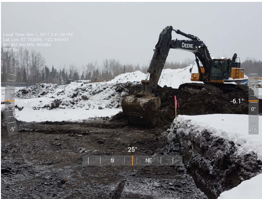
Photograph 1: Backfilling in AEC 1b including cells J2 to L2, looking north
