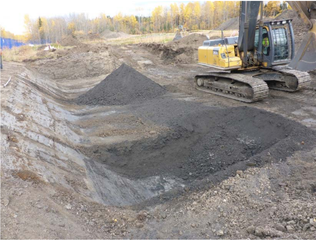
Excavation of impacted material between 2 and 3 m bgs in cell F2
