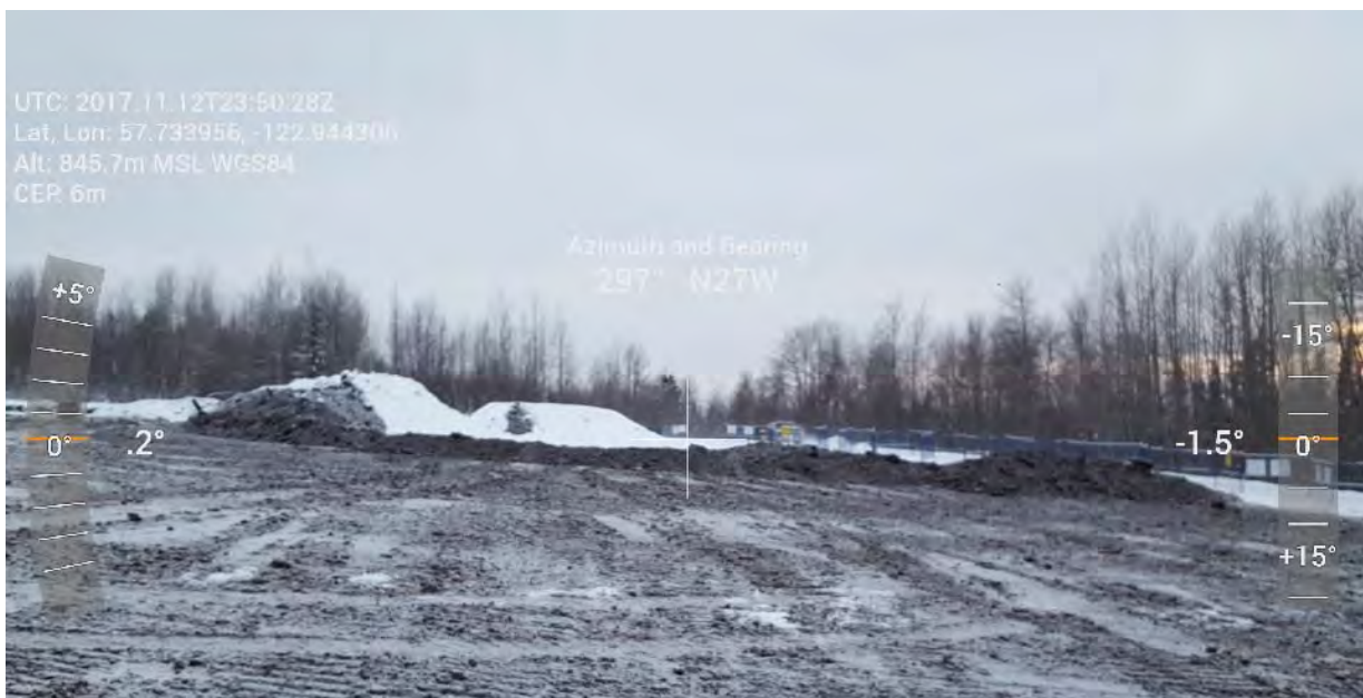
Photo 42: Spreading of overburden over backfilled AEC 1B looking towards the south.
