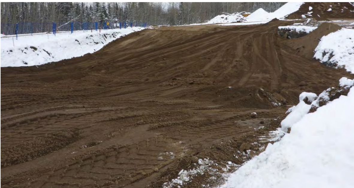
Photo 36: Continued backfilling of AEC 1B looking towards the north-east.
