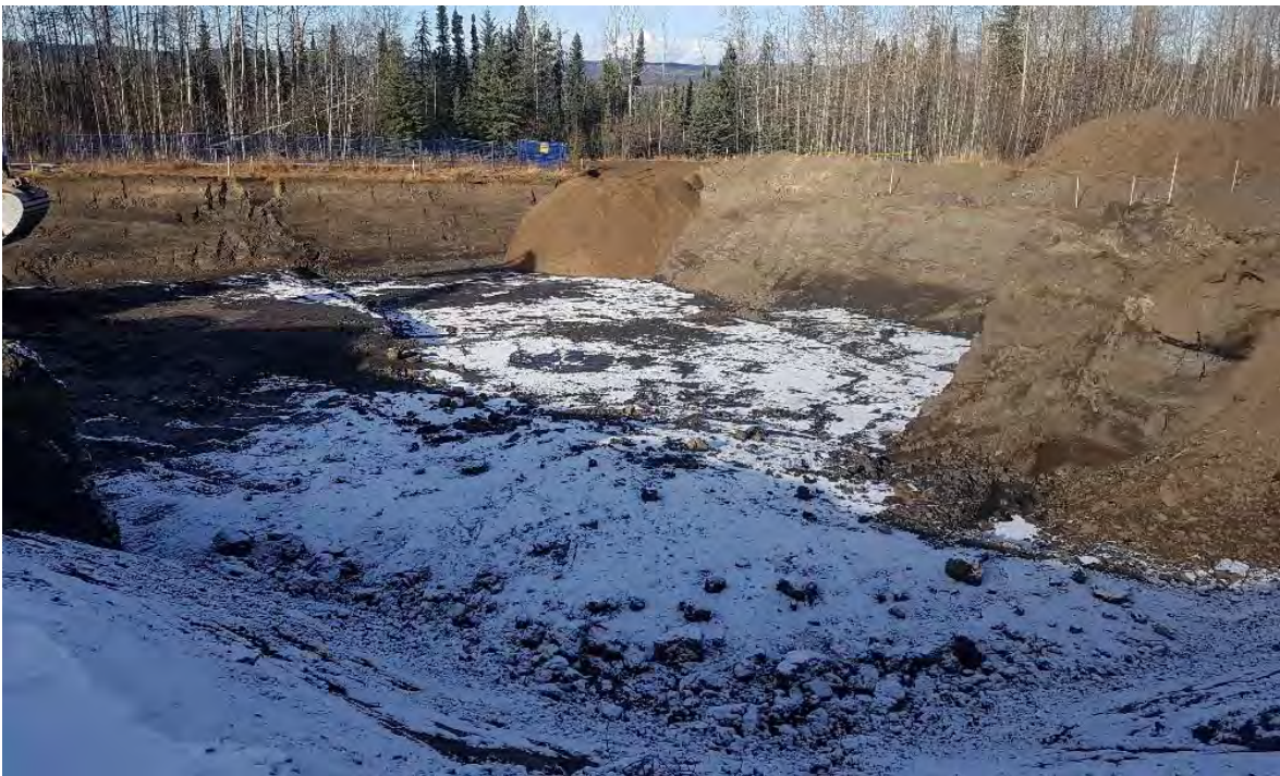
Photo 20: Backfilling north-west corner of AEC 1B looking towards the north-west.
