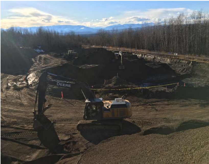
Photograph 2: AEC 1b looking southwest
