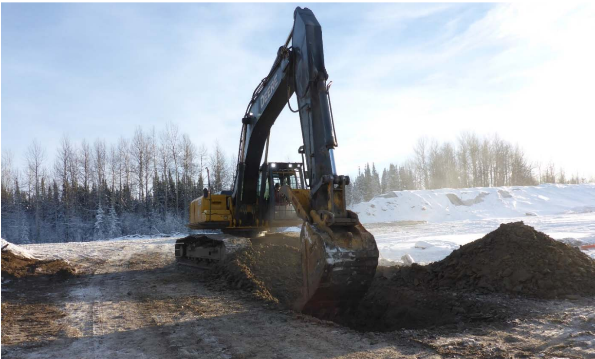
Photograph 6: Excavation of test pit K19-TP18-09 (TP-1), looking southeast. 14 January 2018.
