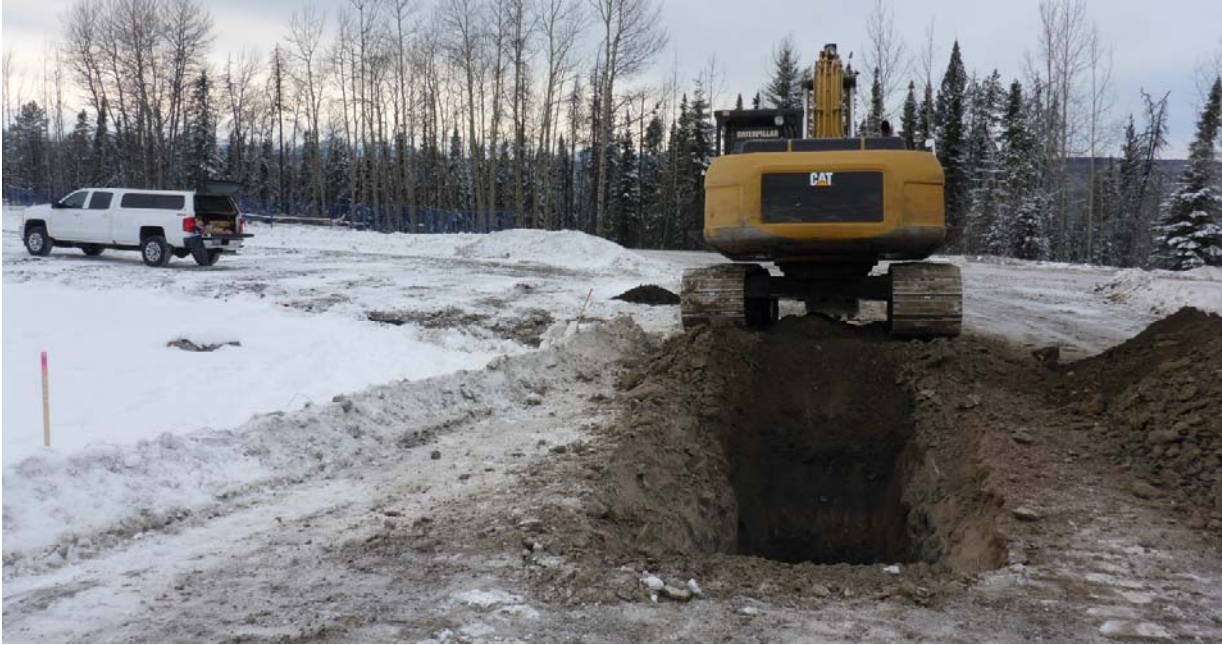
Photograph 5: Excavation of test pit K19-TP18-05 (TP-2), looking northwest. 13 January 2018.
