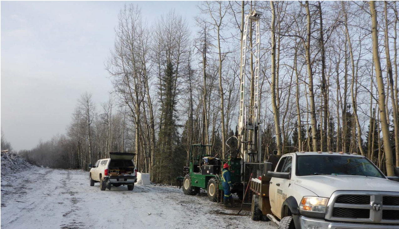
Photograph 15: Drilling groundwater monitoring well K19-MW18-09, looking southwest. 20 January 2018.
