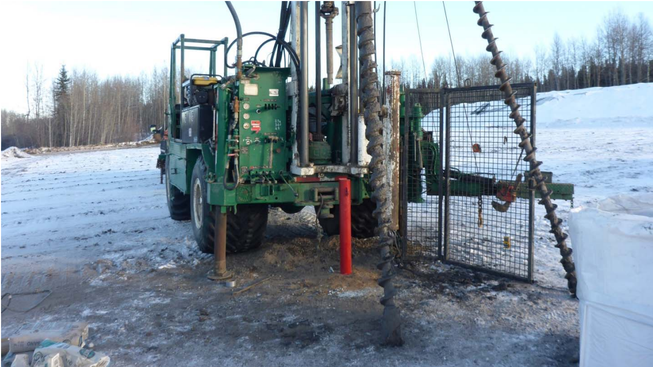
Photograph 13: Installed monitoring well K19-MW18-02, looking northeast. 17 January 2018.
