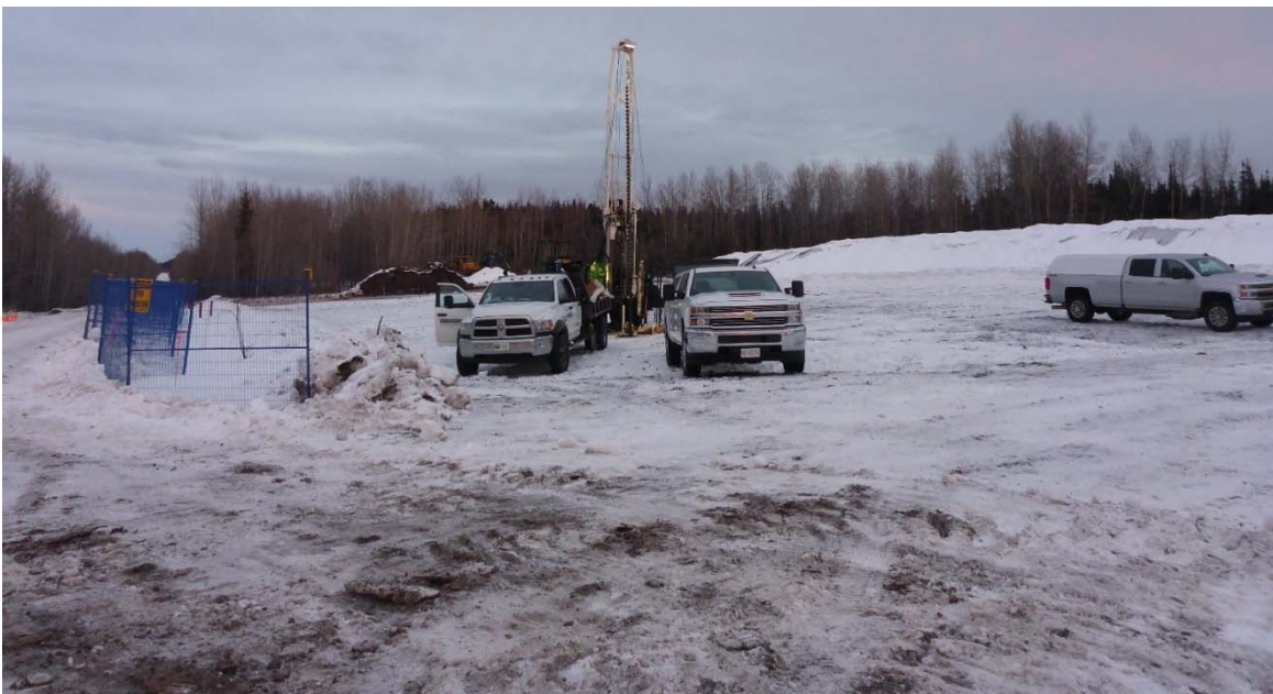
Photograph 12: Drilling of K19-MW18-01 (MW/SVP-11), looking east. 16 January 2018.
