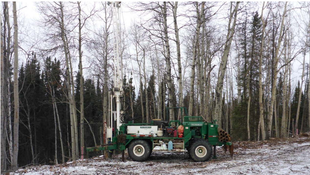
Photograph 14: Drilling groundwater monitoring well K19-MW18-07, looking north. 18 January 2018.
